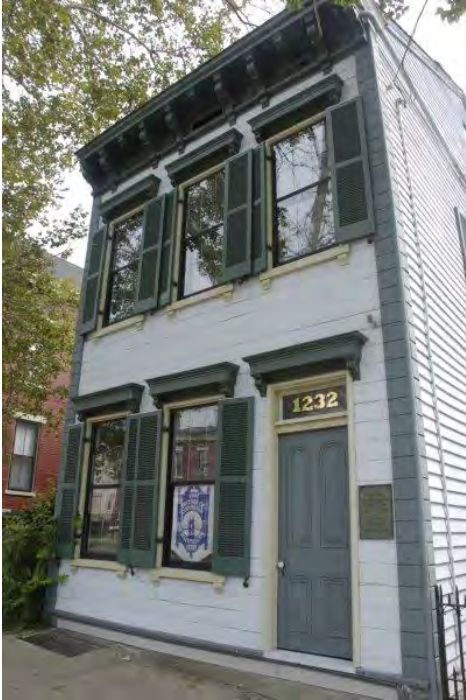
Photo 13, Front (west) façade
