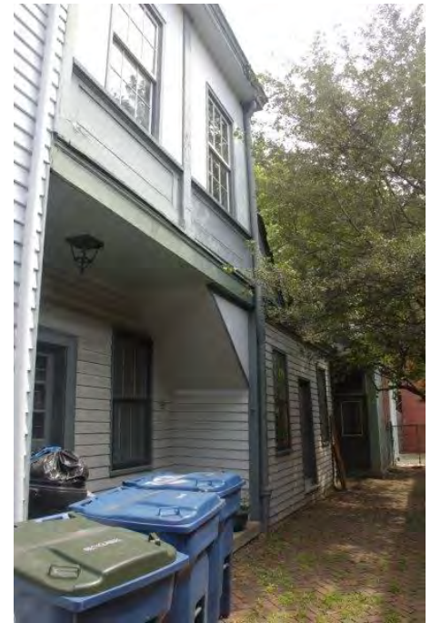
Photo 2: South façade's recessed area
