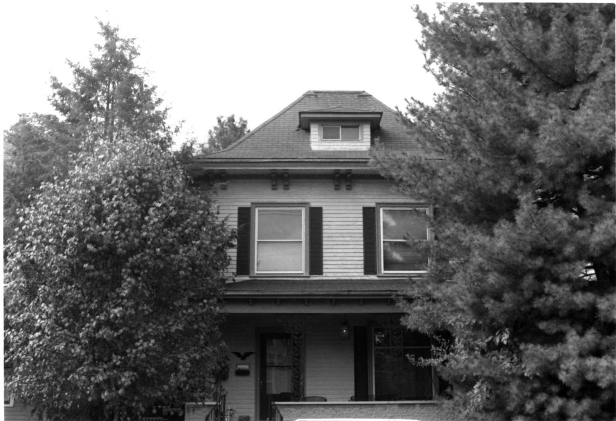
323 E. 9 TH ST., E. SPRING ST. HISTORIC DISTRICT, FLOYD CO., IN, PHOTO No. 15
