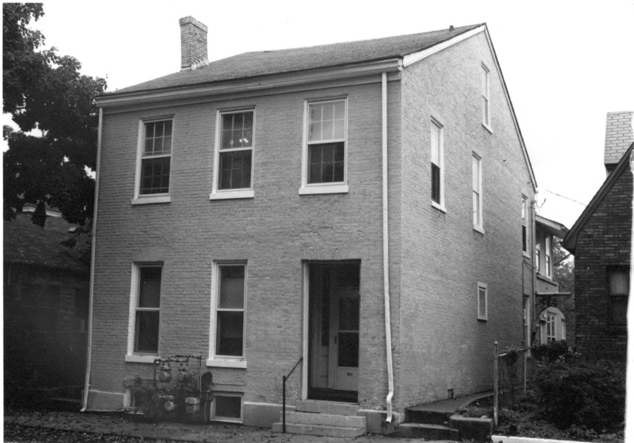
911 E. MARKET ST., E. SPRING ST. HISTORIC DISTRICT, FLOYD CO., IN, PHOTO No. 37
