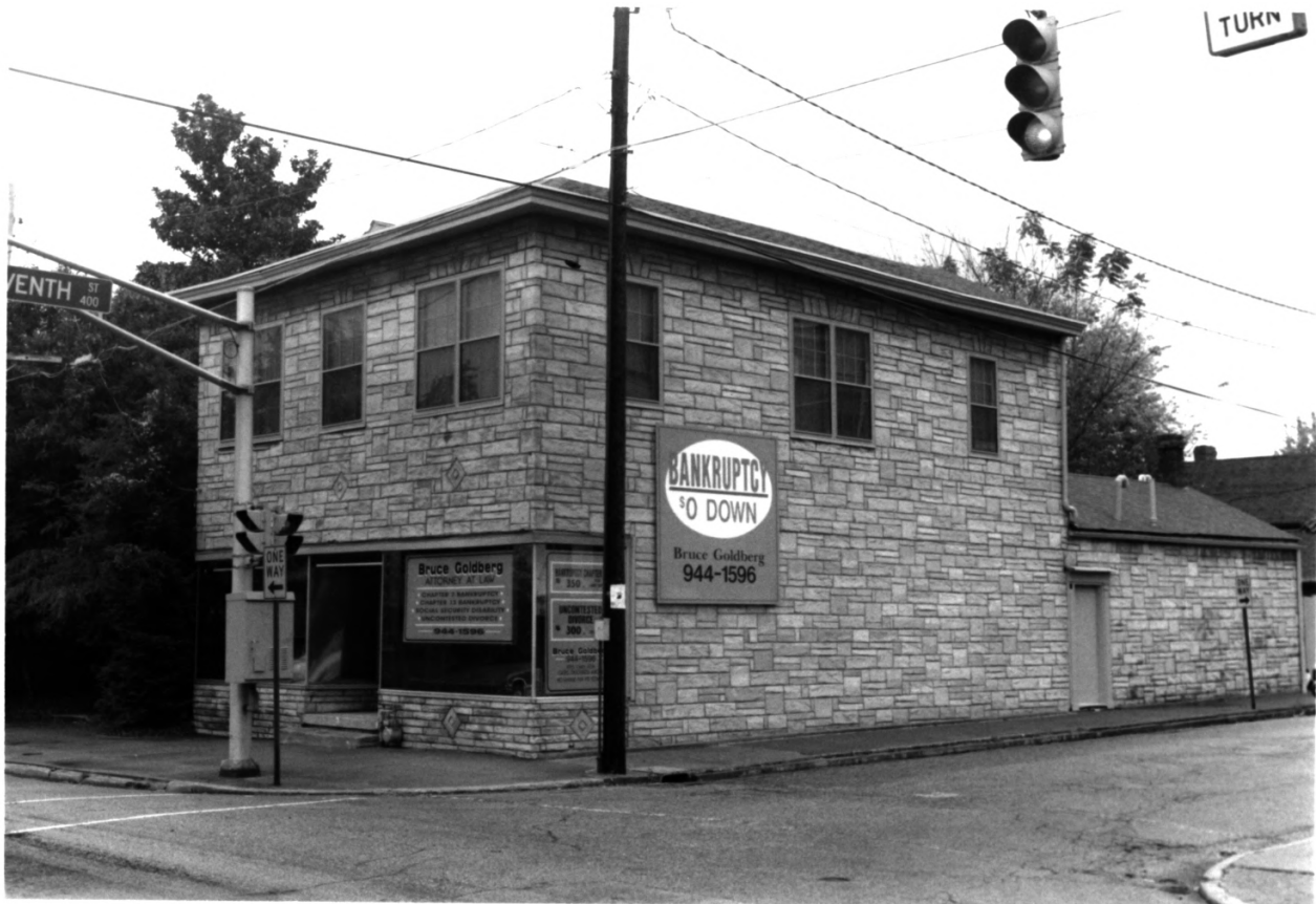
623 E. SPRING ST., E. SPRING ST. HISTORIC DISTRICT, FLOYD CO IN, PHOTO No. 6
