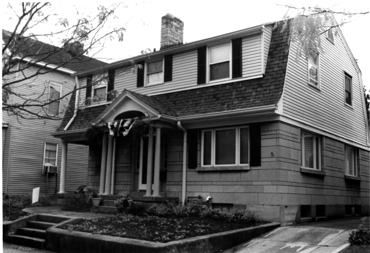
908 E. SPRING ST., E. SPRING ST. HISTORIC DISTRICT, FLOYD CO, IN, PHOTO No. 20
