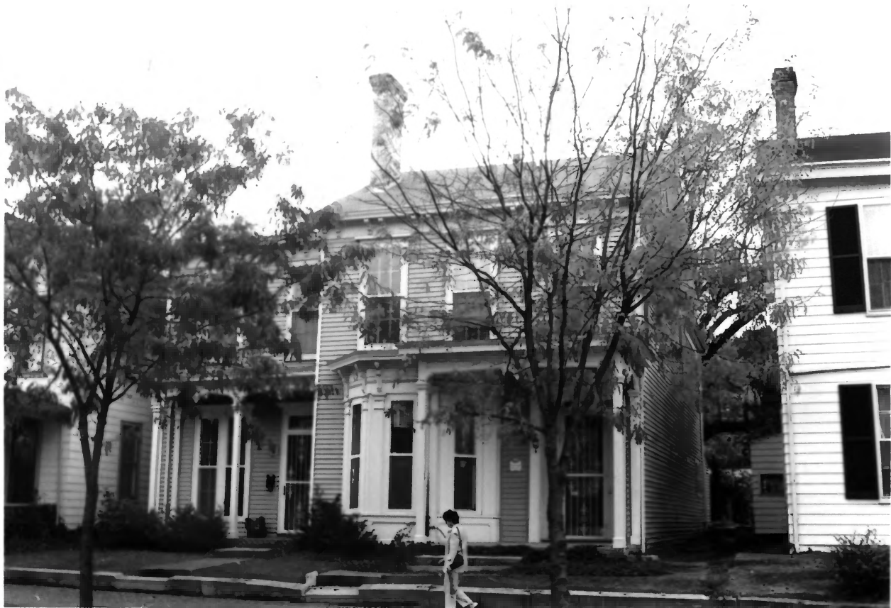
1010 E. SPRING ST., E. SPRING ST. HISTORIC DISTRICT, FLOYD CO. IN, PHOTO No. 27
