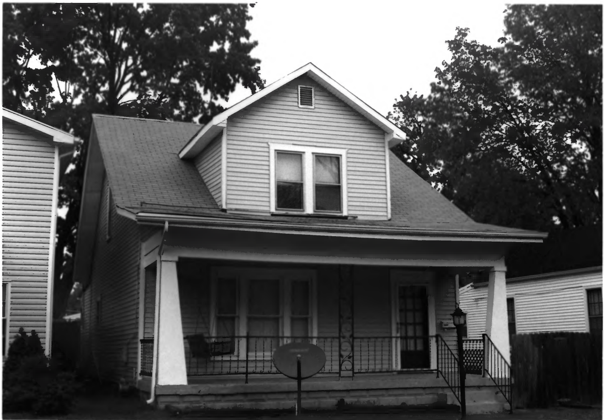
1013 E. MARKET ST., E. SPRING ST. HISTORIC DISTRICT, FLOYD CO.: IN. PHOTO NO. 3.
