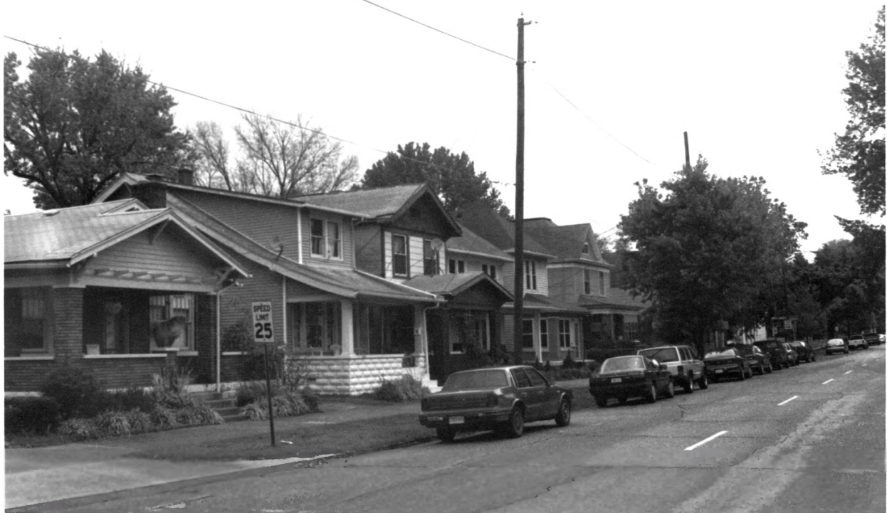
505-517 E. MARKET ST., E. SPRING ST. HISTORIC DISTRICT, FLOYD CO., IN, PHOTO NO. 50
