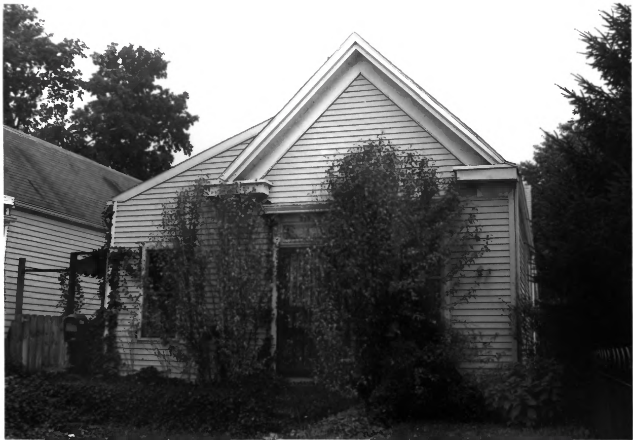
315 E. 11 TH ST., E. SPRING ST. HISTORIC DISTRICT, FLOYD CO., IN, PHOTO No. 29
