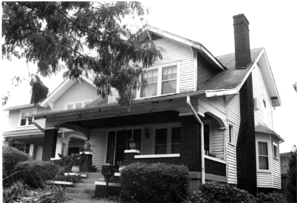
920 E. SPRING ST., E. SPRING ST. HISTORIC DISTRICT, FLOYD CO. IN, PHOTO NO. 21
