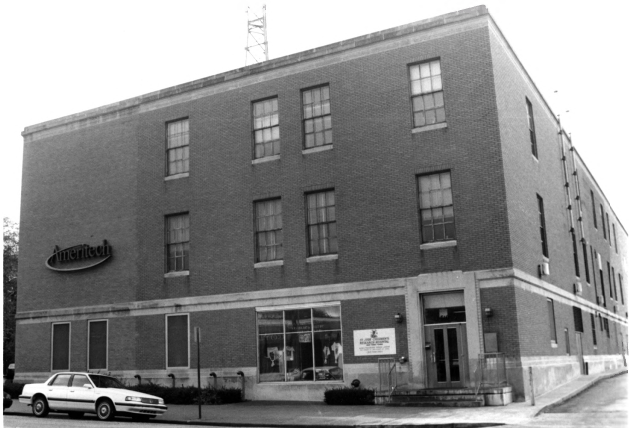
510 E. SPRING, E. SPRING ST. HISTORICAL DISTRICT, FLOYD CO., IN, PHOTO No. 1
