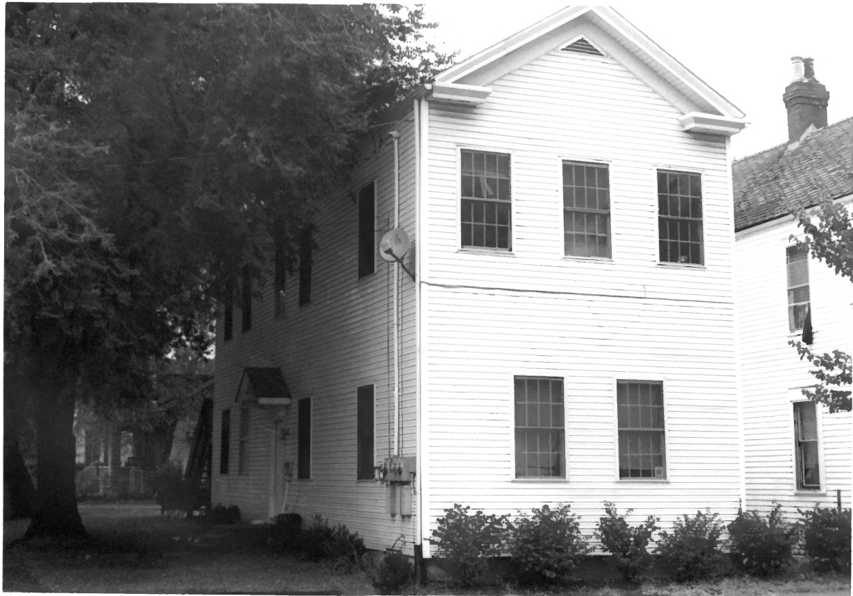
1001 E. MARKET ST., E. SPRING ST. HISTORIC DISTRICT, FLOYDCO., IN, PHOTO No. 53
