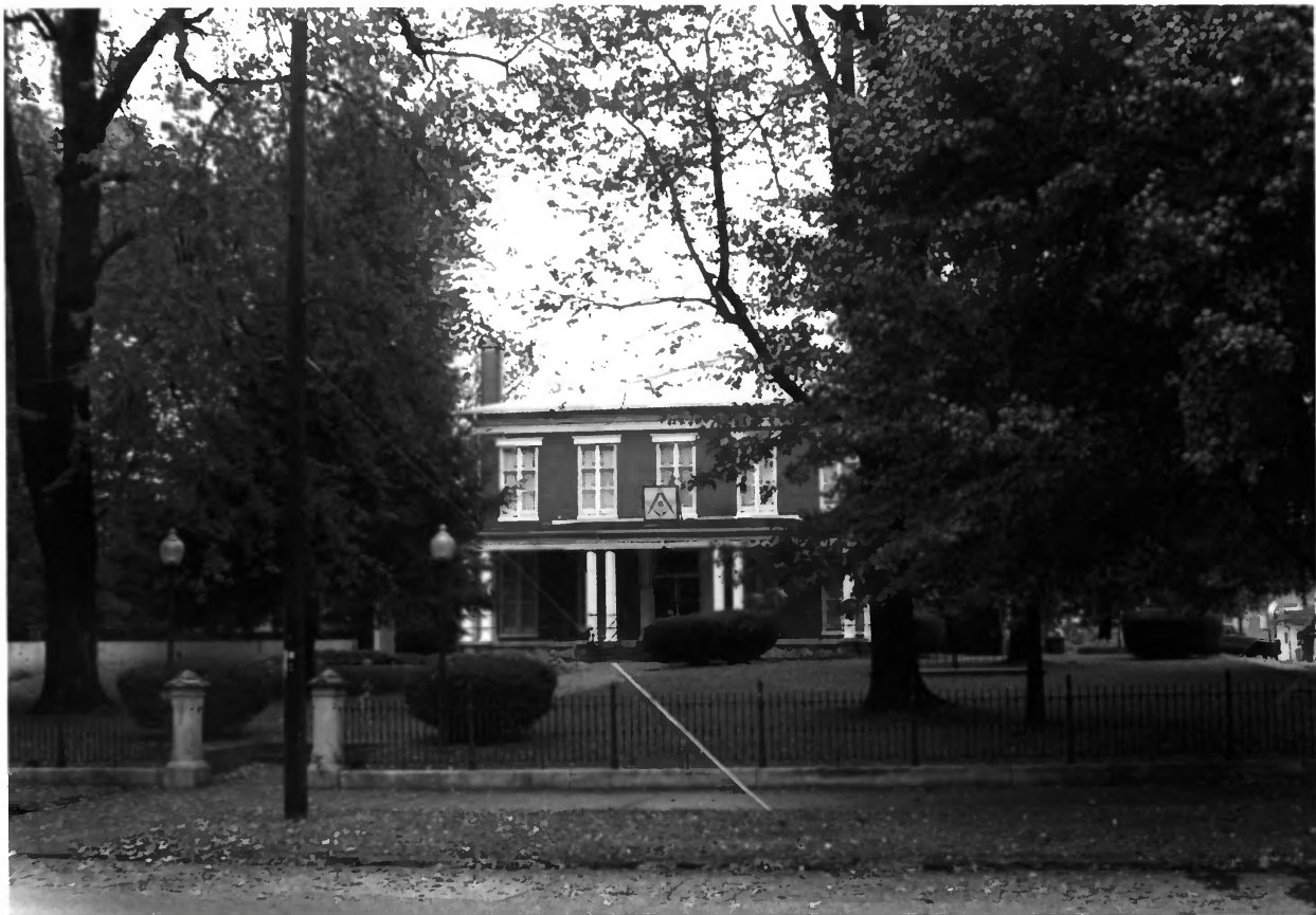
805 E. MARKET ST., E. SPRING ST. HISTORIC DISTRICT, FLOYD CO., IN., PHOTO No 41
