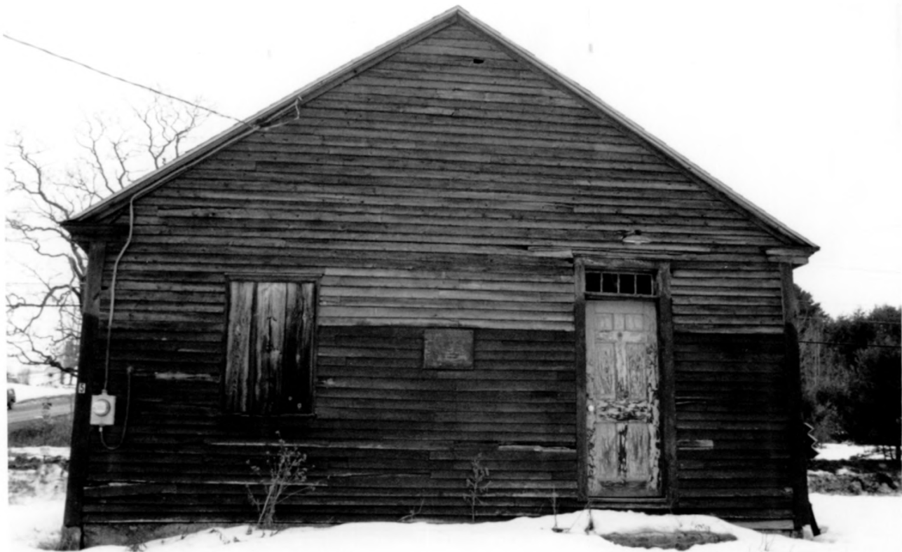
DUDLEY'S CORNER SCHOOLHOUSE; SOMERSET CO., MAINE
