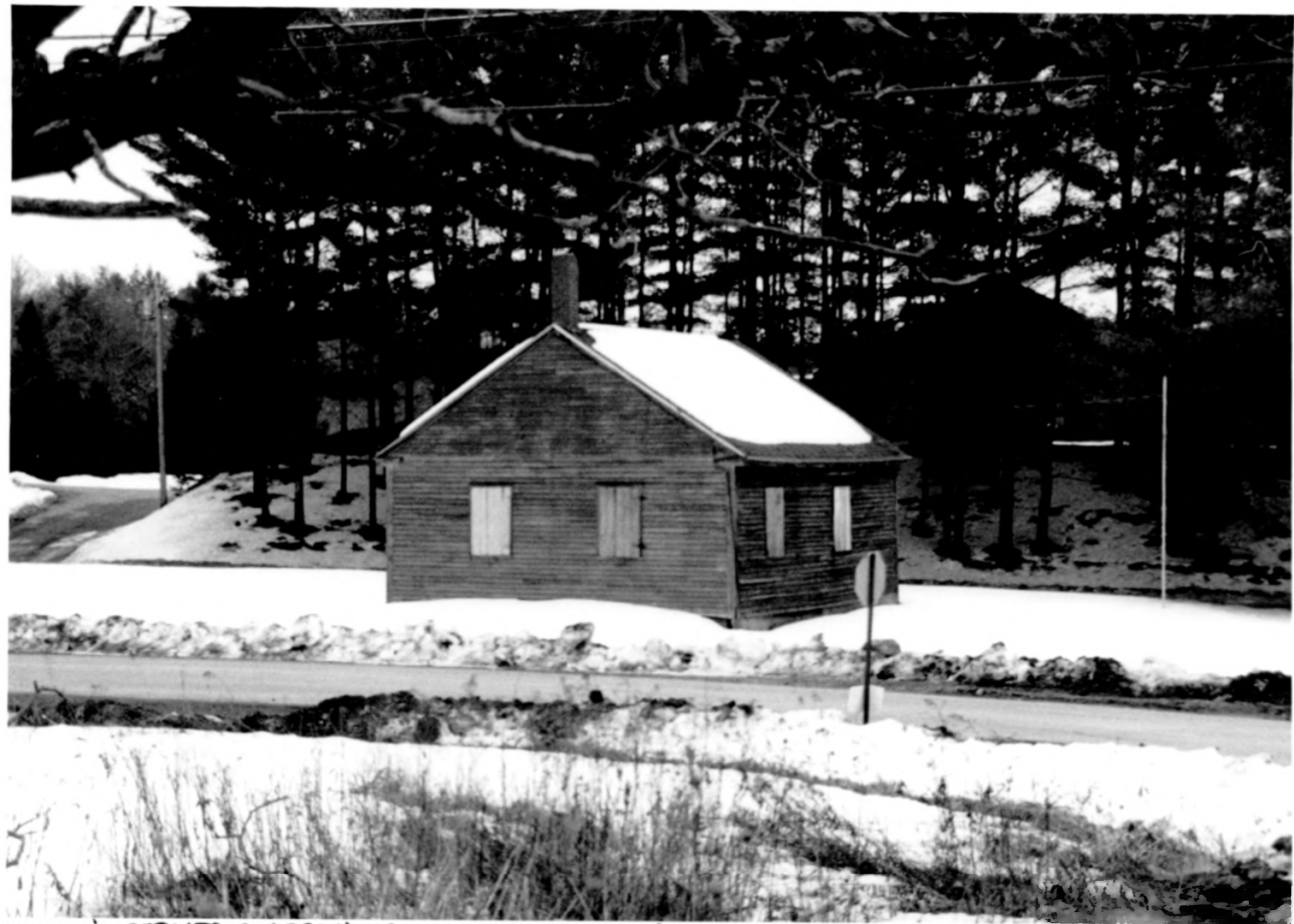
DUDLEY'S CORNER SCHOOLHOUSE ; SOMERSET CO., MAINE
