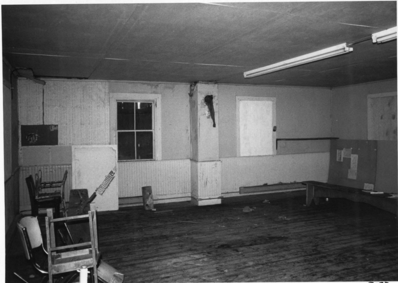
DUDLEY'S CORNER SCHOOLHOUSE; SOMERSET CO., MAINE
