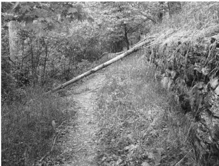
Photo#0017 Retaining wall near Fairy Steps. View to the east.
