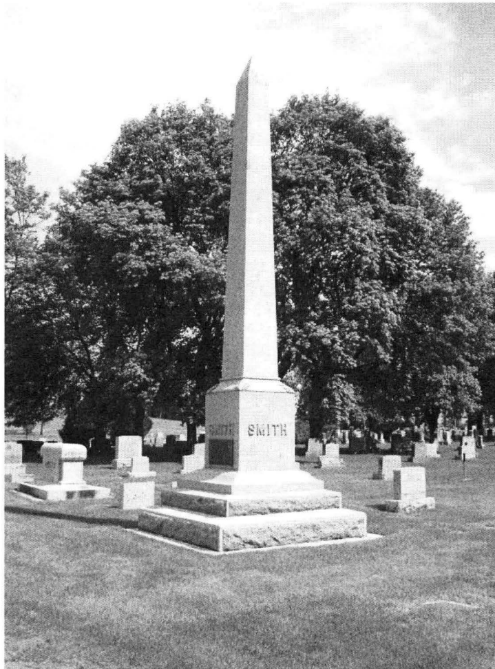
Photo# 0019 North and east elevations, Governor Smith obelisk, Section H. View to the southwest.
