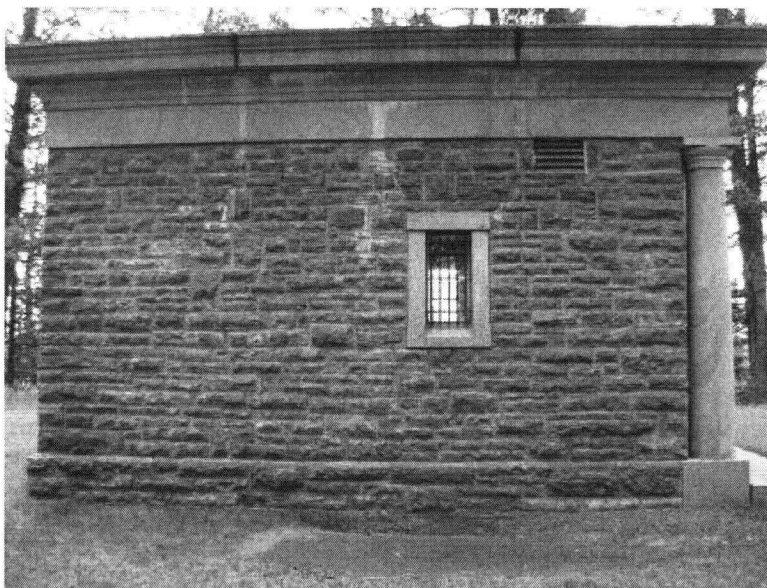
Photo# 0009 Conrad Mausoleum, west elevation. , View to the east.
