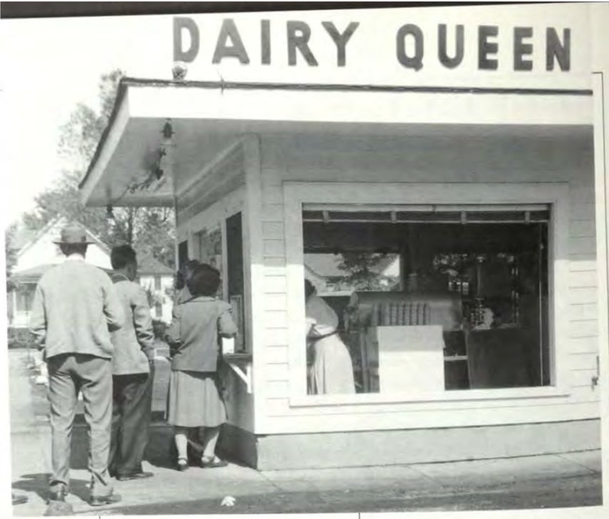
Figure 8: The McCulloughs' Dairy Queen store in Moline, Illinois, 1941, which influenced the prototypical post-war design ( The Cone with the Curl on Top: The "Dairy Queen" Story )
