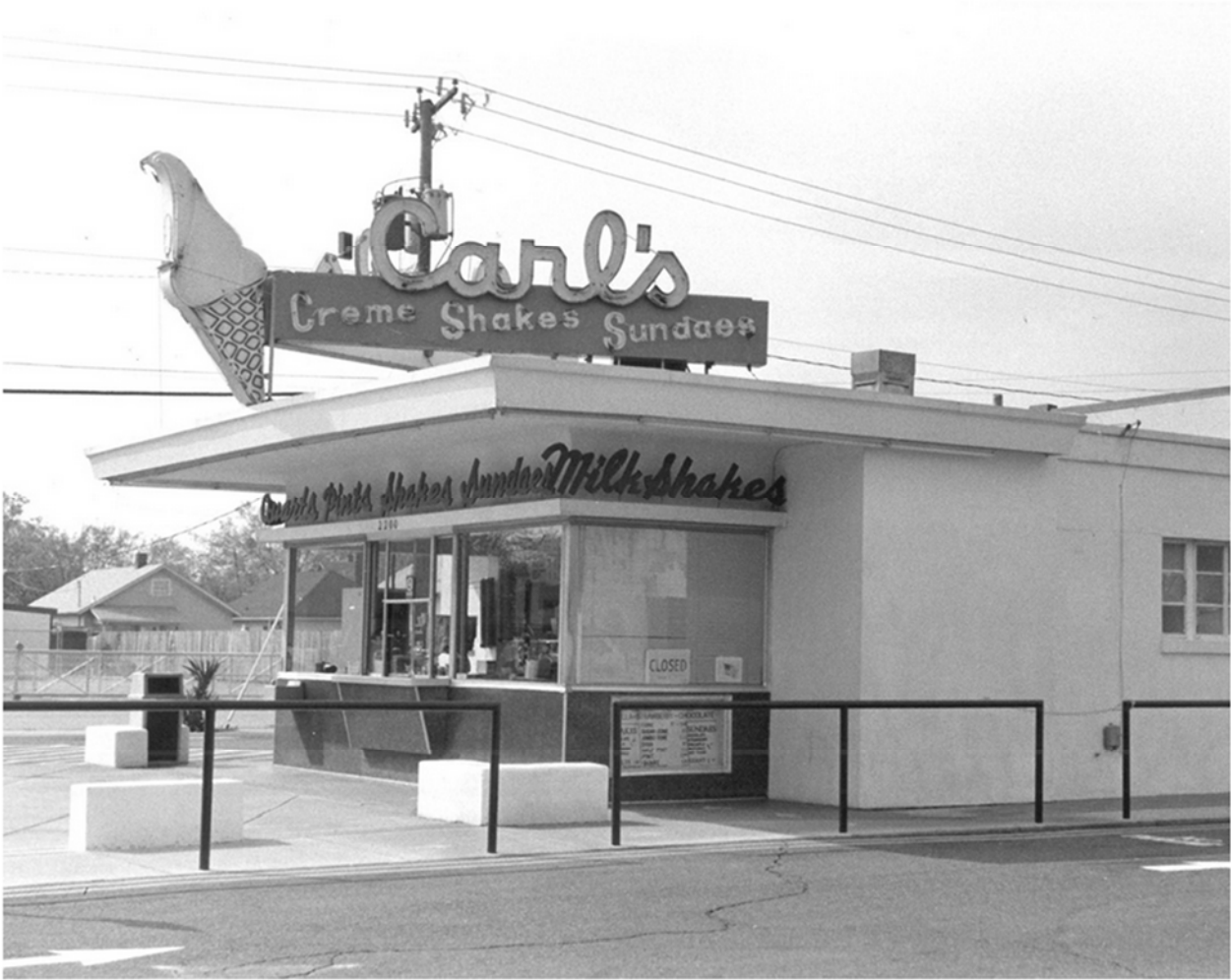
Figure 27: Independent Carl's Frozen Custard in Fredericksburg, VA, built 1953, with similar design features to Dairy Queen (Virginia Department of Historic Resources)
