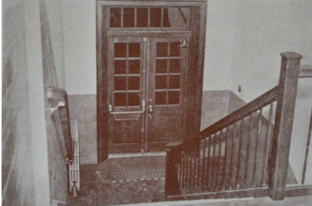
Rollinsford Grade School in 1937 showing the original exterior doors. Image from the American School Board Journal, November/December 1937.
