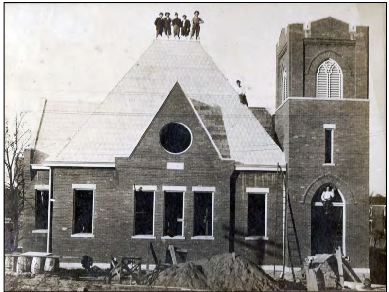
Figure 1: Presbyterian Church, U.S.A., under Construction in 1910. Source of Photo Unknown
