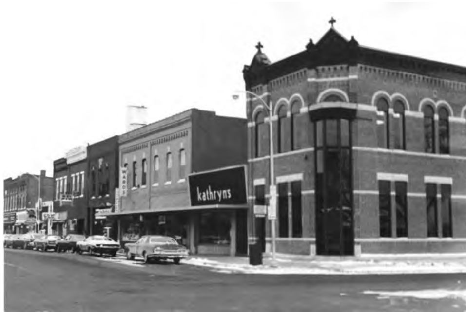
Figure T View of West Main Street, facing north, 1980, photographer Camille Kudzia. National Register of Historic Places, Wabasha Commercial Historic District, Wabasha County, Minnesota, National Register Nomination #82003063.
