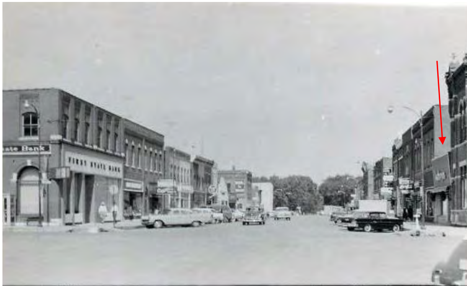
Figure P View of West Main Street, facing northwest, 1950s. John Schmidt Building identified by red arrow. Courtesy of Lakesnwoods.com.
