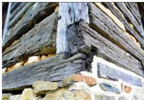
Complex joinery was needed to keep the building tight and sturdy. The drawing illustrates the corner post bottom to sill joinery used in the shop.
