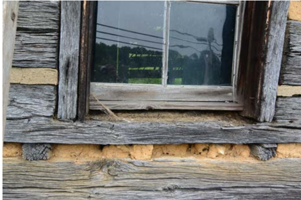
Evidence suggests that many log interstices never had chinking (left). Only the south wall was fully chinked (right), and the chinking was only for the exterior daubing. A few of the long chinking pieces were pegged in place.
