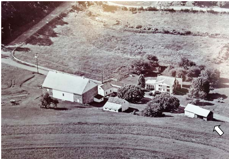
This 1974 aerial view shows the rear elevation of the shop (indicated by arrow), barn, and other outbuildings.
