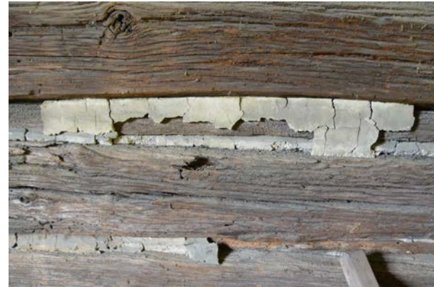
The mud daubing, a mixture of clay, stream bed sediment/sand, and a very little chunk lime was used to fill the bulk of the cracks. (left) Without lime coat protection, the mud daubing weathered very quickly. Very small amounts of original lime daubing were located on both the gable end walls. The south gable daubing, shown here (right), was applied during two different periods. The narrow V joint profile is original. It was later covered by the more liberally-applied lime coat during a second campaign of daubing.
