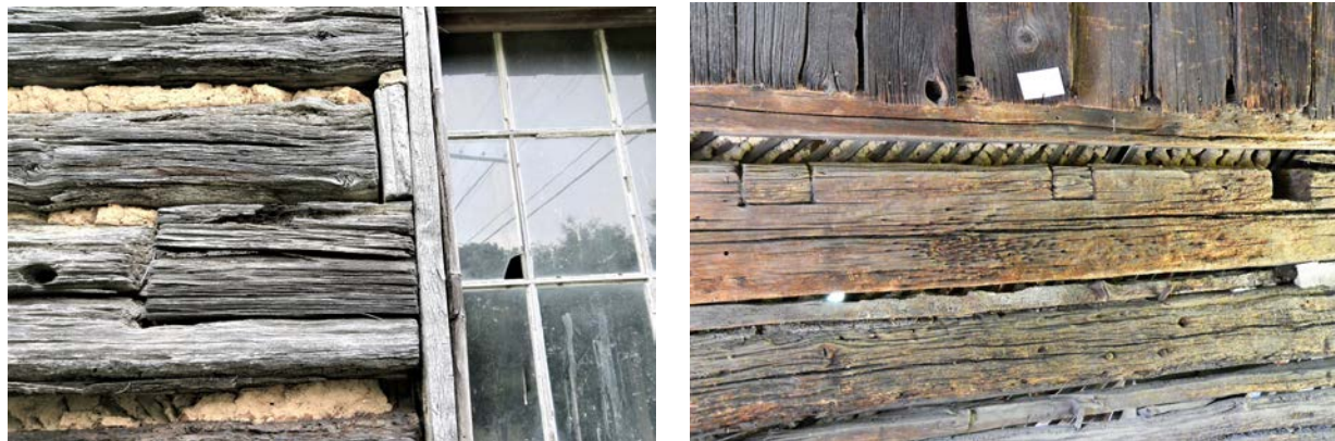
In the left photo, two blocks are visible left of the window. The smaller, upper block extended a log's width. The larger block below it filled in a window or door opening cut for the earlier building. In the right photo, this log, just under a top plate, had four joists remaining from the prior building.
