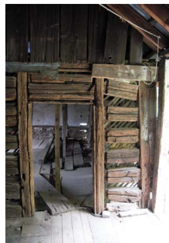
Second floor view of the interior, showing the north-facing gable-end wall (left) and the former exterior Dutch door of the south-facing end wall, now covered by the interior of the garage addition (right). These Type 1 door posts are typical of every building with door openings in log walls.
