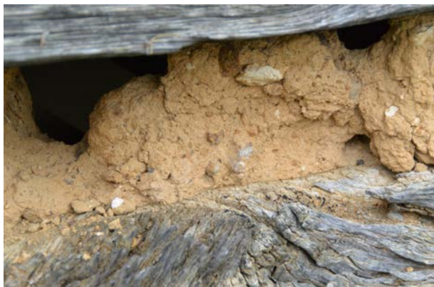
The mud daubing, a mixture of clay, stream bed sediment/sand, and a very little chunk lime was used to fill the bulk of the cracks. (left) Without lime coat protection, the mud daubing weathered very quickly. Very small amounts of original lime daubing were located on both the gable end walls. The south gable daubing, shown here (right), was applied during two different periods. The narrow V joint profile is original. It was later covered by the more liberally-applied lime coat during a second campaign of daubing.
