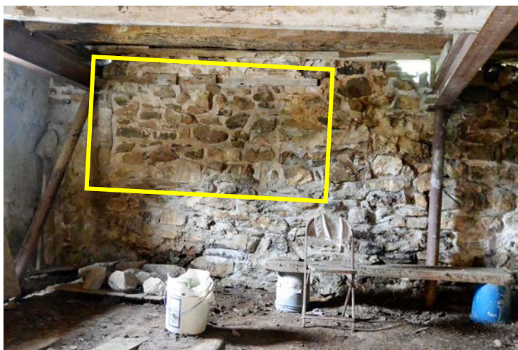
The outline (left photo) surrounds an area believed to be a former window. The vertically-oriented jamb stones flanking an existing window (right) were typical in well-laid stone masonry. This wall, facing the road, has been repointed.
