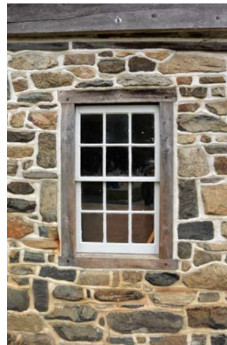
The outline (left photo) surrounds an area believed to be a former window. The vertically-oriented jamb stones flanking an existing window (right) were typical in well-laid stone masonry. This wall, facing the road, has been repointed.
