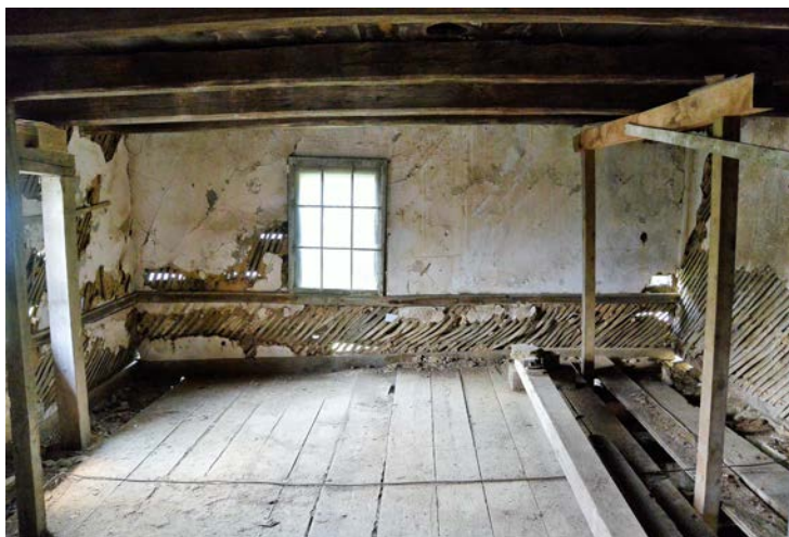
Second floor view of the interior, showing the north-facing gable-end wall (left) and the former exterior Dutch door of the south-facing end wall, now covered by the interior of the garage addition (right). These Type 1 door posts are typical of every building with door openings in log walls.
