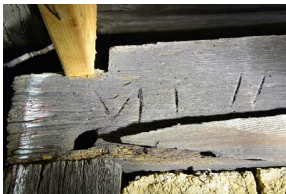
Roman numerals and markings carved into the logs indicated how they would fit together. Slashes indicated a particular wall, and numbers denoted the order of the individual logs within that wall. Here the numbers rise from the bottom log up, from 1 to VII.
