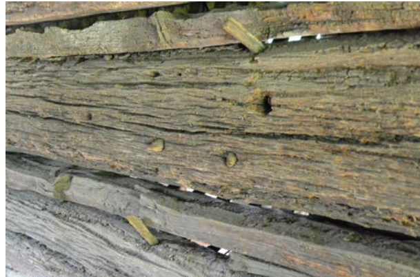
Evidence suggests that many log interstices never had chinking (left). Only the south wall was fully chinked (right), and the chinking was only for the exterior daubing. A few of the long chinking pieces were pegged in place.
