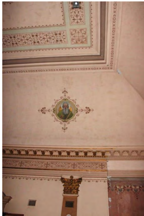
FIGURE 27. CHURCH: NAVE CEILING, DETAIL OF ORNAMENT ON COFFERED SECTION, 2016.
