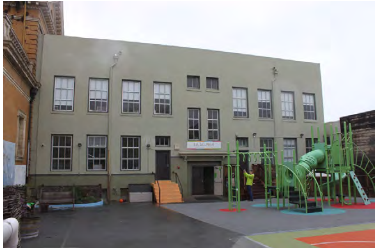
FIGURE 44. SCHOOL: REAR (SOUTH) ELEVATION AND SCHOOL YARD, 2016.
