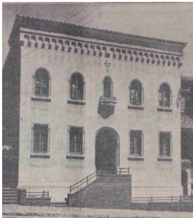
FIGURE 60. SACRED HEART CONVENT JUST AFTER COMPLETION IN 1936. SOURCE: CATHOLIC MONITOR, AUGUST 15, 1936
