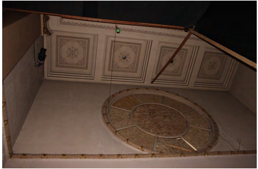
FIGURE 29: CHURCH: NORTH TRANSEPT SHOWING DECORATIVE DETAILING, 2016.
