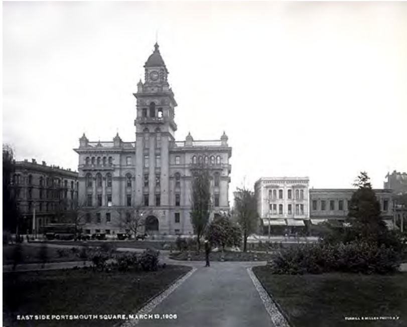
FIGURE 78. WELSH'S SAN FRANCISCO SUPREME COURT (HALL OF JUSTICE) AS BUILT, 1906. SOURCE: SAN FRANCISCO SHERIFF'S DEPARTMENT
