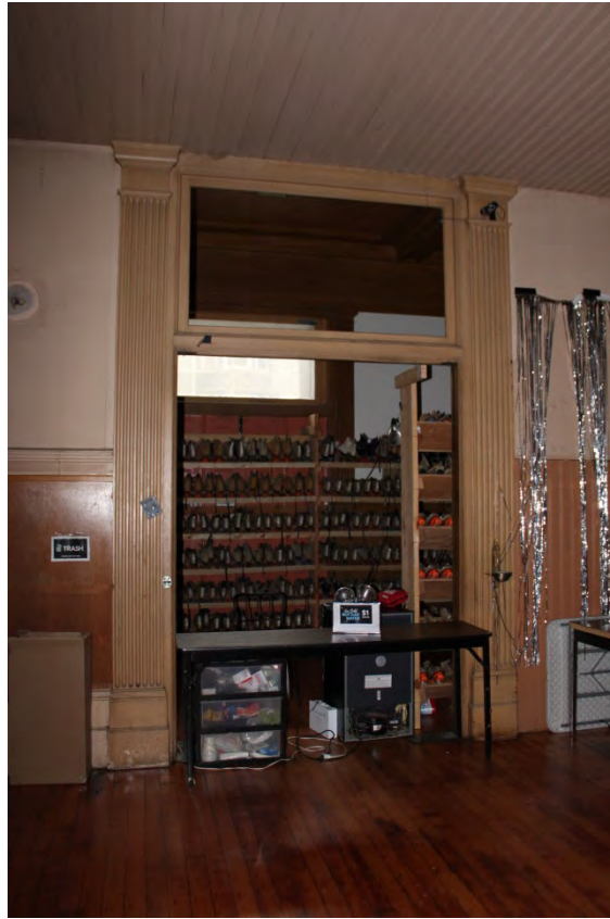
FIGURE 25. CHURCH: NAVE, NORTH DOOR FROM NARTHEX, 2016.
