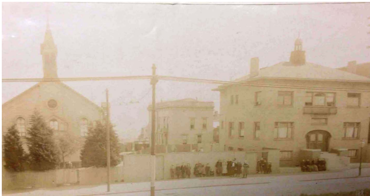
FIGURE 51. SACRED HEART PARISH COMPLEX IN THE MID-1890S SHOWING ORIGINAL CONFIGURATION OF RECTORY (RIGHT), THE FIRST CONVENT (CENTER RIGHT), AND THOMAS WELSH'S 1888 WOOD-FRAME SACRED HEART CHURCH (LEFT). SOURCE: ARCHIVES OF THE ARCHDIOCESE OF SAN FRANCISCO
