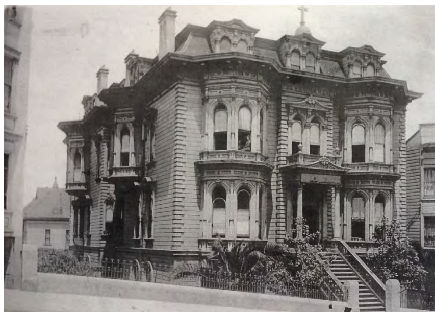
FIGURE 58. OLD SUTRO MANSION/SACRED HEART SCHOOL AND CONVENT, HAYES AND FILLMORE STREETS, SAN FRANCISCO, CA. 1910. (DEMOLISHED 1914) SOURCE: ARCHIVES OF THE DOMINICAN SISTERS OF SAN RAFAEL, SAN RAFAEL, CA
