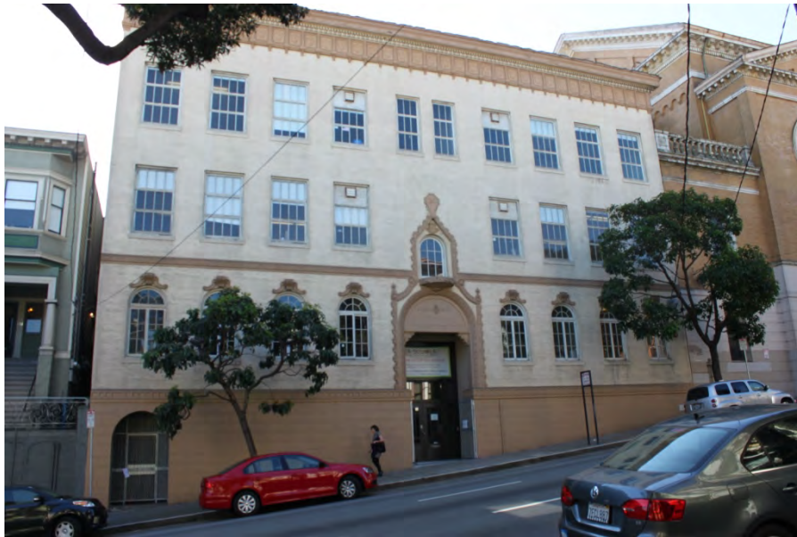
FIGURE 42. SCHOOL: MAIN (NORTH) ELEVATION, LOOKING SOUTH FROM FELL STREET, 2015.
