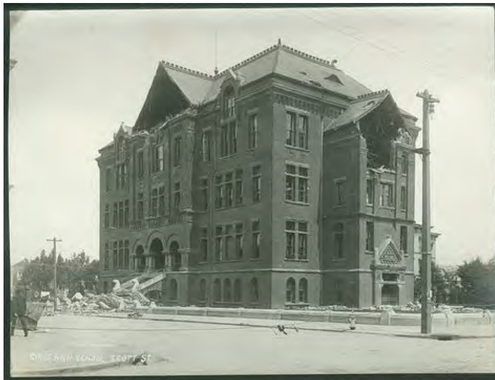
FIGURE 80. WELSH'S GIRLS HIGH SCHOOL AFTER DAMAGE IN THE 1906 EARTHQUAKE. SOURCE: DELGOYER LIBRARY, SOUTHERN METHODIST UNIVERSITY
