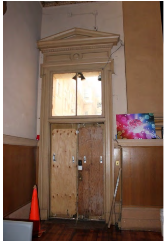
FIGURE 30: CHURCH: NAVE, SOUTH TRANSEPT ENTRY TO ALLEY, 2016.
