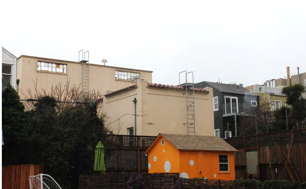
FIGURE 49. CONVENT: REAR (NORTH) ELEVATIONS OF CHAPEL ELL AND MAIN BLOCK, 2016.
