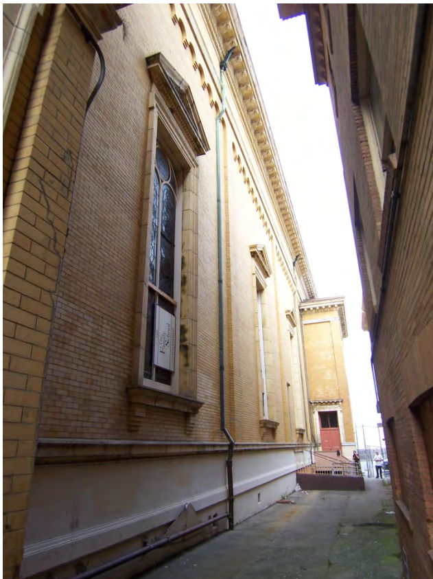
FIGURE 9. CHURCH: SOUTH ELEVATION LOOKING EAST. (PHOTO 2009. COURTESY CHRIS VERPLANCK)
