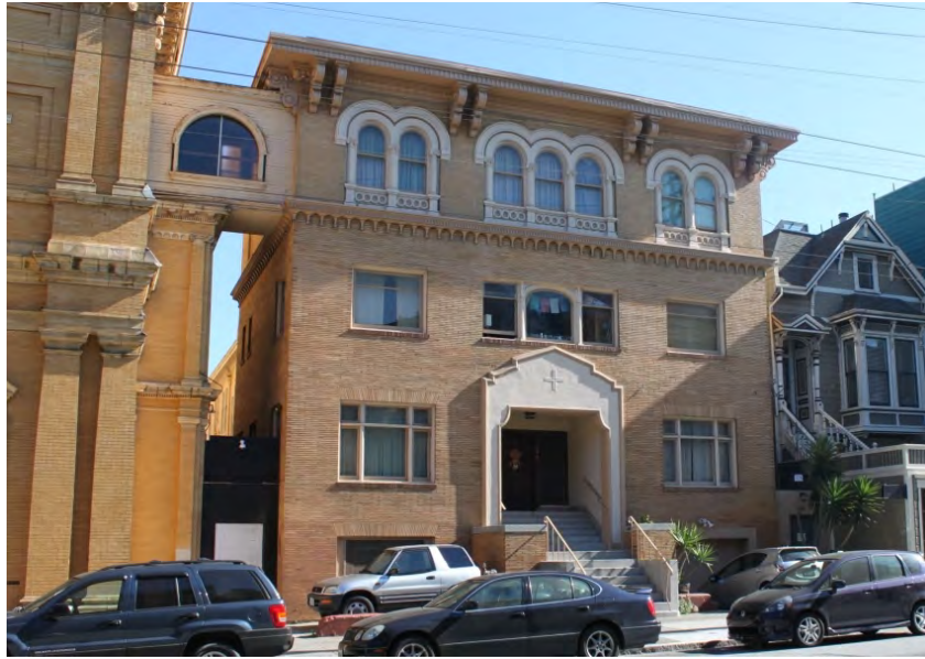
FIGURE 37. RECTORY: MAIN (WEST) ELEVATION FROM FILLMORE STREET, 2015.
