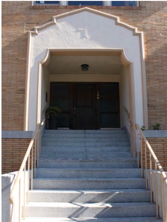
FIGURE 38 (LEFT). RECTORY: MAIN ENTRANCE, 2015.
