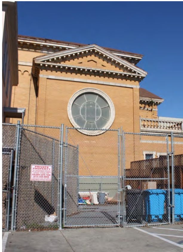
FIGURE 10: CHURCH: SOUTH TRANSEPT AND SACRISTY LOOKING NORTH FROM PARKING AREA OFF OAK ST., 2015.
