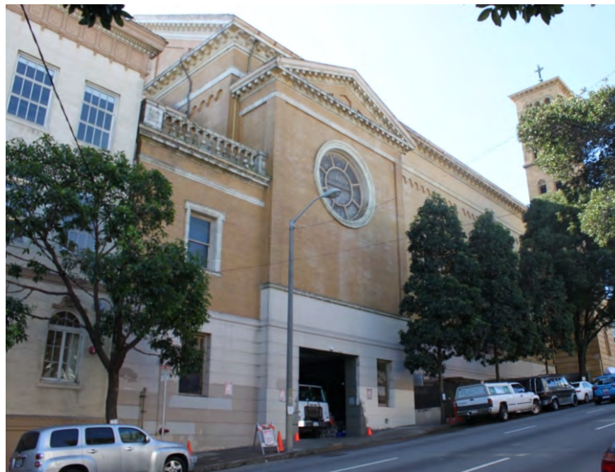
FIGURE 7. CHURCH: NORTH ELEVATION, LOOKING SOUTHWEST FROM FELL ST., 2015.
