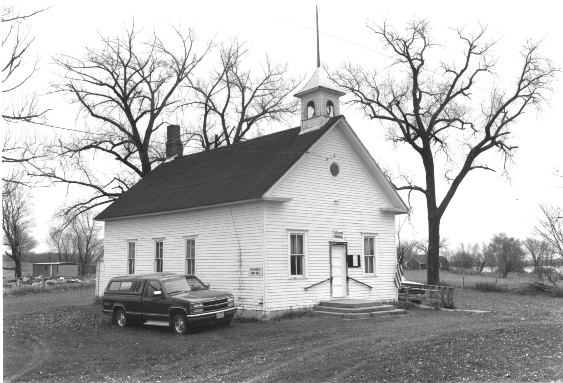
District No. 48 School Off Co. Hwy. 6, Collinwood Township Meeker Co., Mn 010045-10/10A
