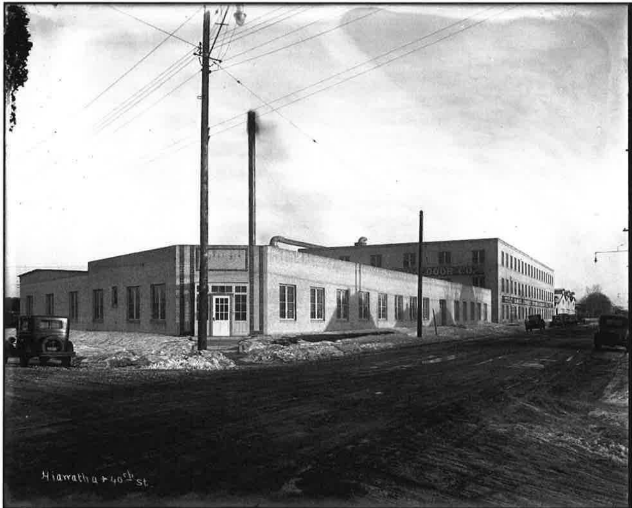
Figure 4: Lake Street Sash and Door Company, view southeast towards corner of 40 th Street and Hiawatha Avenue. (Left to right) Warehouse, Factory 2 and Lumber Shed, ca. late-1920s.
