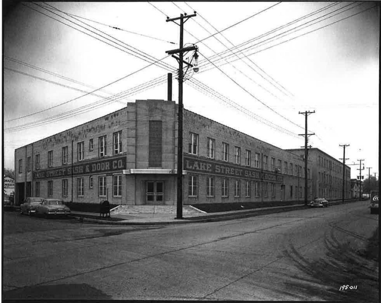
Figure 6: Lake Street Sash and Door Company, view southeast towards corner of 40 th Street and Hiawatha Avenue. (Left to right) Warehouse, Factory 2 and Lumber Shed, 1950.
