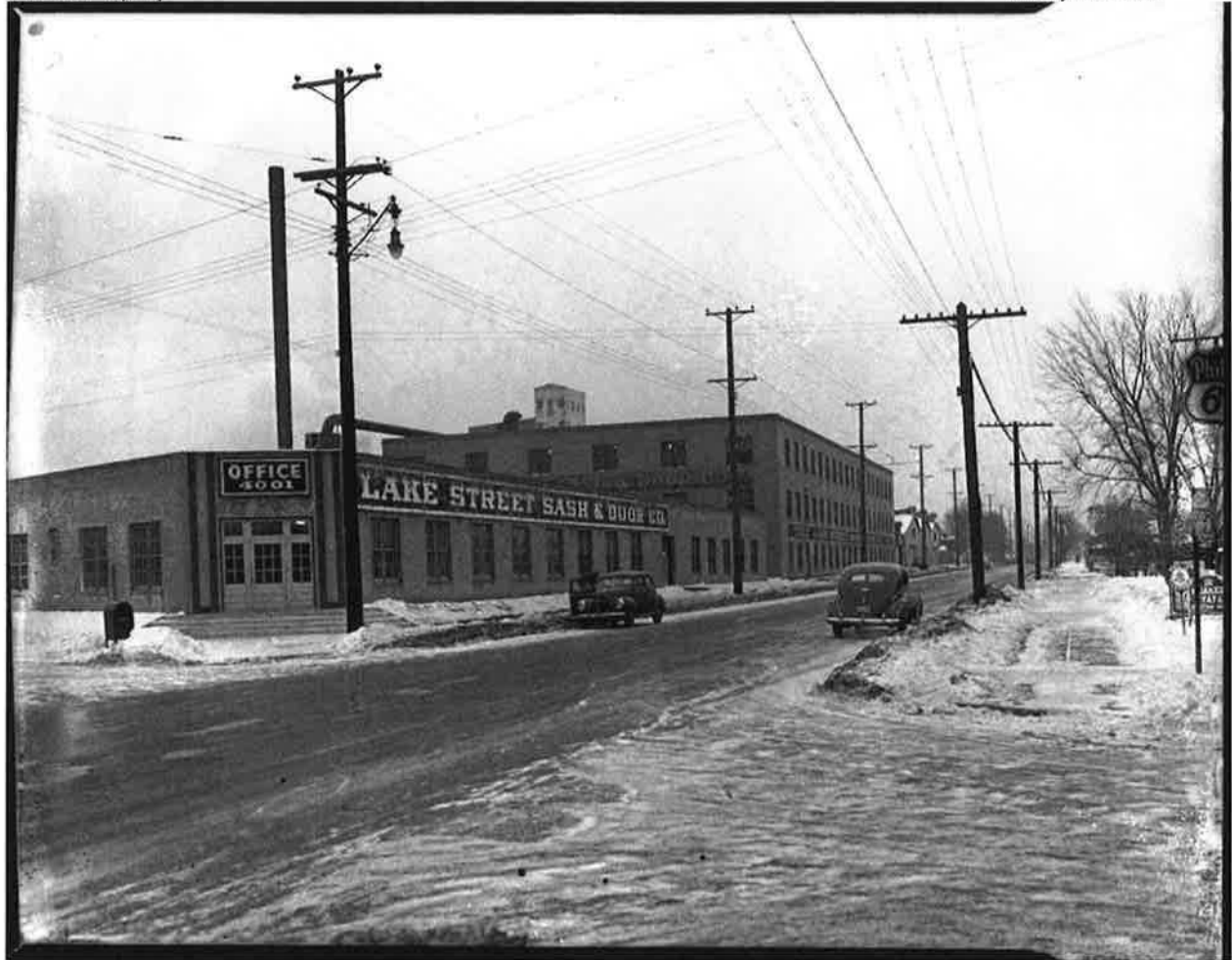
Figure 5: Lake Street Sash and Door Company, view southeast towards corner of 40 th Street and Hiawatha Avenue. (Left to right) Warehouse, Factory 2 and Lumber Shed, 1945.
