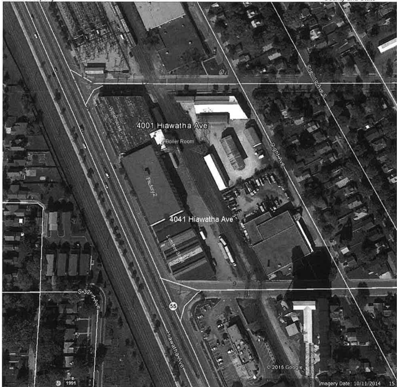
Figure 2: Contemporary aerial view of the Lake Street Sash and Door Company with exterior photographs keyed to locational view.
