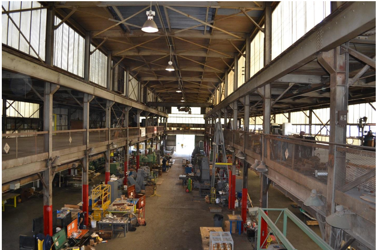
Photo 15 – Building #11, interior view north from second floor, June 2017.
