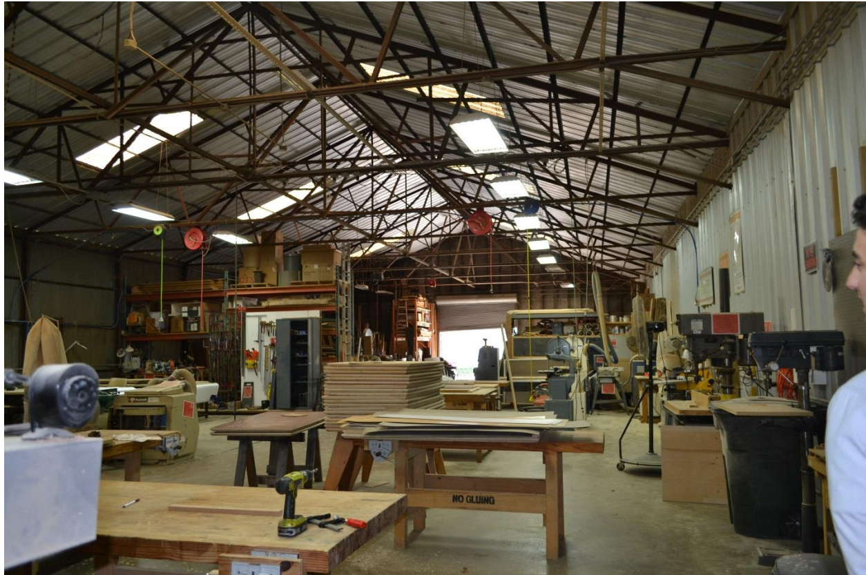
Photo 20 – Building #19, view south, October 2017. Party wall between Building #19 and Building #15 is visible on the right.
