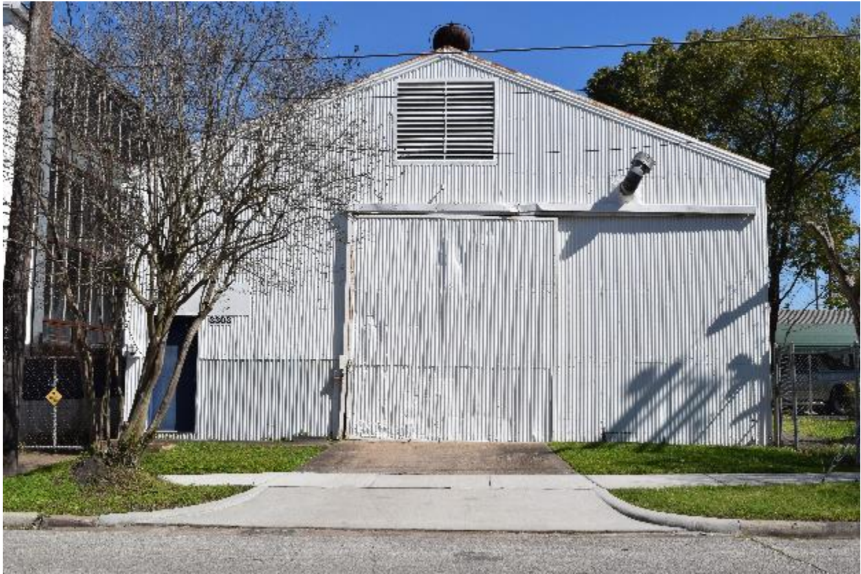
Photo 21 – South (front) elevation of Building #17, view north, February 2017.
