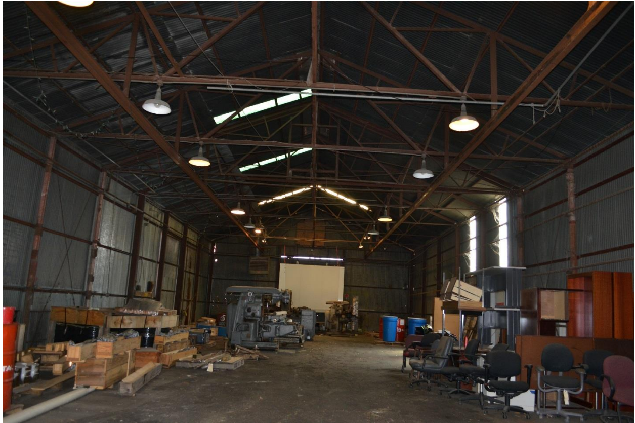
Photo 22 – Interior of Building #17, view north, June 2017.
