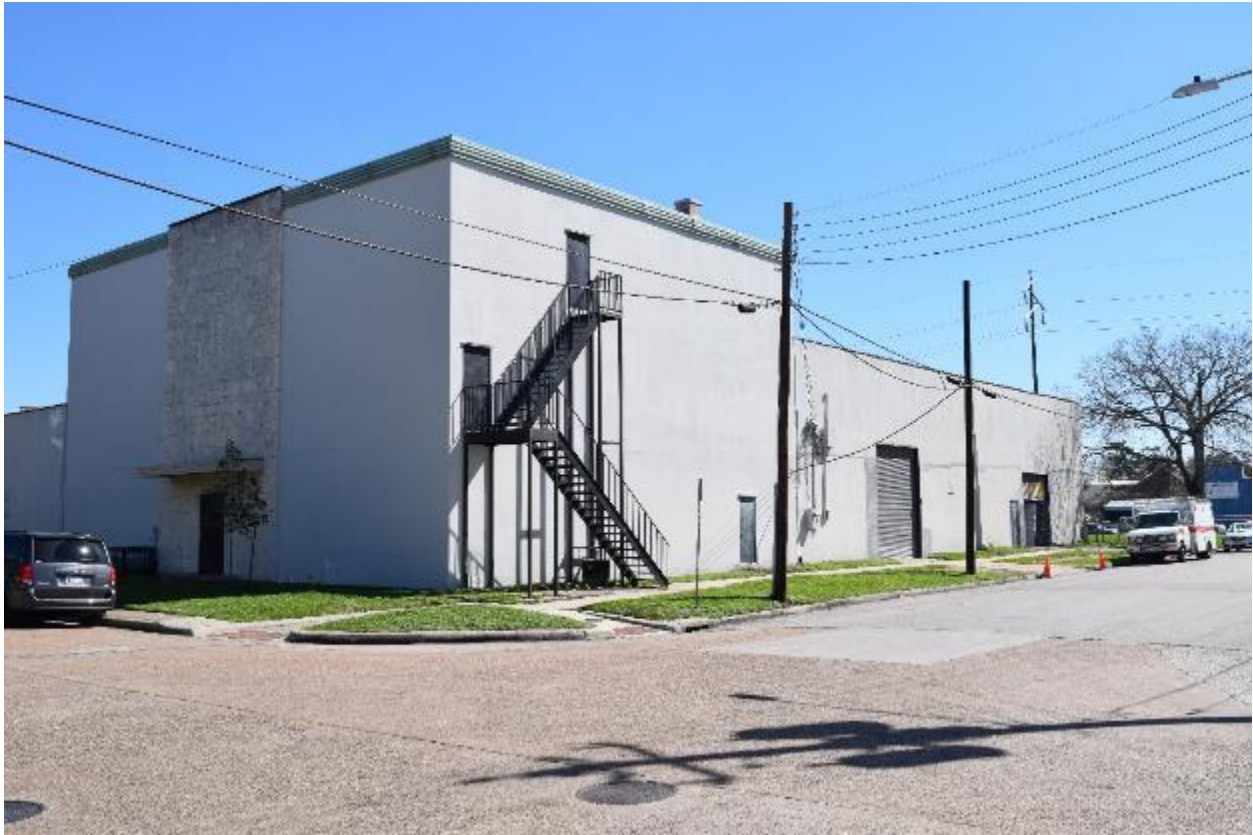
Photo 16 – West (front) and south elevations of Building #13 (left), view northeast, February 2017. South elevations for Buildings #15 and #19 are visible on right.
