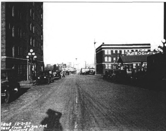
View looking east along Blanchard Street, December 2, 1930, after the final phase of regrading had been completed. The lower portion of the primary south façade of the Windham Apartments is visible at the left edge of the frame. (Seattle Municipal Archives Photograph Collection, item no. 4565.)
