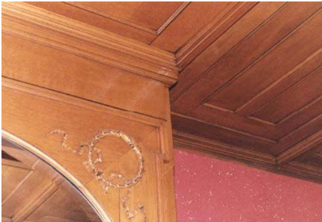
Wood Ceiling above Fireplace
