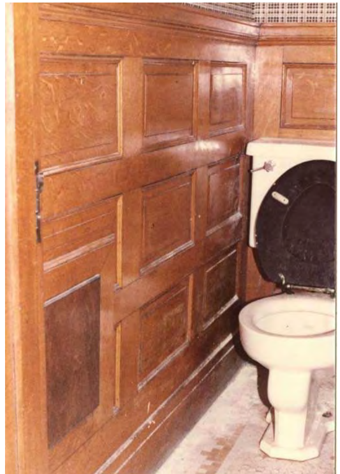
Wood Paneling in Restroom
