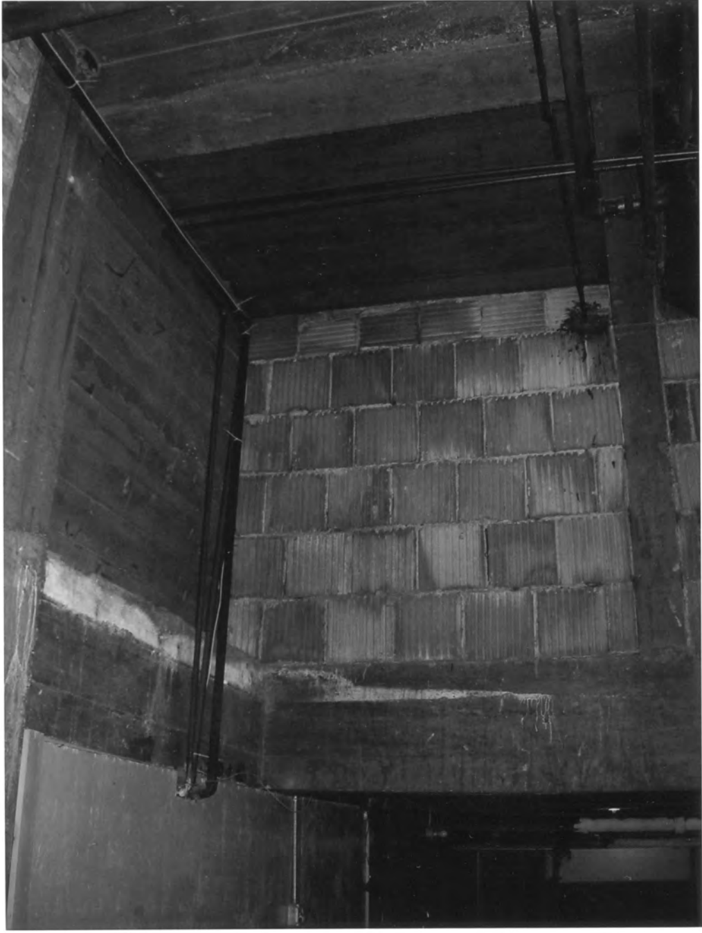
Southmoor Apartment Hotel, Lake Co., IN #15 (bottom of image to left)
