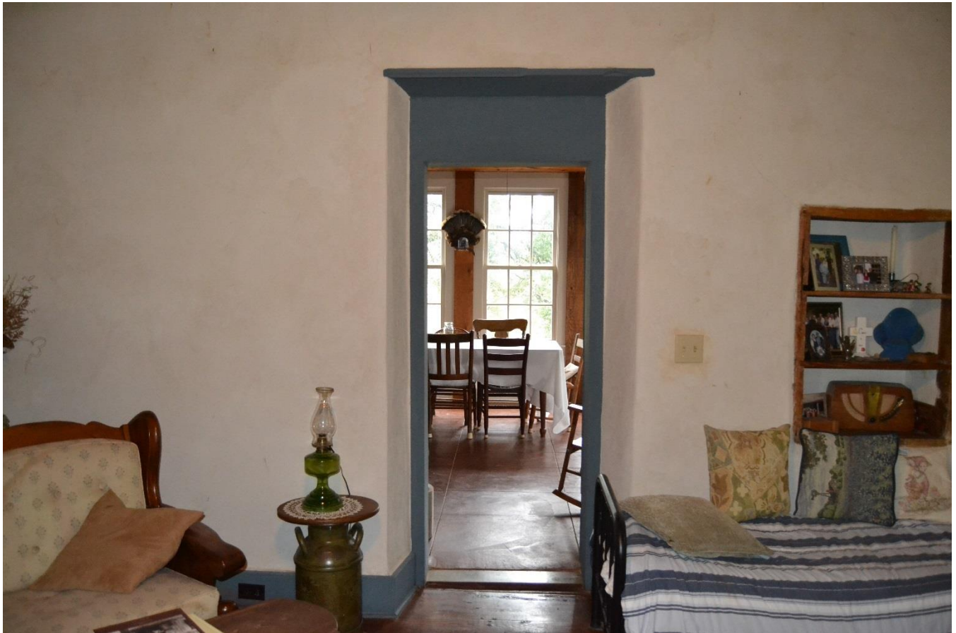
Photo No. 14. View of interior door to rear addition of house (RIDN 81039 a). Door was originally a window, view facing north.
