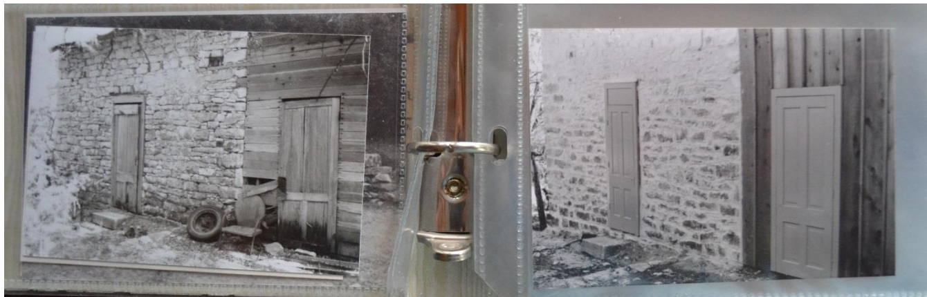
Figure 2. Photographs of north rear wall of Walzem house. Photograph on left shows center passage way enclosed with horizontal wood boards prior rehab work. Photograph on right shows center passage way enclosed with board-and-batten after rehab work. With the construction of the rear addition, the board-and-batten was removed and the passage way is now open. Source: Alton Rahe.
