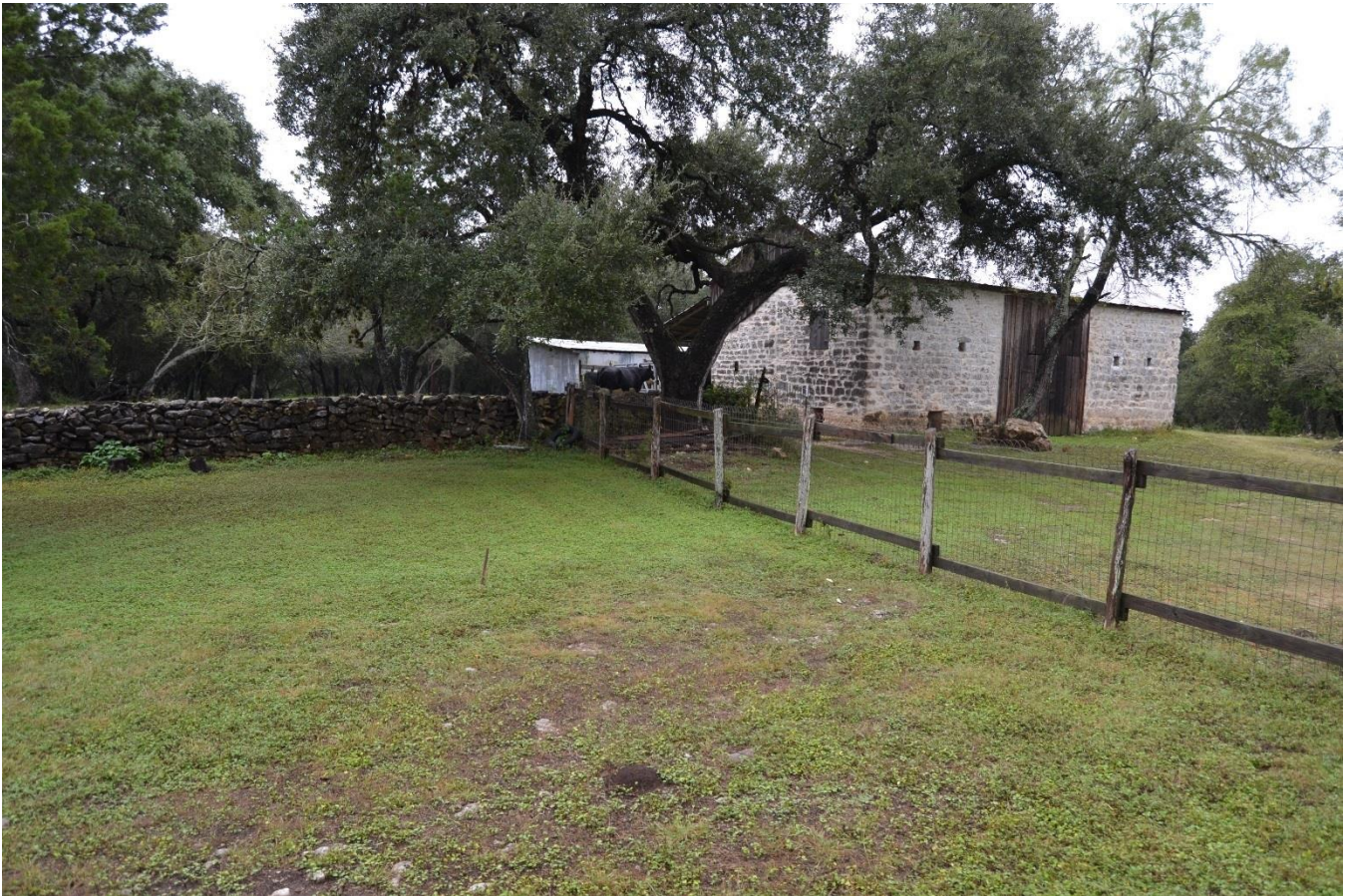
Photo No. 33. View of wood and wire fence (RIDN 81039 h) separating the area in front of the house from the barns, view facing southwest.
