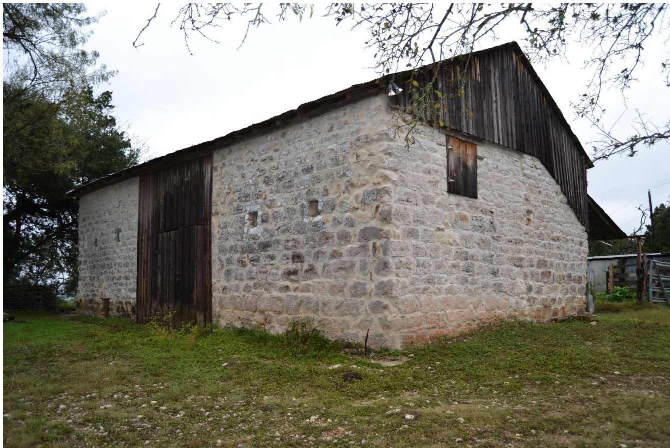
Photo No. 20. Oblique view of barn (RIDN 81039 b), view facing southeast.
