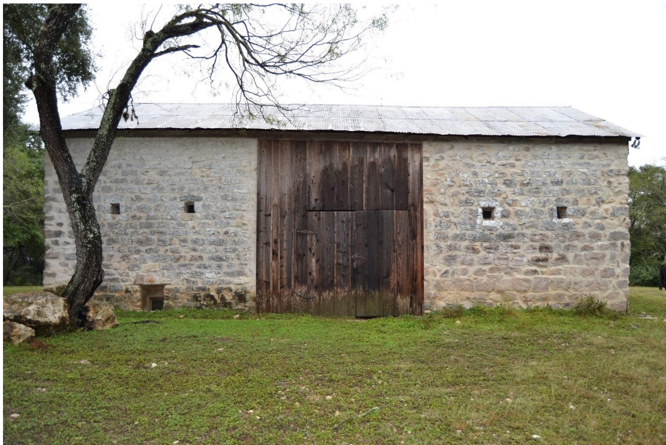
Photo No. 19. Front façade of barn (RIDN 81039 b), view facing southeast.
