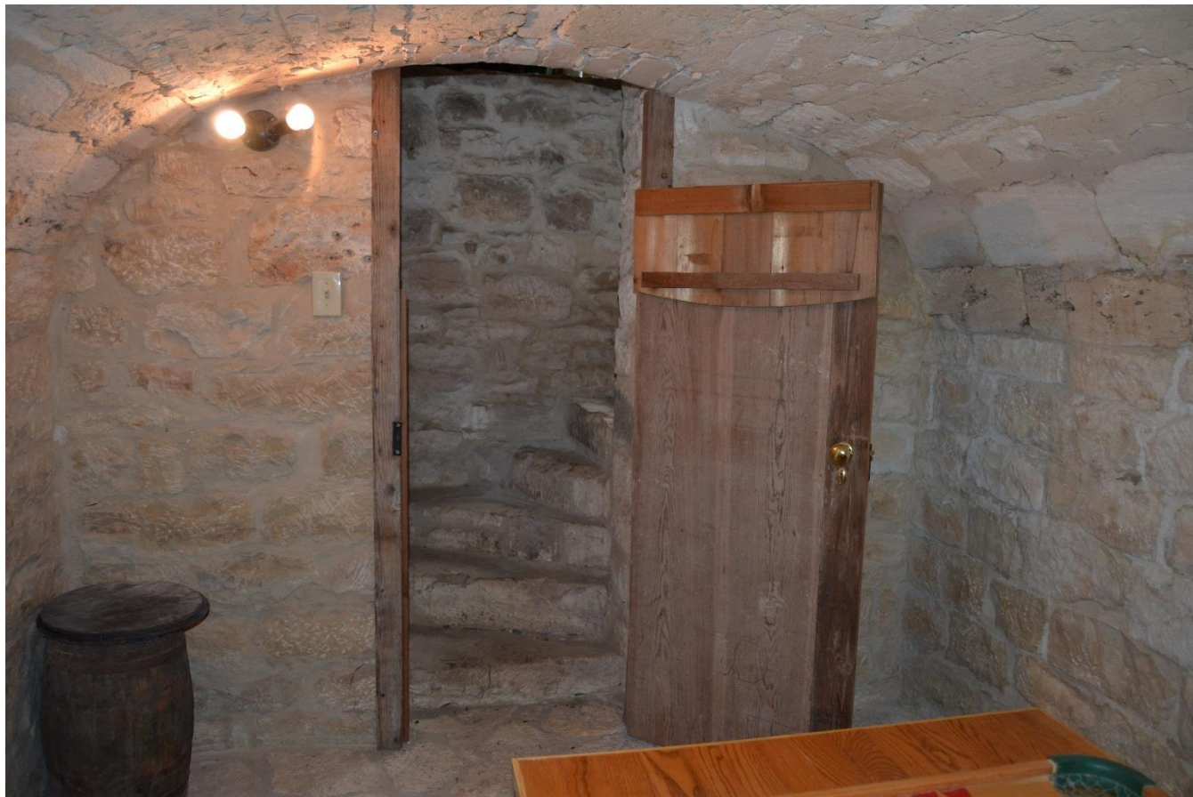
Photo No. 22. View of root cellar in barn (RIDN 81039 b) and curved stairway, view facing west.
