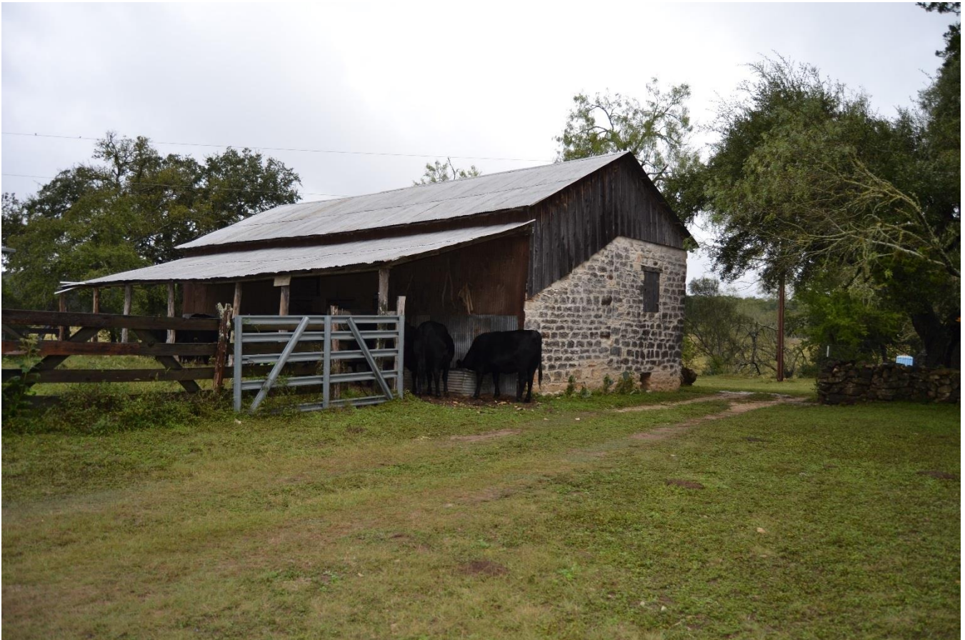
Photo No. 21. Oblique view of rear south façade of barn (RIDN 81039 b), view facing northwest.
