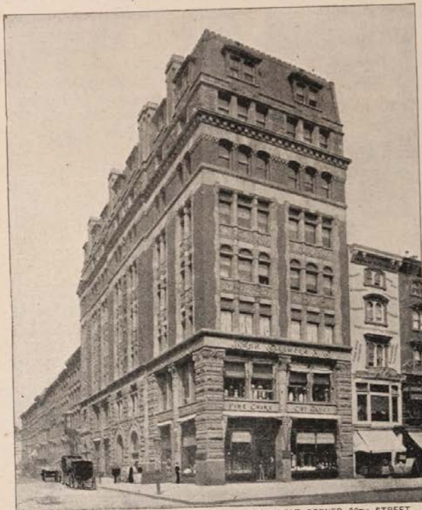
GILMAN COLLAMORE & CO., FIFTH AVENUE, NORTHWEST CORNER 30TH STREET.
