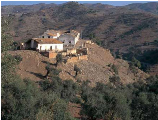
Figure 75: Aerial view of Cortijo Rosa Capilla in Almogía (Málaga), Spain, n.d.
