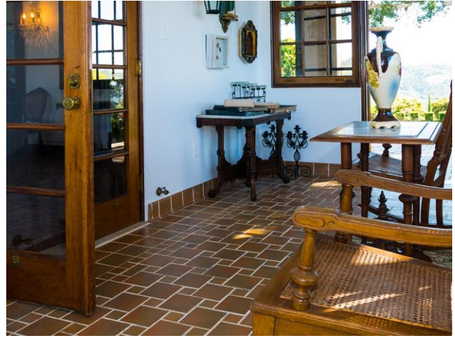
Figure 29: Detail of the sun porch floor arranged in the traditional hopscotch pattern (looking northeast), 2017.
