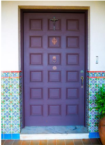
Figure 17: Mahogany door with eighteen entrepaños at the exterior foyer (looking west), 2017.
