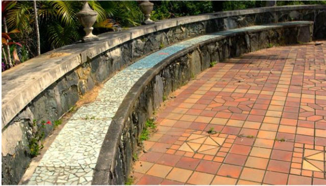
Figure 65: View of the curved bench facing the water fountain featuring the trencadís technique (looking northeast), 2017.
