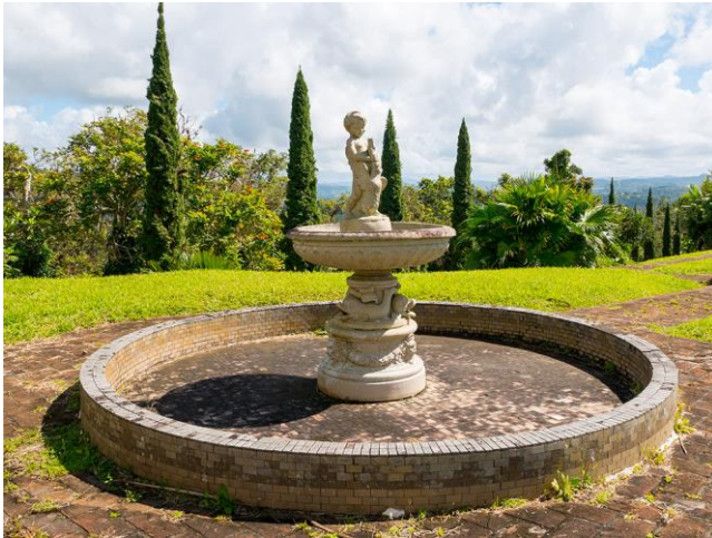
Figure 73: View of the glazed terracotta water fountain at El Cortijo (looking east), 2017.
