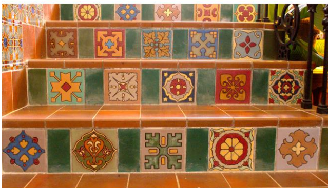
Figure 45: Detail of the main staircase steps, finished in terracotta quarry tiles and the risers are faced with Faience hand-decorated olambrillas (looking east), 2017.
