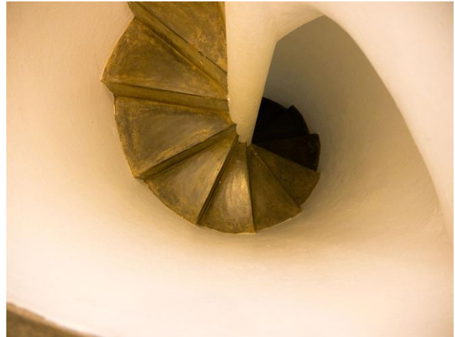
Figure 48: Detail of the concrete helical stairway in the tower (looking down), 2017.
