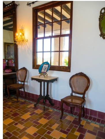
Figure 24: Detail of the floor finish at the living room, arranged in a modified hopscotch pattern surrounded by a Faience strip of floral motifs and a losetas border (looking north), 2017.
