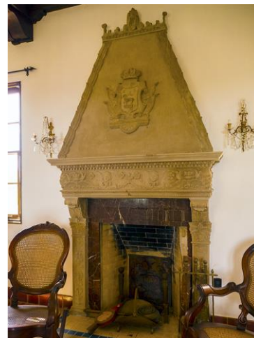
Figure 26: View of the stone carved trumeau fireplace (looking east), 2017.
