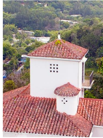
Figure 54: Detail of the fourth floor mirador and the square openings on its west façade (looking east), 2017.
