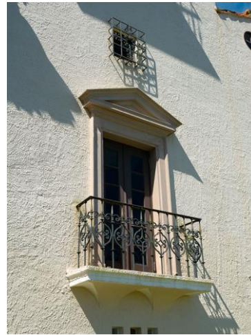
Figure 8: Detail of an open balcony at the main façade (looking west), 2017.
