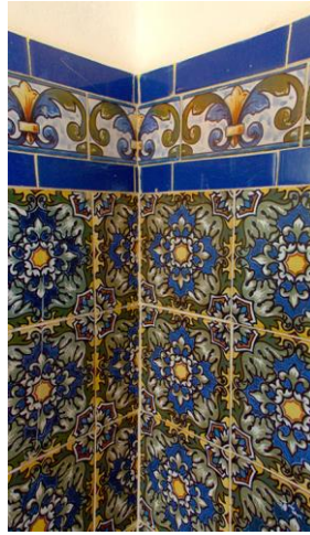
Figure 31: Detail of the wainscot in the formal dining room (looking northeast), 2017.
