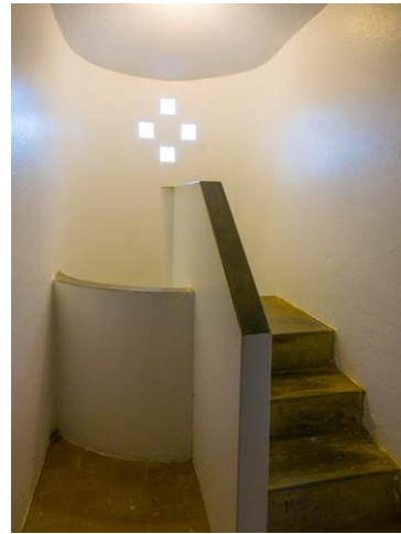
Figure 50: Detail of the steps and curved wall in the third level of the tower that protected the house from flooding in case of a cistern leakage (looking west), 2017.
