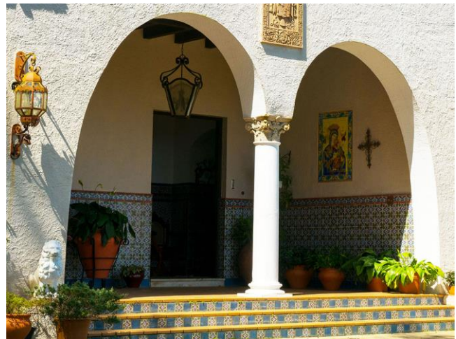
Figure 14: Close-up view of the elevated entrance foyer (looking west), 2017.
