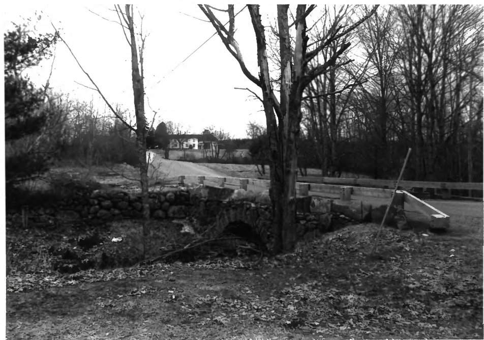
ARCH BRIDGE & LINCOLN CO., MAINE
