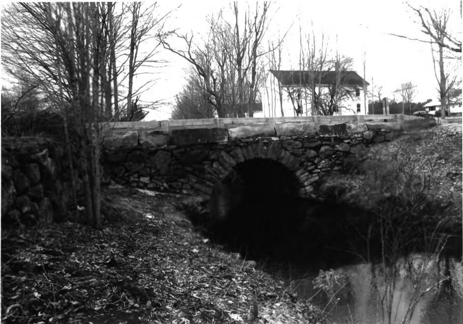
ARCH BRIDGE ; LINCOLN CO., MAINE
