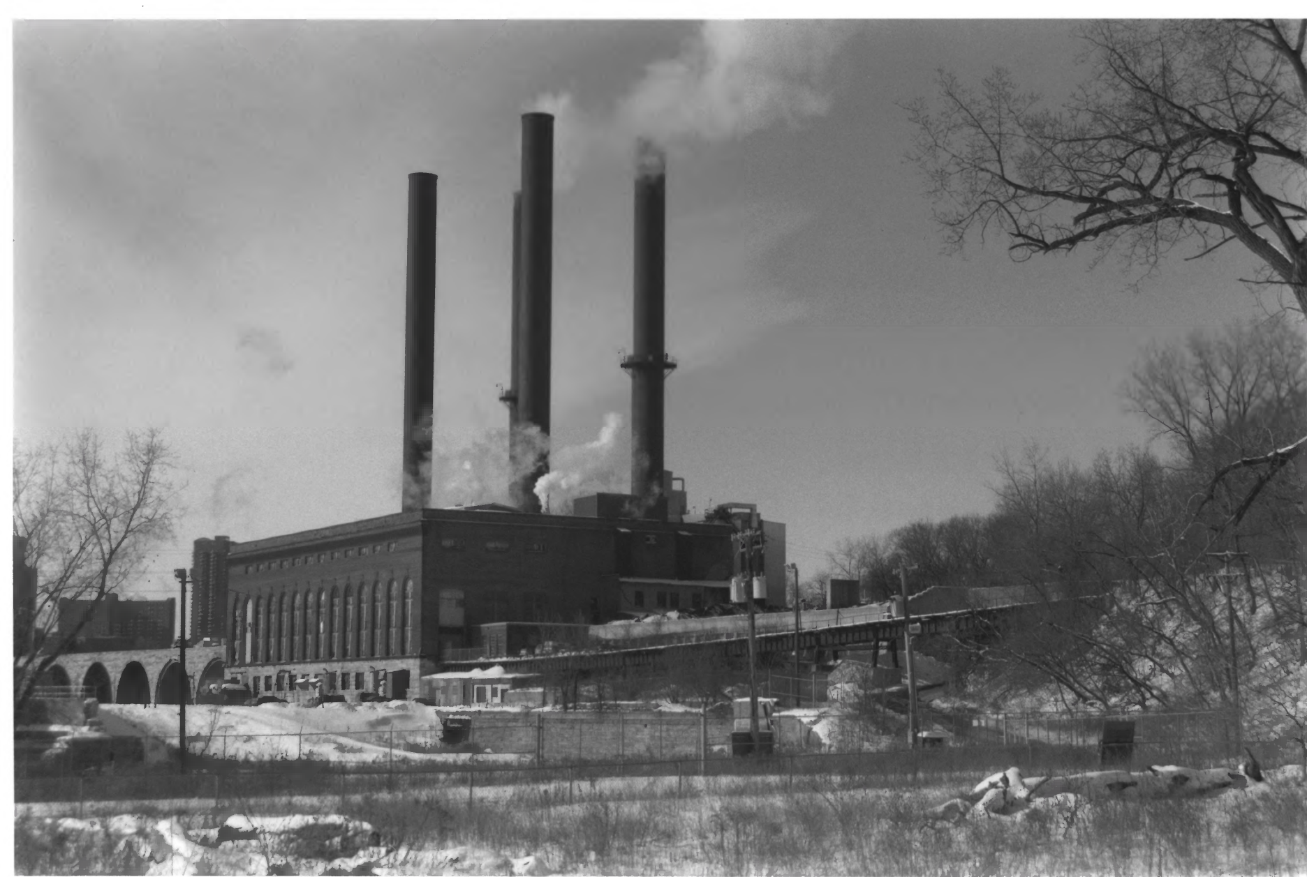
The Twin City Rapid Transit Steam Power Plant 12-20 Sixth Avenue Southeast, Minneapolis Hennepin County
