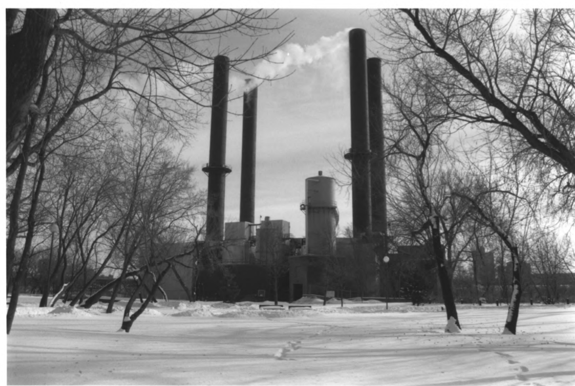
The Twin City Rapid Transit Steam Power Plant 12-20 Sixth Avenue Southeast, Minneapolis Hennepin County
