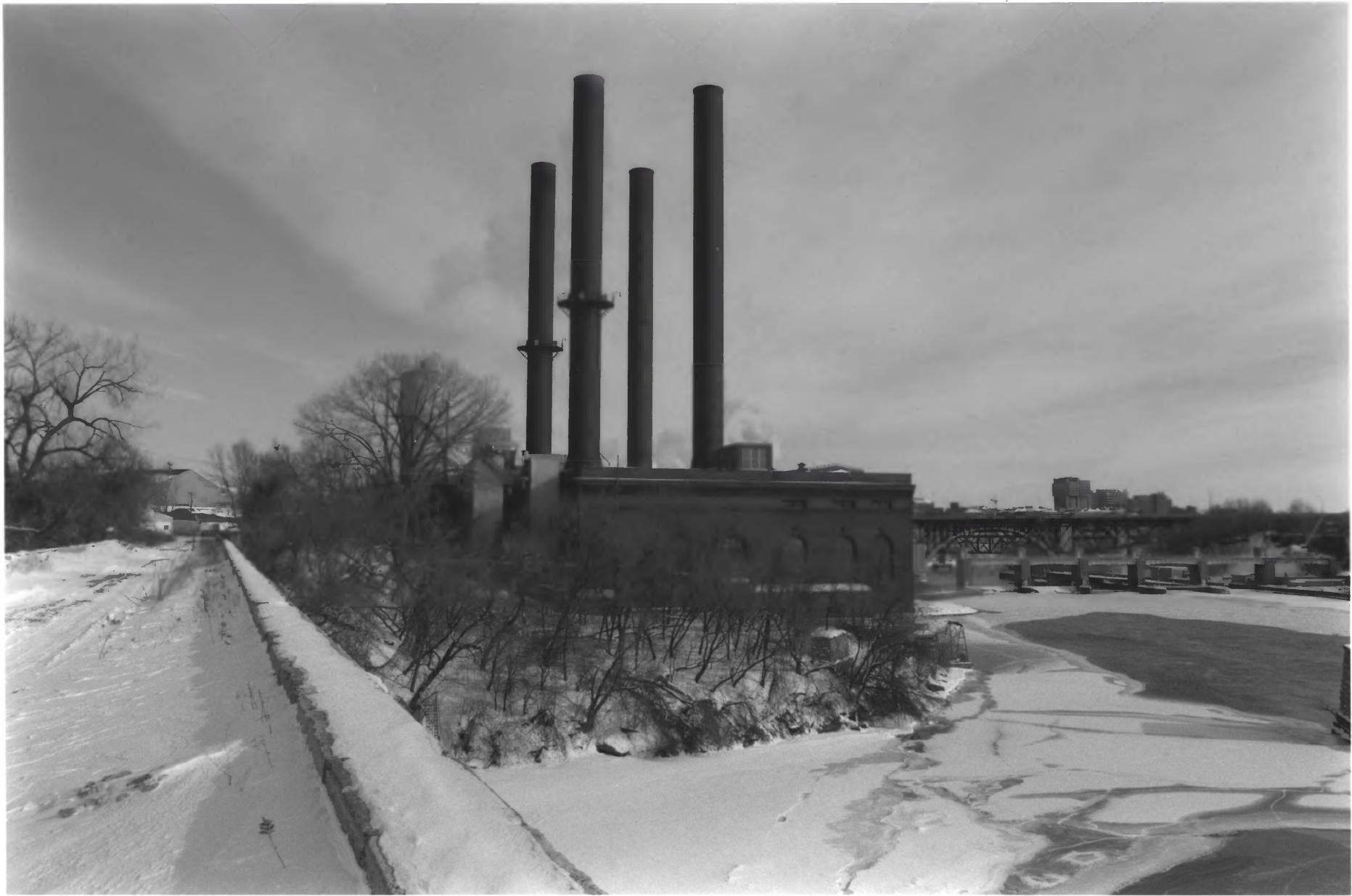
The Twin City Rapid Transit Steam Power Plant 12-20 Sixth Avenue Southeast, Minneapolis Hennepin County
