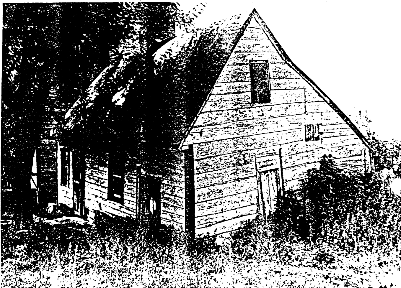
Stagg Hall. View of kitchen wing from southeast. Ca. 1930s. HABS photograph.
