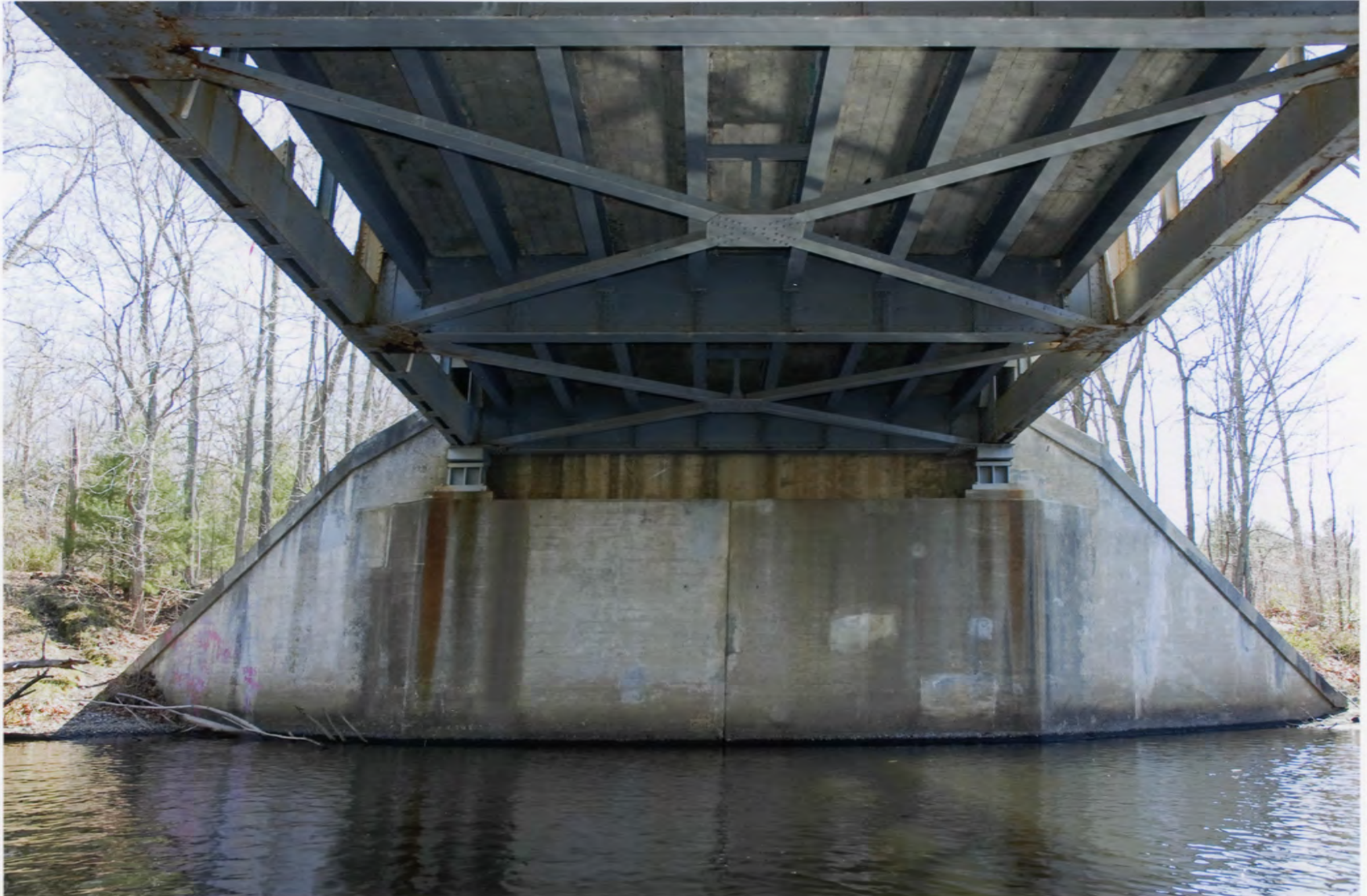
Butts Bridge, Windham County, CT
