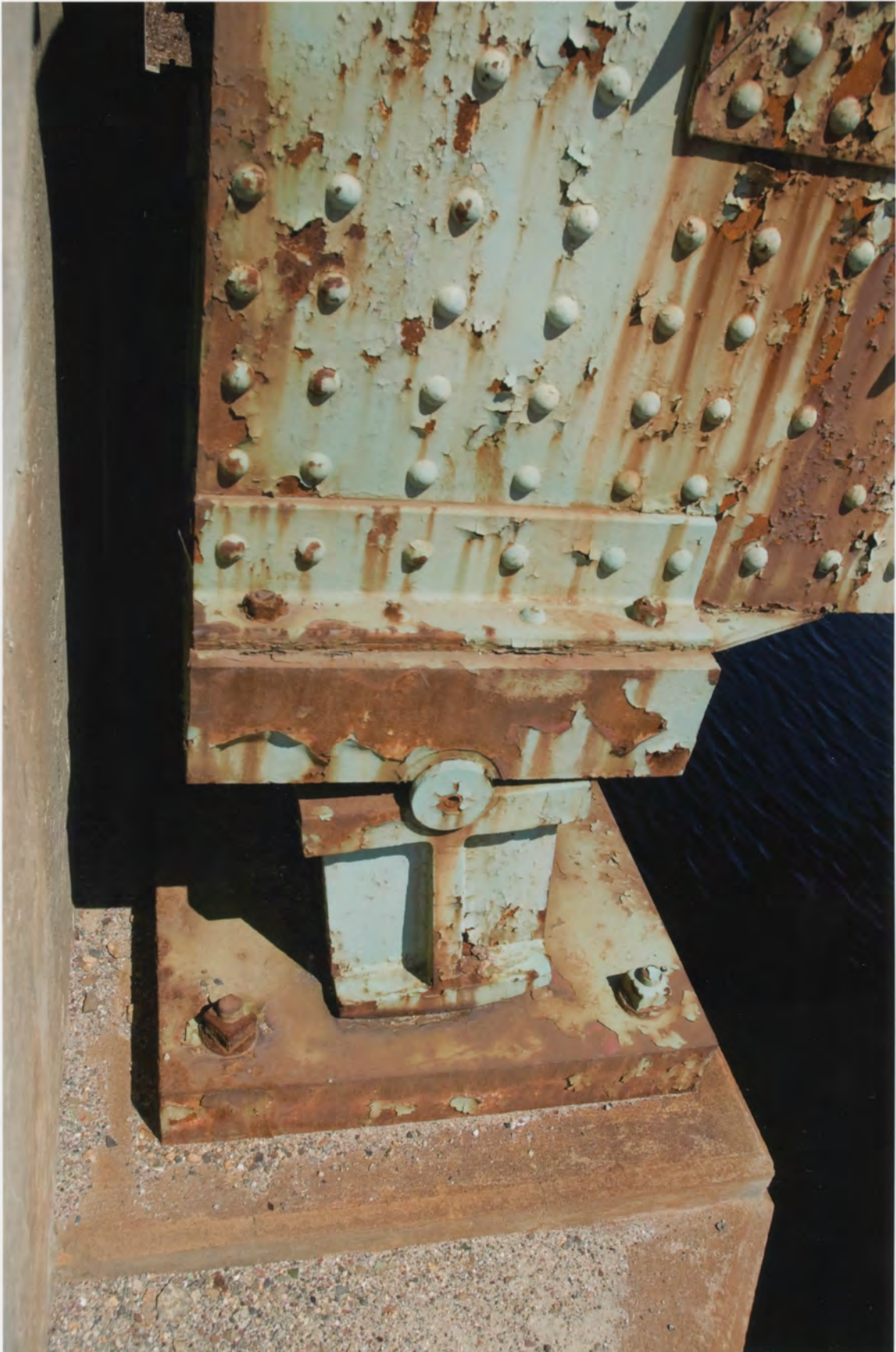
Butts Bridge, Windham County, CT
