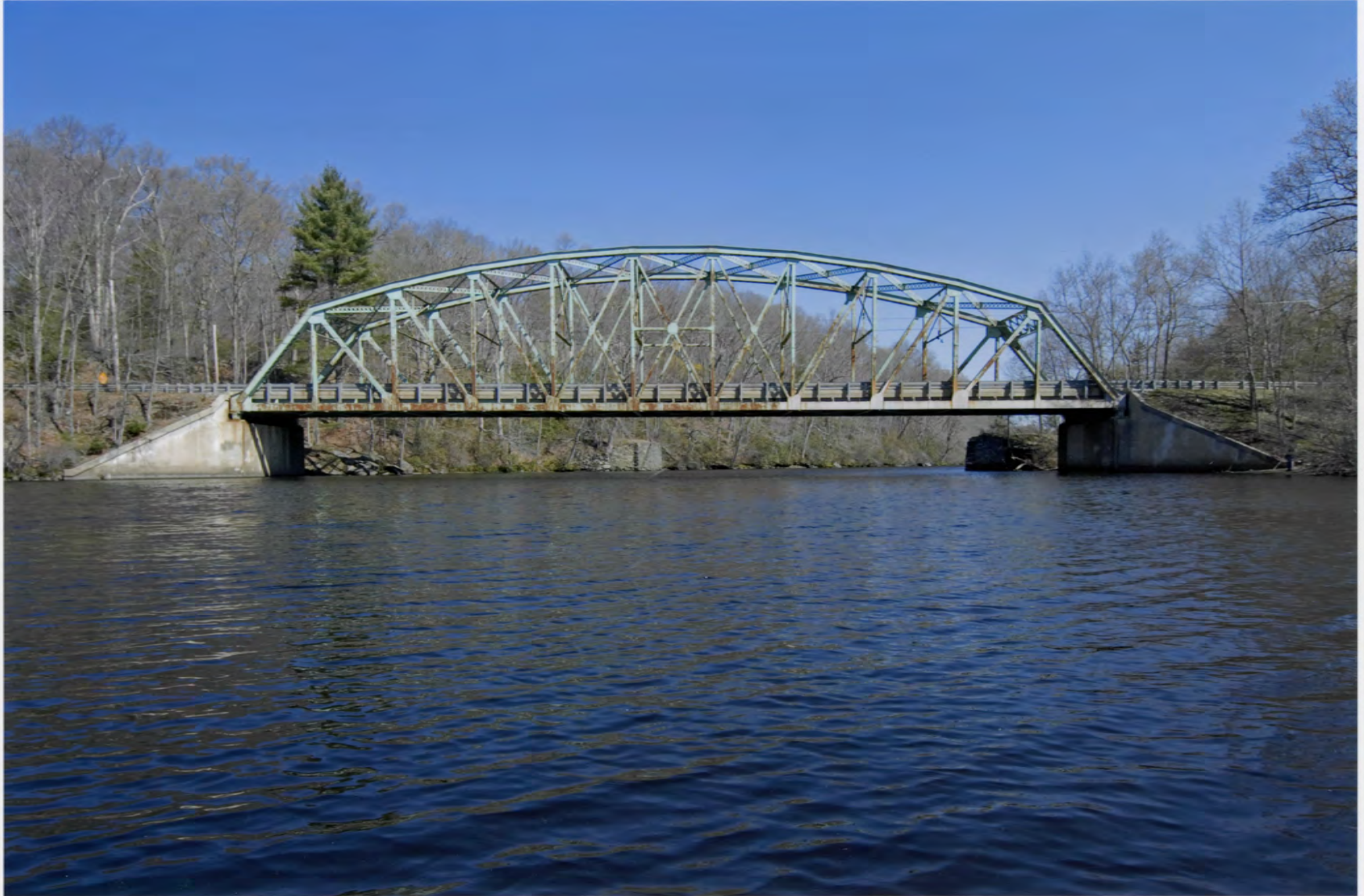
Butts Bridge, Windham County, CT
