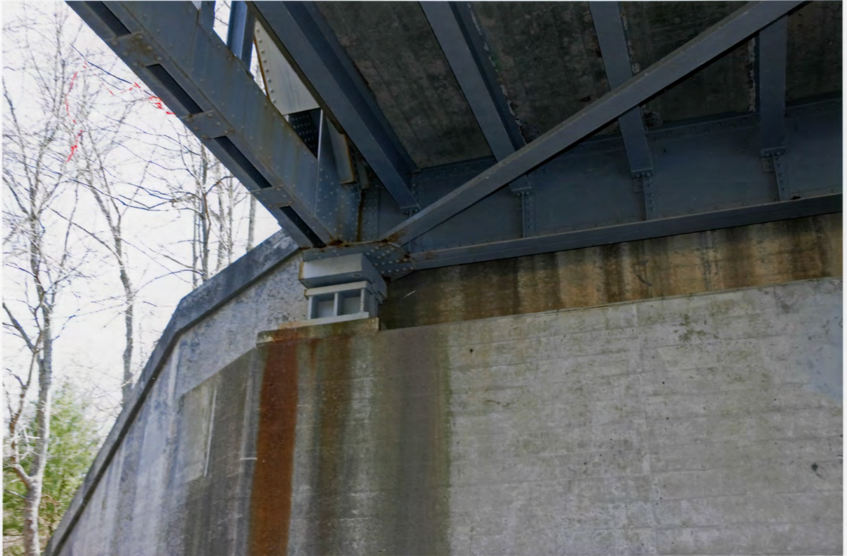
Butts Bridge, Windham County, CT
