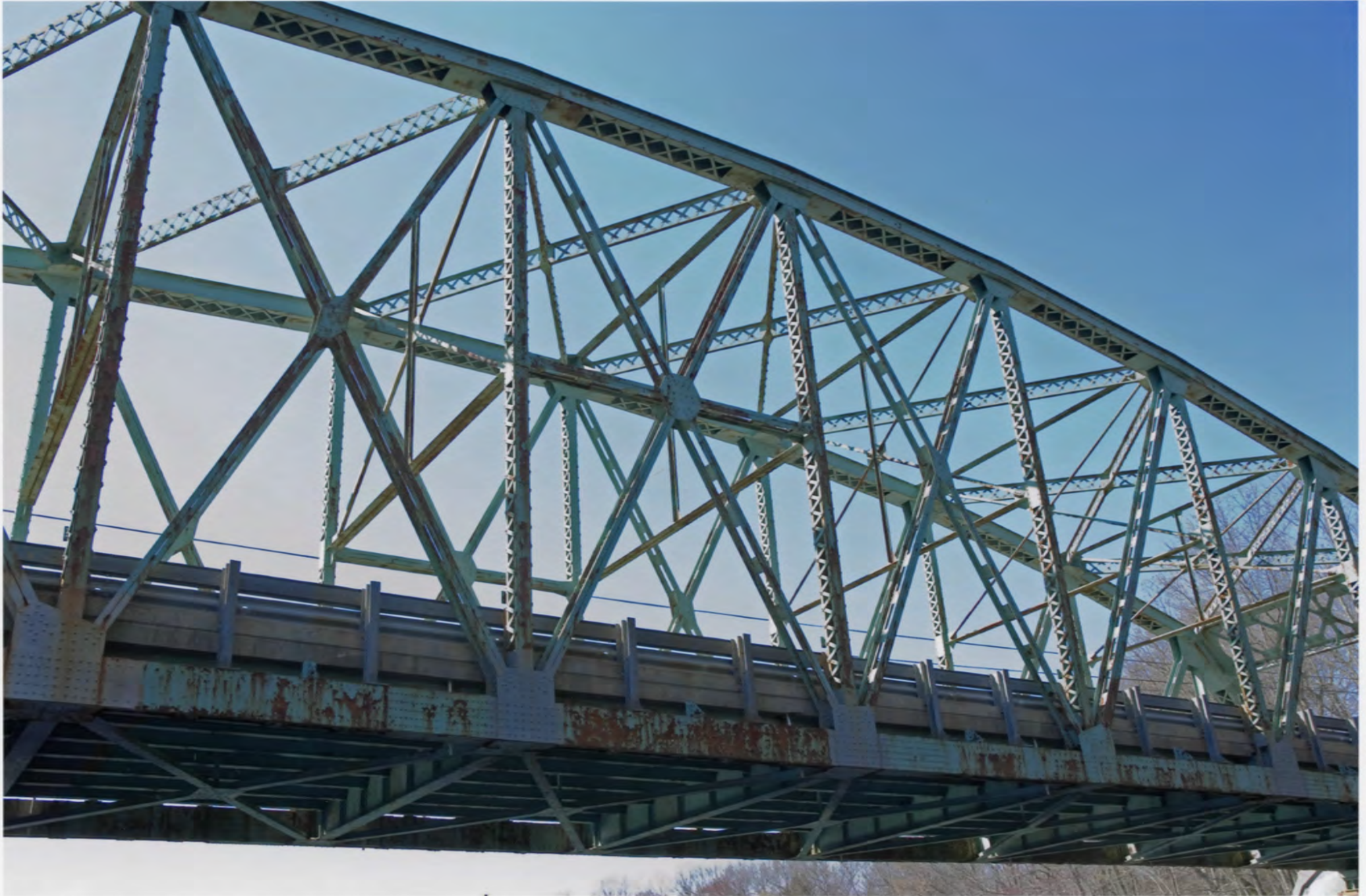
Butts Bridge, Windham County, CT
