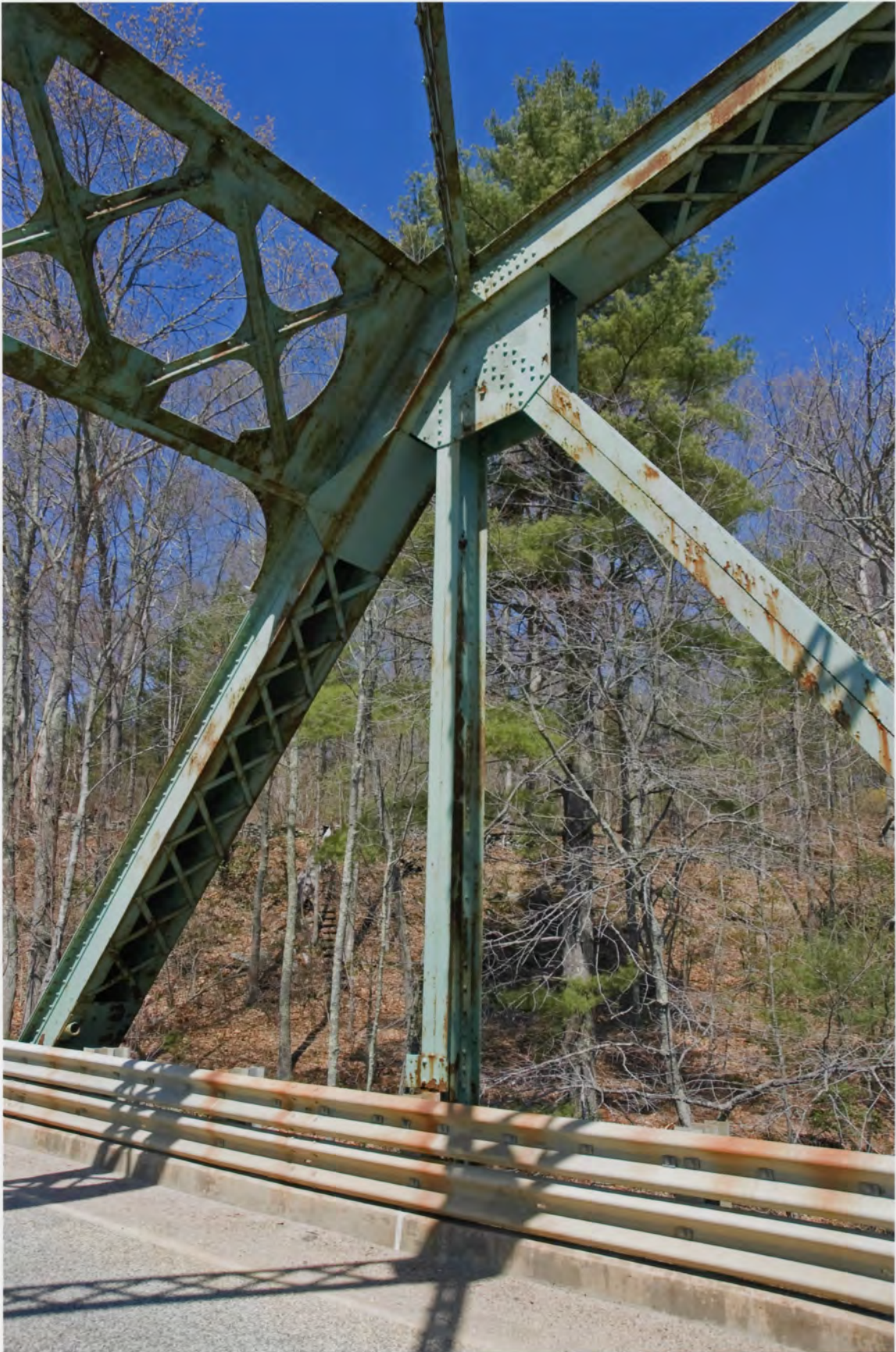
Butts Bridge, Windham County, CT
