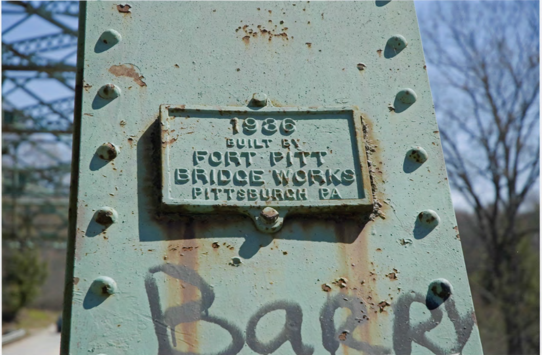
Butts Bridge, Windham County, CT
