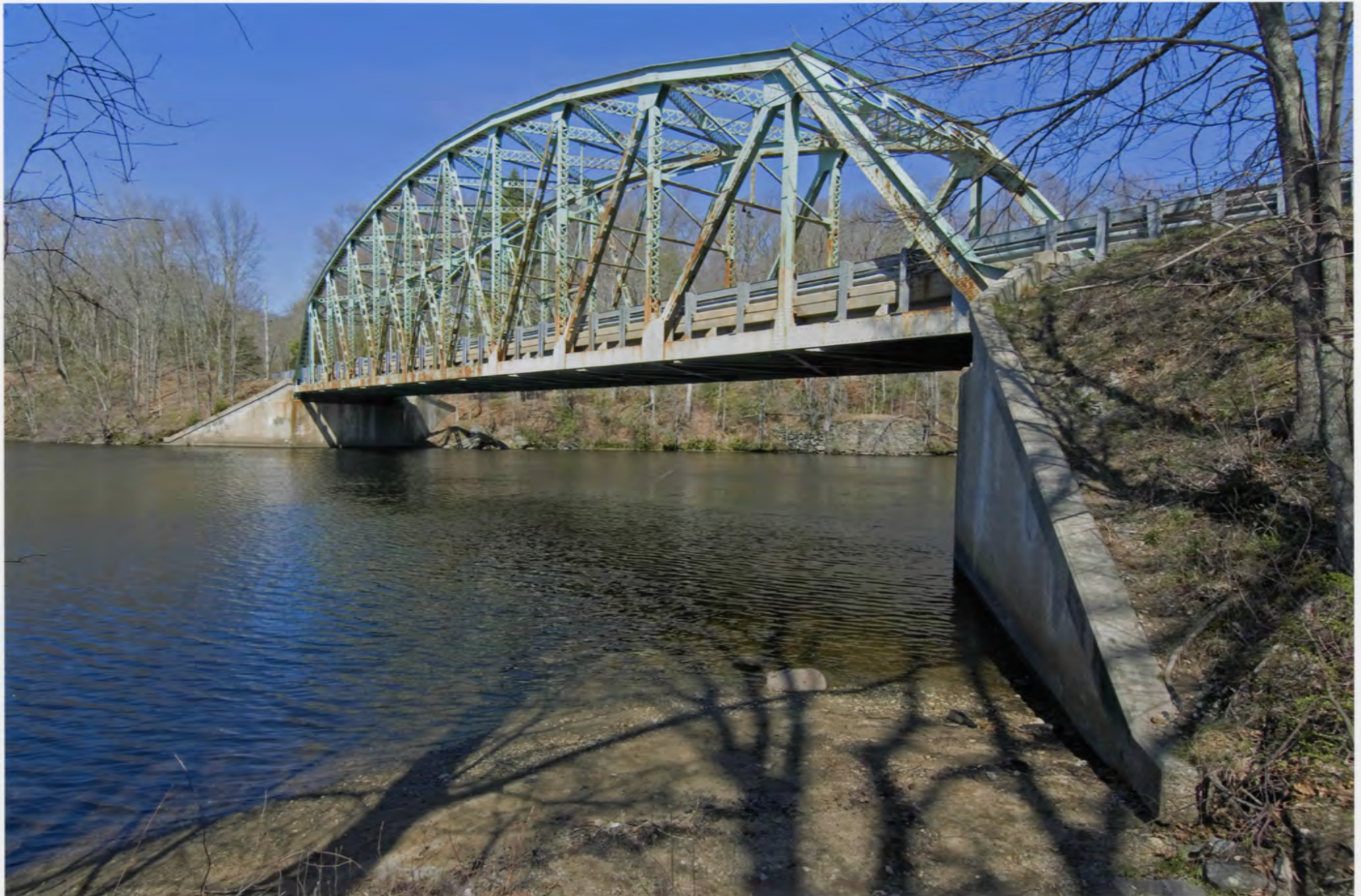
Butts Bridge, Windham County, CT
