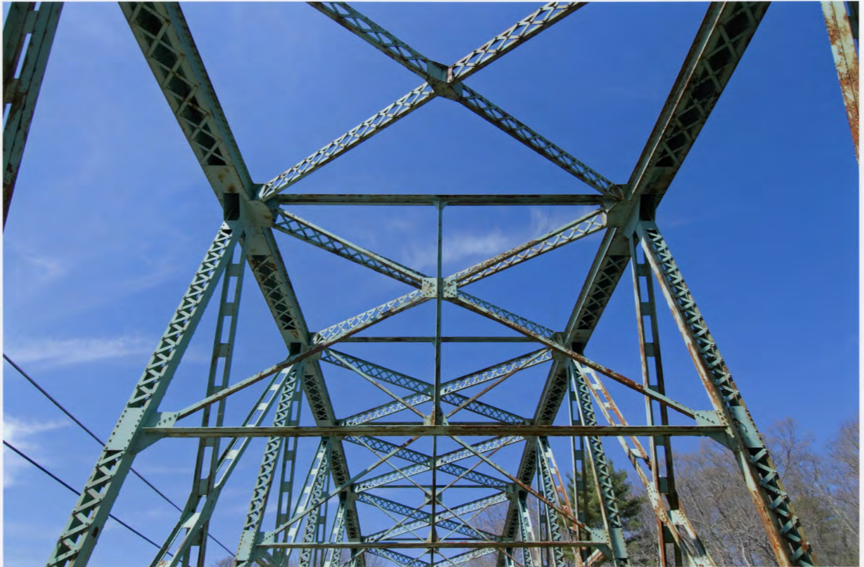
Butts Bridge, Windham County, CT
