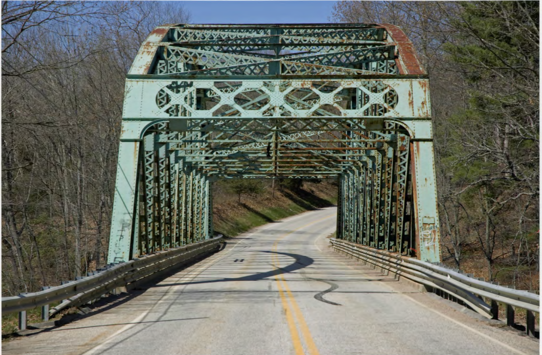
Butts Bridge, Windham County, CT
