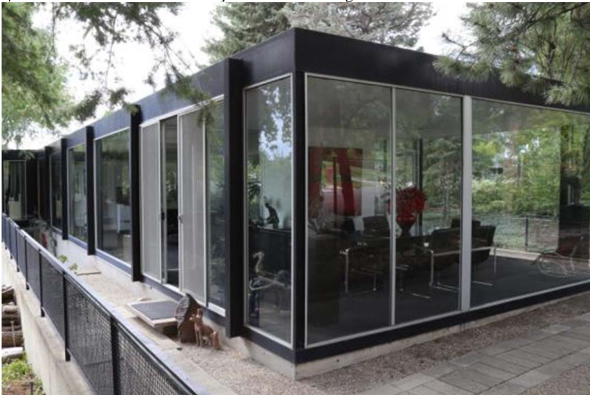
Photograph 6 of 20. View of Southeast Façade. Camera facing northwest.
