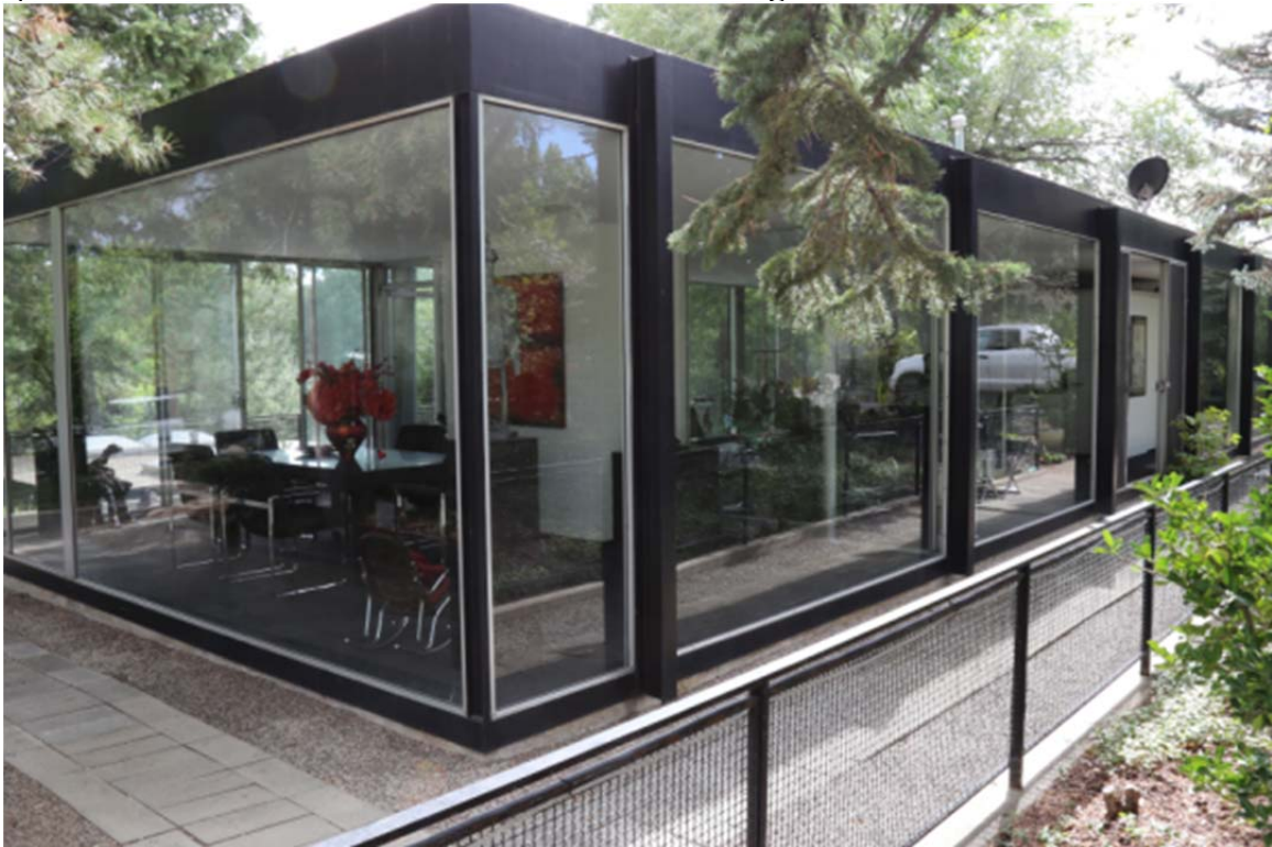
Photograph 1 of 20. View of Northeast elevation. Camera facing southwest.
