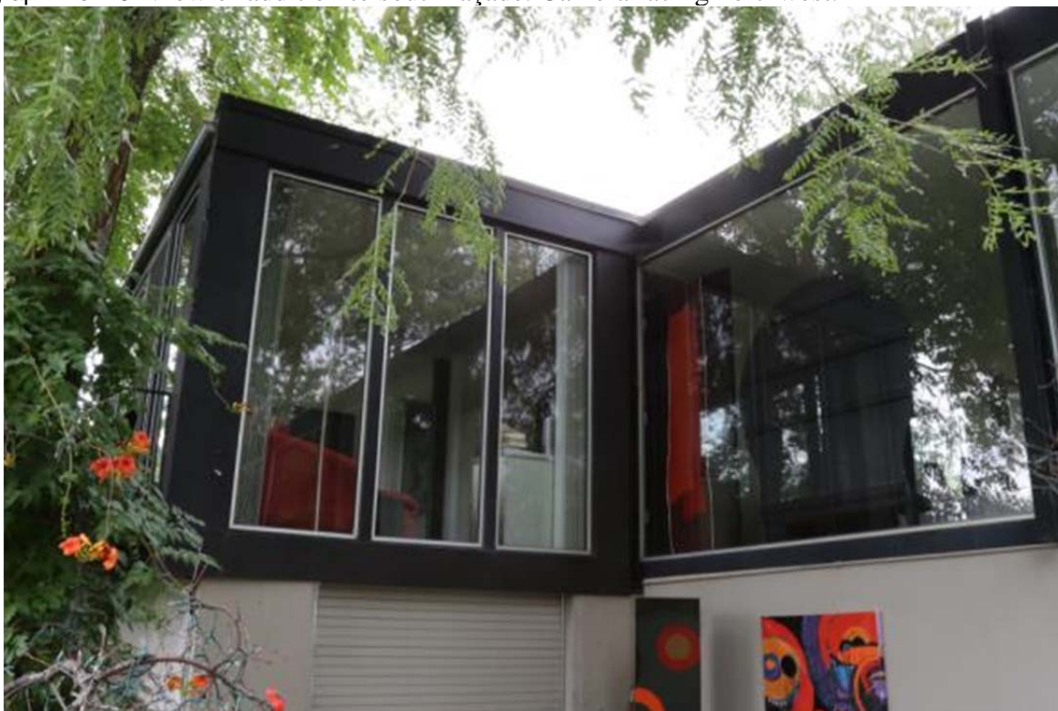
Photograph 7 of 20. View of addition to south façade. Camera facing northwest.
