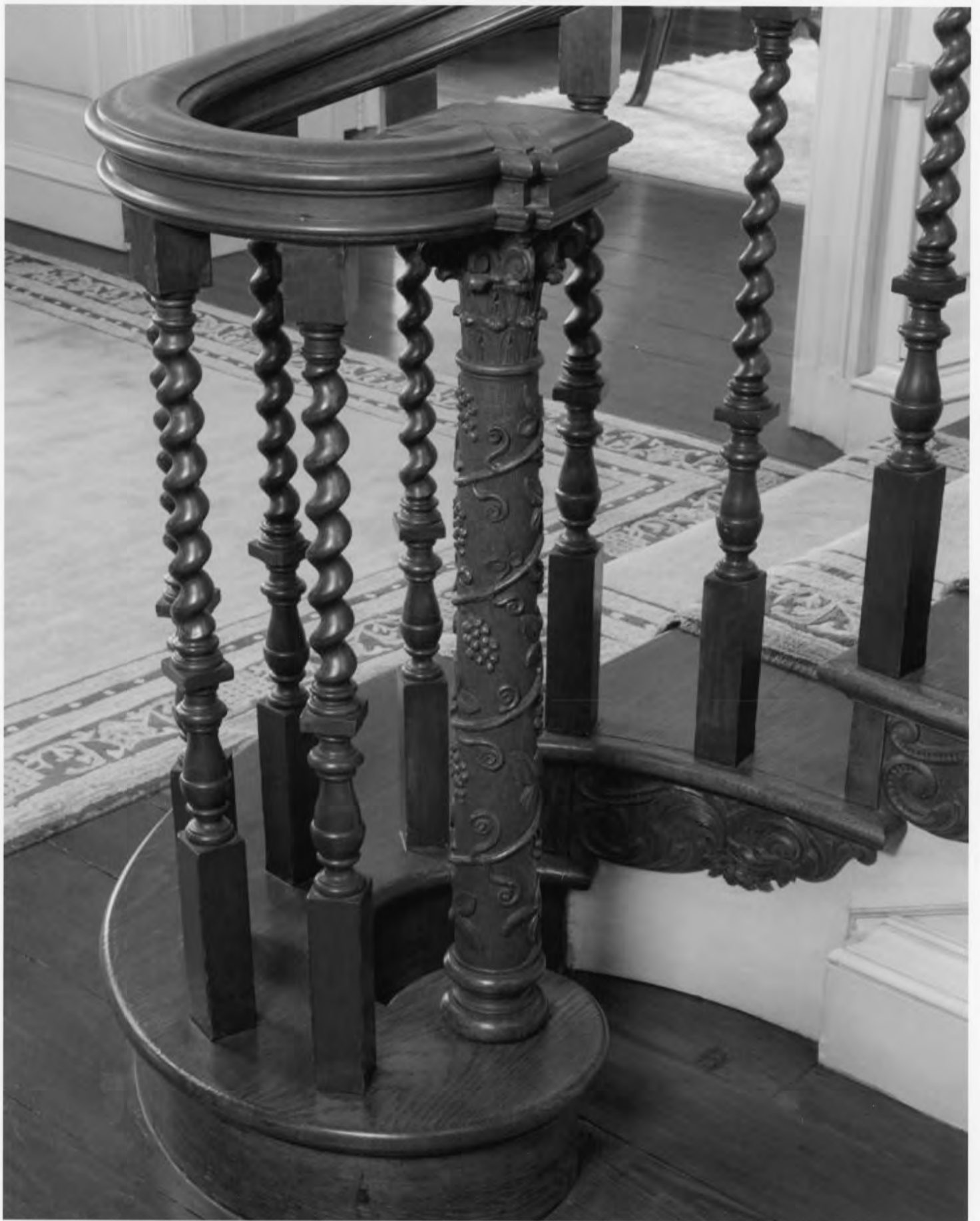
DE_New Castle County_Stockton/Montmorency newel post of staircase in center hall 18 of 49
