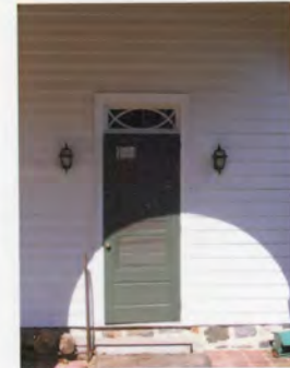
façade entrance - caretaker's cottage (shadow – brick arch support)
