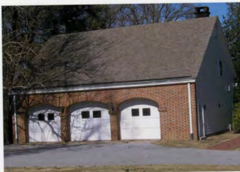
new, three-bay frame garage with brick veneer
