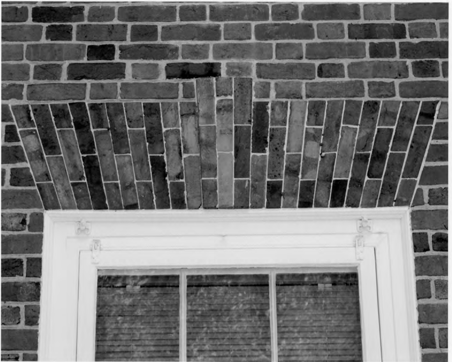
DE_New Castle County_Stockton/Montmorency detail - gauge brick lintel west facade 12 of 49
