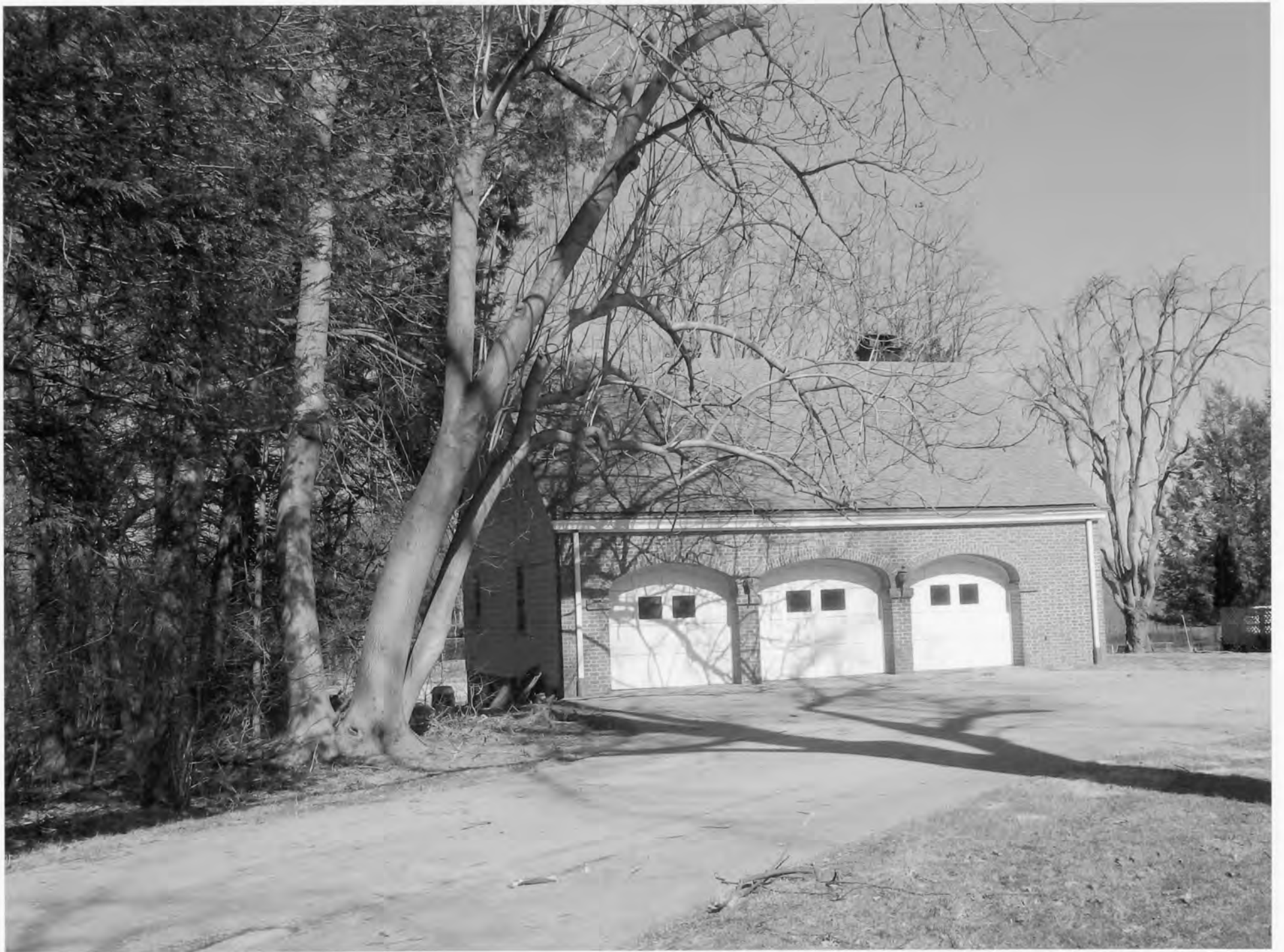
DE_New Castle County_Stockton/Montmorency new three-car garage north of house 46 of 49
