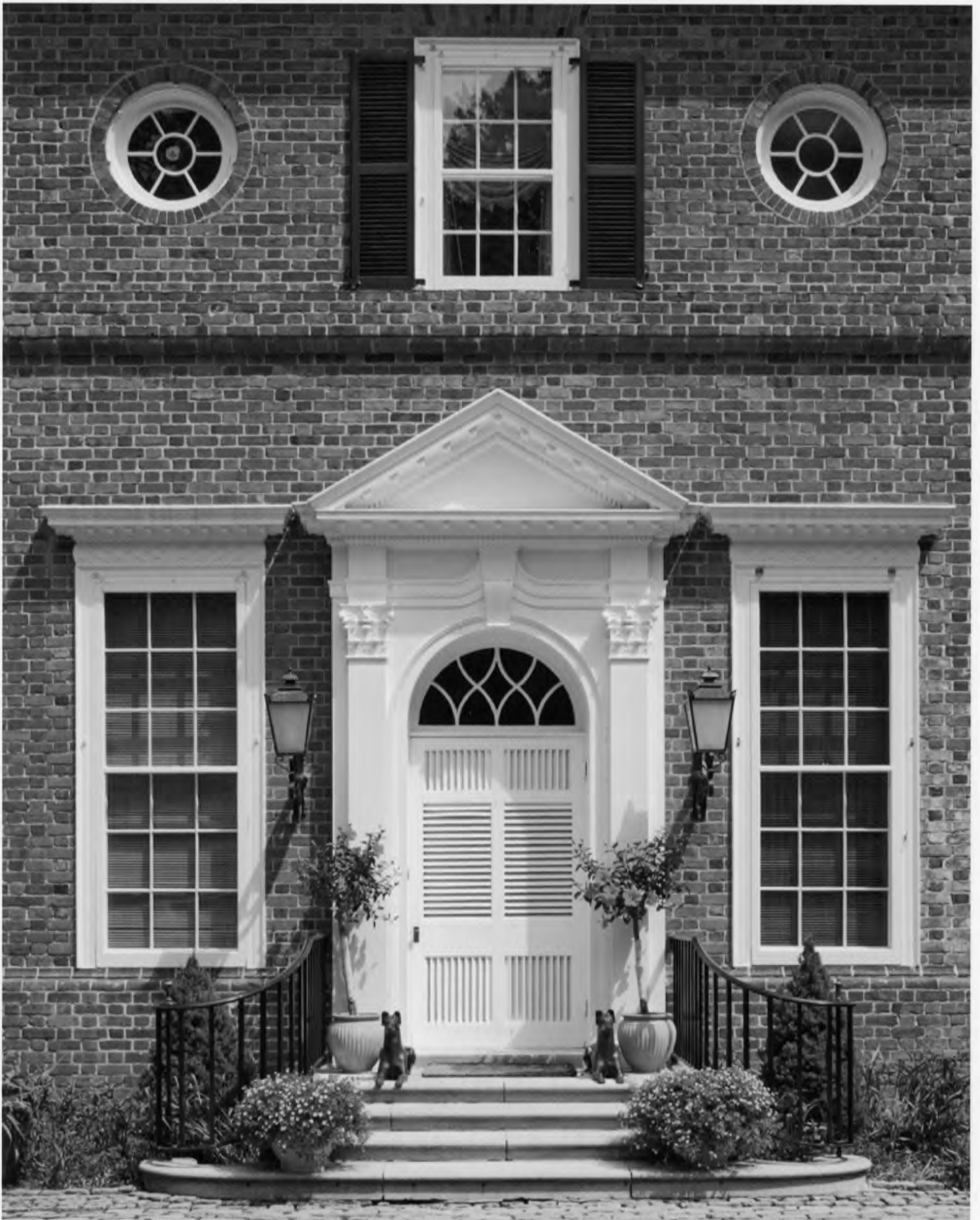
DE_New Castle County_Stockton/Montmorency detail - west facade entrance 10 of 49
