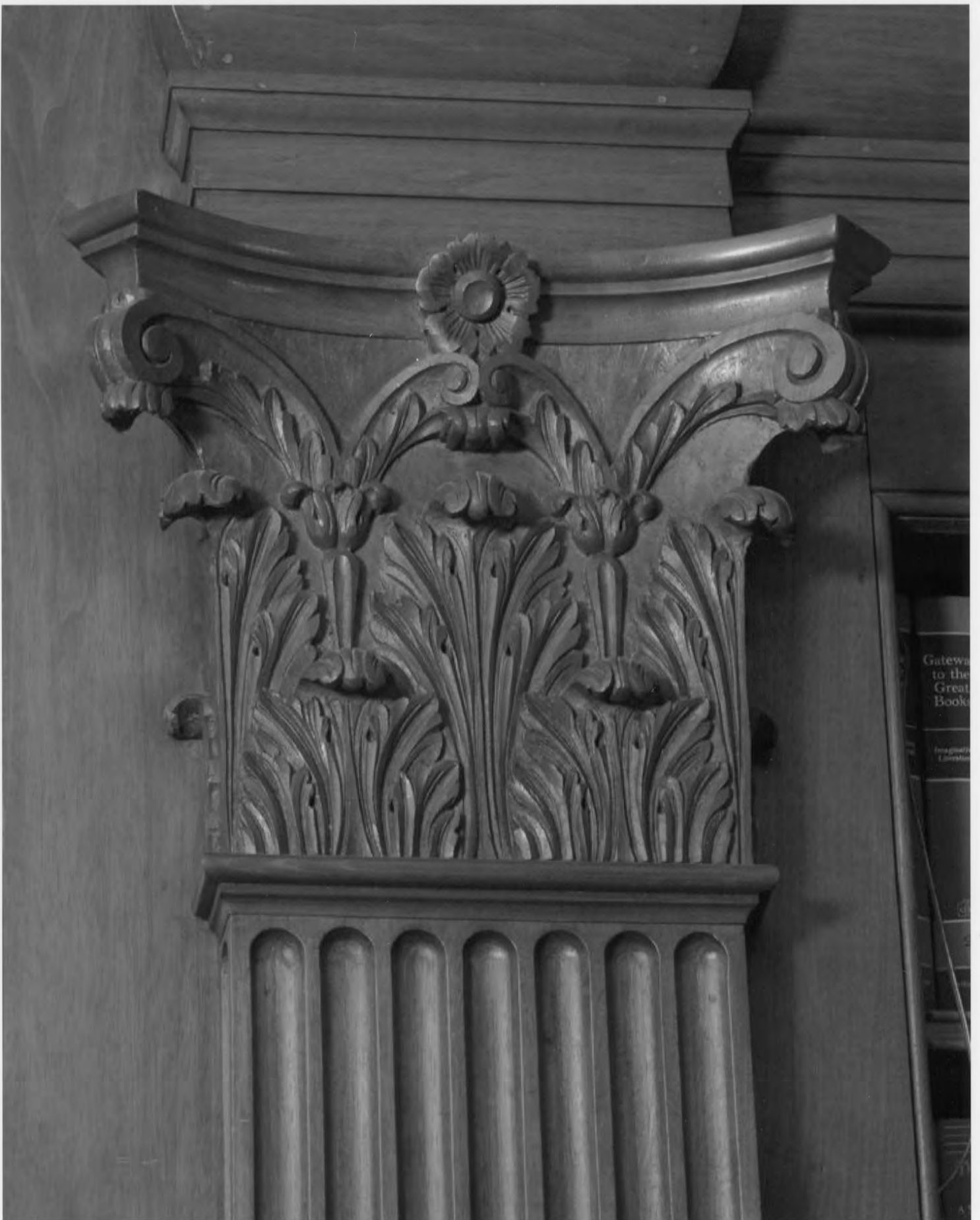
DE_New Castle County_Stockton/Montmorency detail- ornate pilaster - library
