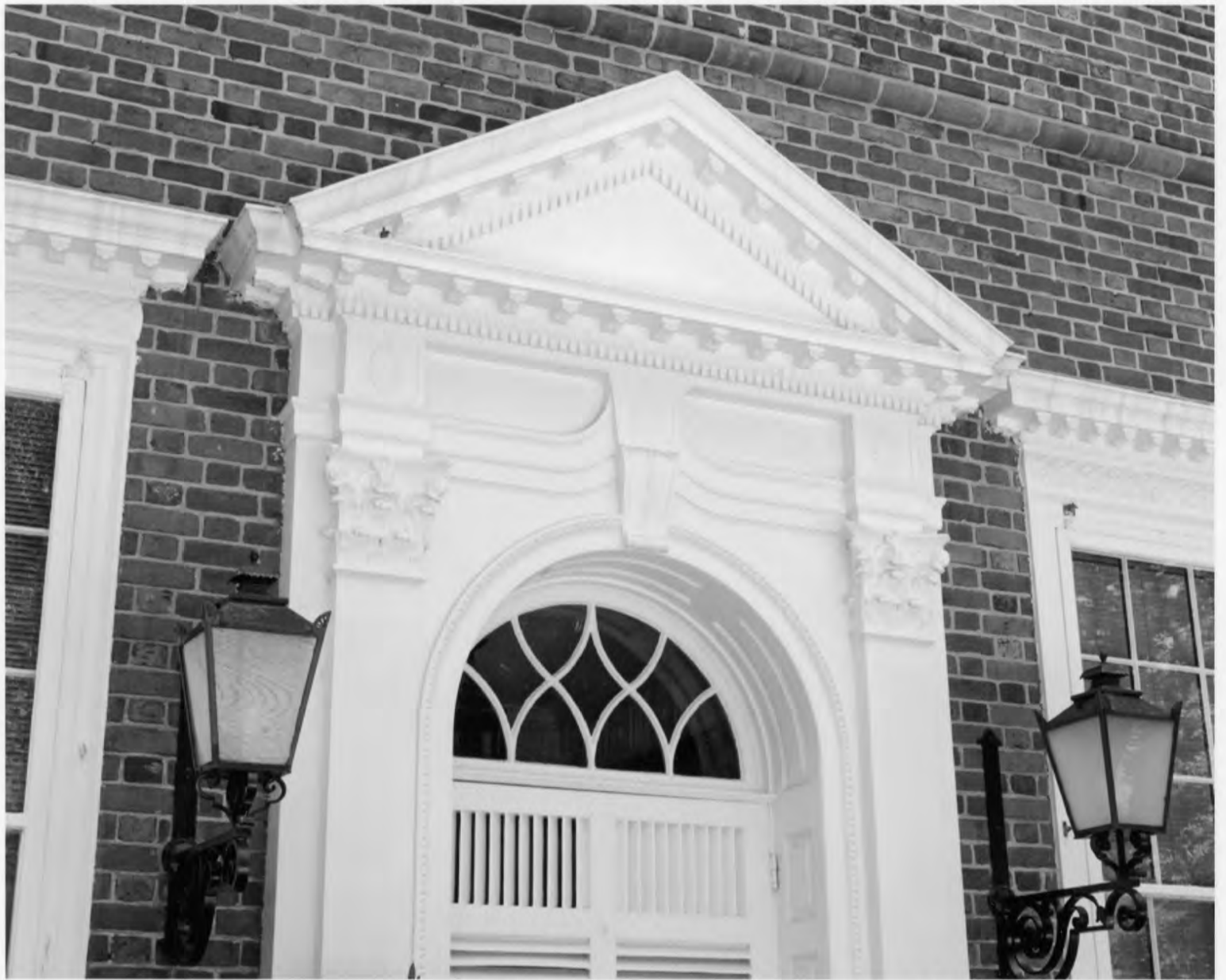
DE_New Castle County_Stockton/Montmorency detail of decorative elements - west entrance 11 of 49
