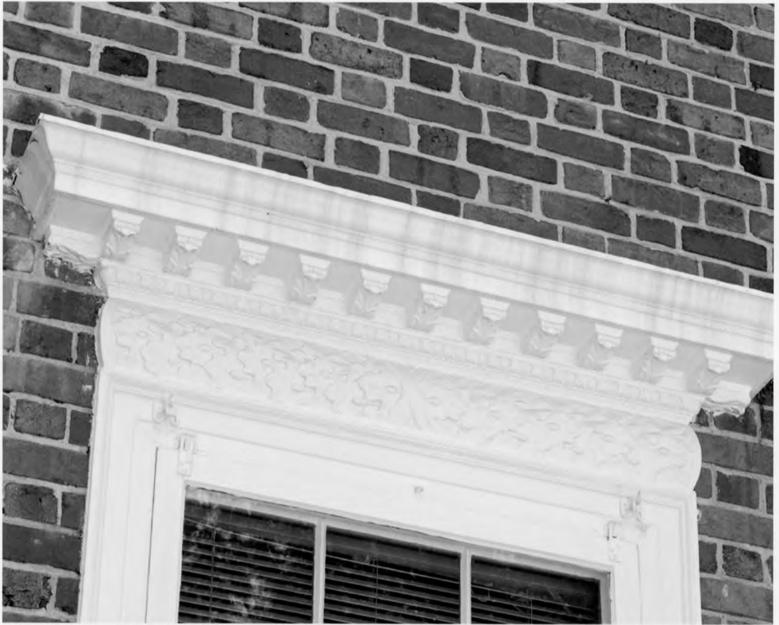
DE_New Castle County_Stockton/Montmorency detail -window lintel and cornice west facade 13 of 49
