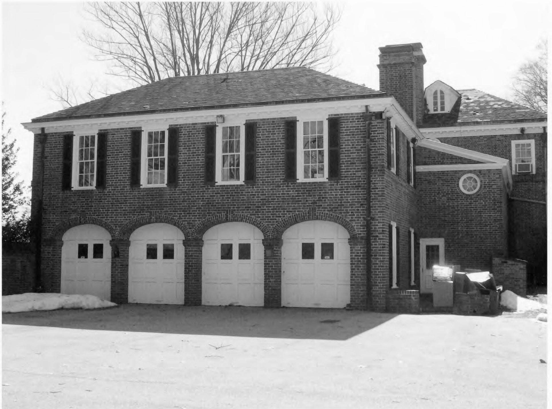
DE_New Castle County_Stockton/Montmorency north end of house, section of hyphen, and three-car garage
