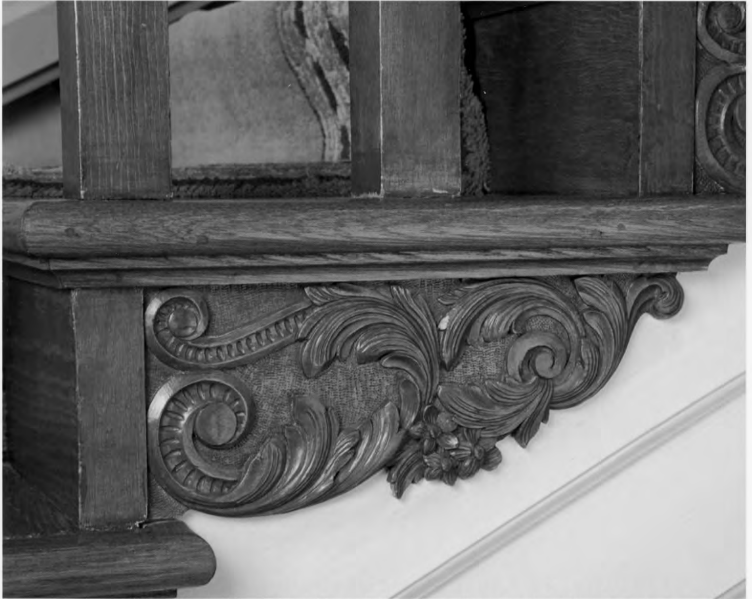
DE_New Castle County_Stockton/Montmorency decorative edge of staircase - center hall 19 of 49
