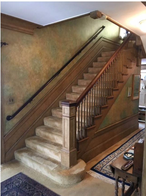
Photo #13 of 25 (WA_King County_Hannah Lewis House_0013) Staircase from entry foyer to second floor, camera facing southeast
