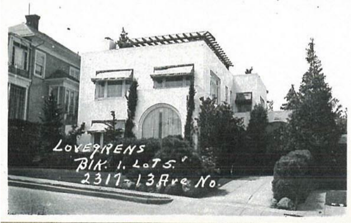
King County Assessor Photo – c. 1948. Note 3 rd floor pergola
