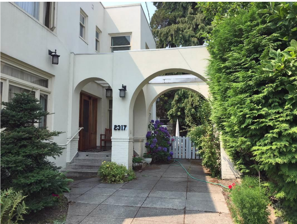
Photo #3 of 25 (WA_King County_Hannah Lewis House_0003) Porte cochere, camera facing west
