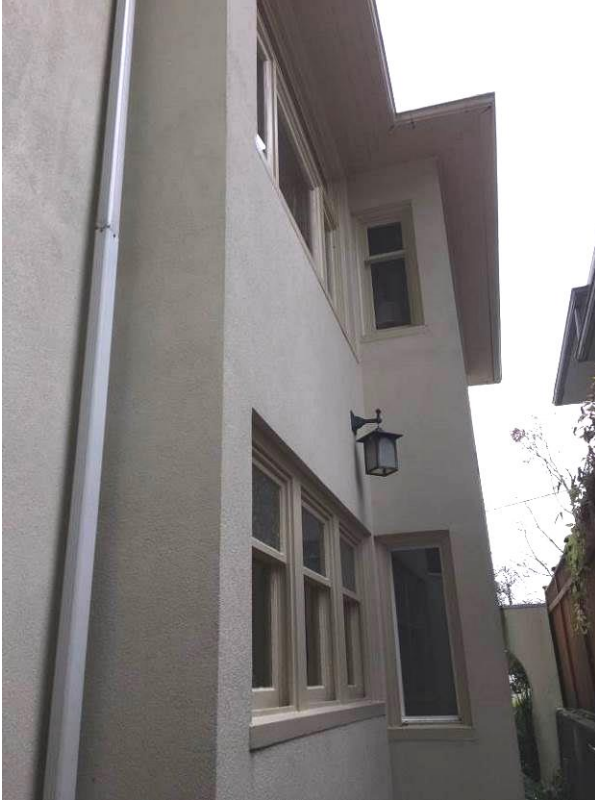
Photo #22 of 25 (WA_King County_Hannah Lewis House_0022) South elevation, camera facing east
