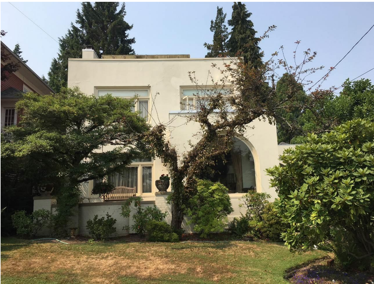
Photo #1 of 25 (WA_King County_Hannah Lewis House_0001) East façade, camera facing west
