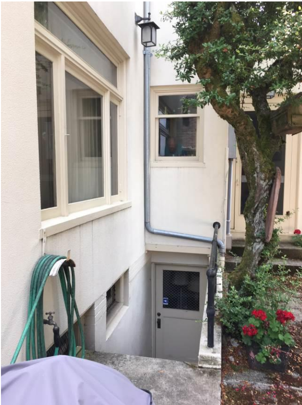
Photo #6 of 25 (WA_King County_Hannah Lewis House_0006) Detail of west façade (left) and stairwell to basement (center), camera facing south
