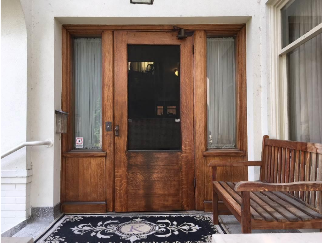
Photo #4 of 25 (WA_King County_Hannah Lewis House_0004) Primary entry, north elevation, camera facing south
