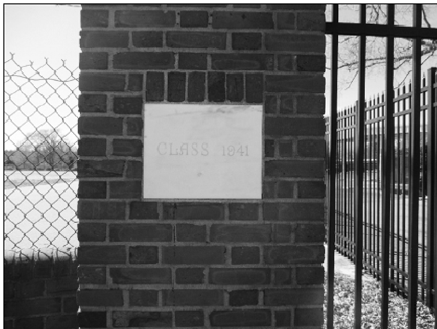
13. Brick Pier at Entrance to Former Oceana School Property
