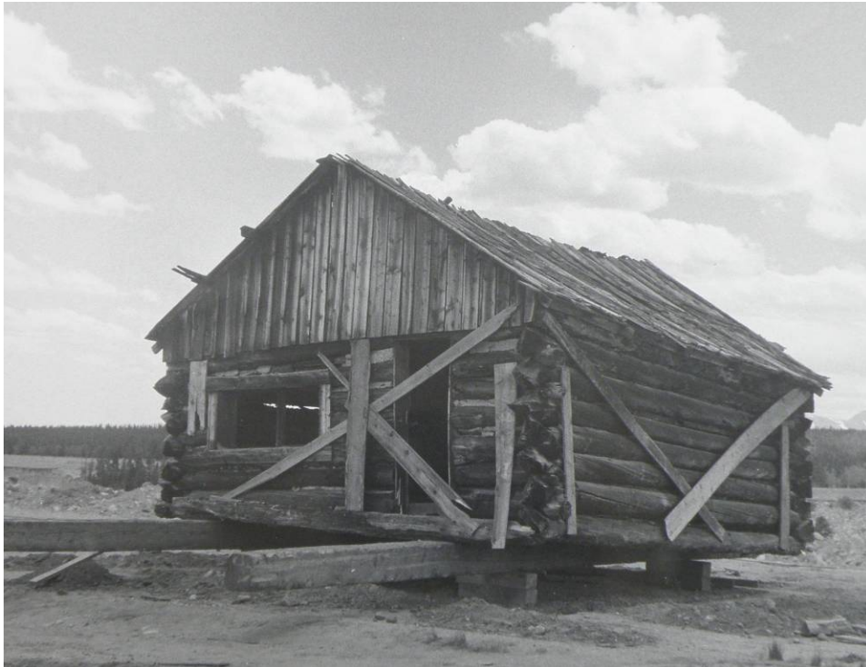
H3. Blacksmith Shop move in progress. c.1958.
