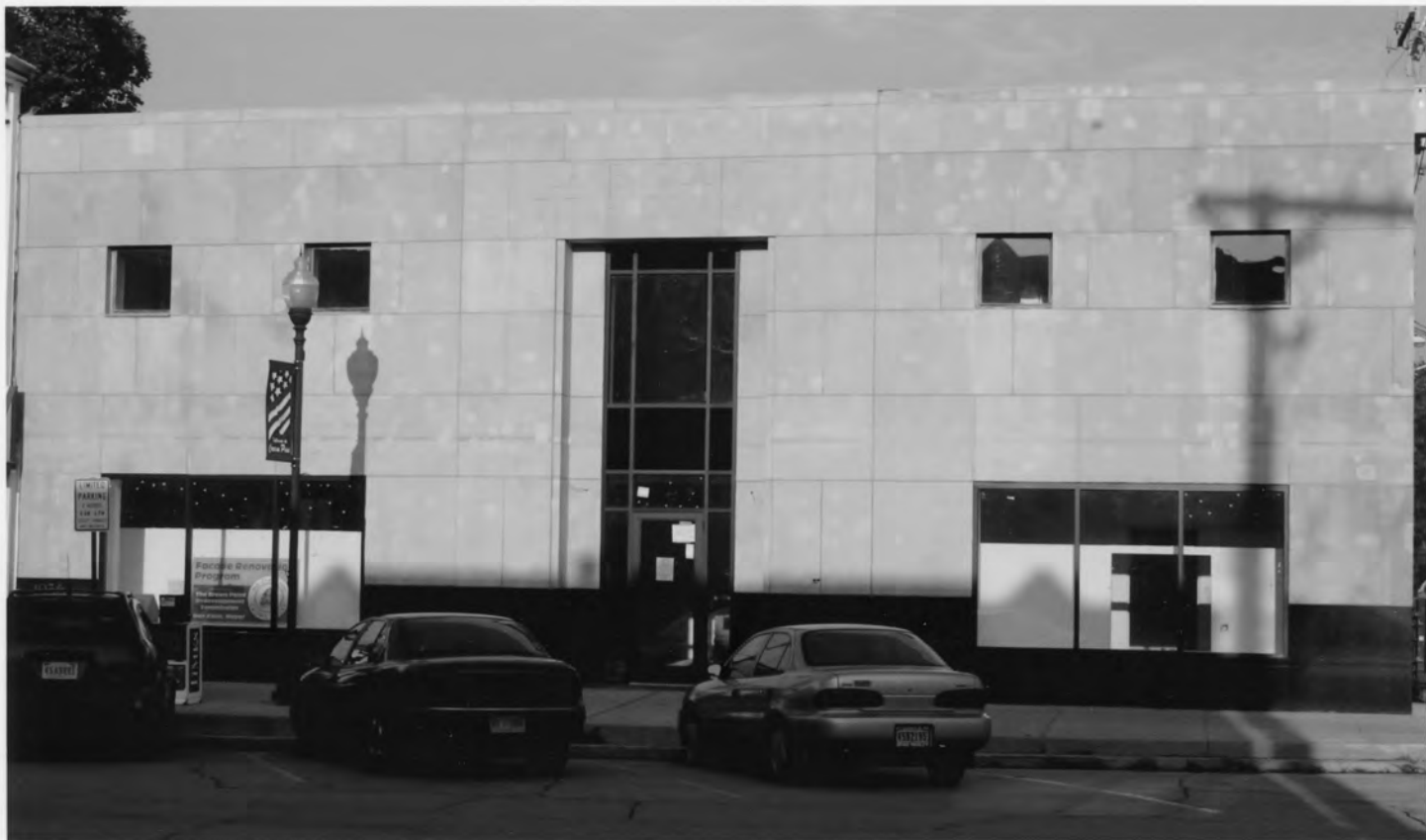
#1 Crown Point Courthouse Square Historic District Boundary Increase II (208 Main) Lake Co., IN
