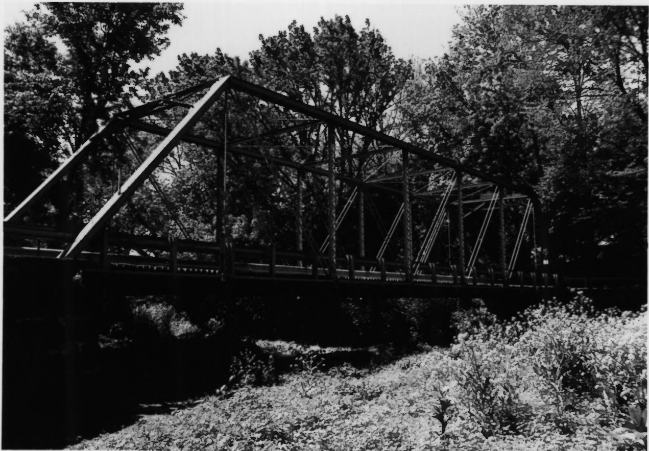
HIGGINSVILLE RD. BRIDGE, SOMERSET + HUNTERDON COUNTIES, HILLSBOROUGH-READINGTON, NT #B-1
