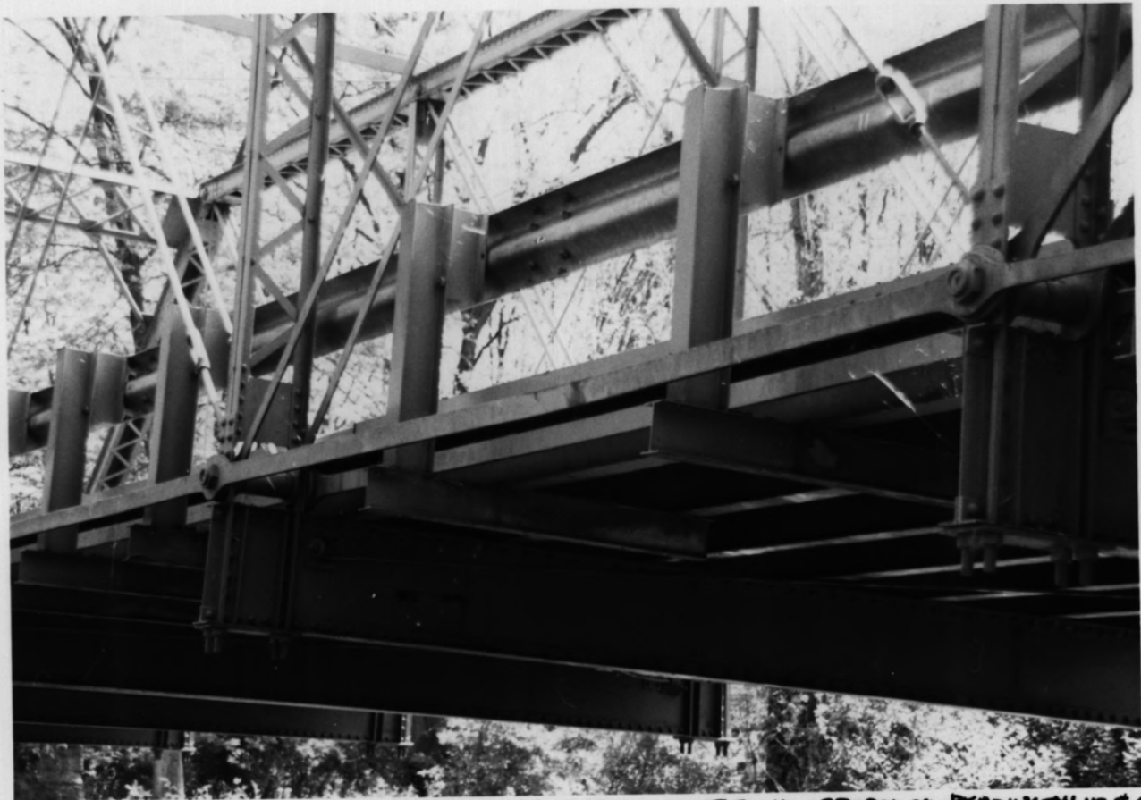
HIGGINSVILLE RD. BRIDGES, SOMERSET + HUNTERDON COUNTIES, HILLSBOROUGH-READINGTON, NJ #A-3
