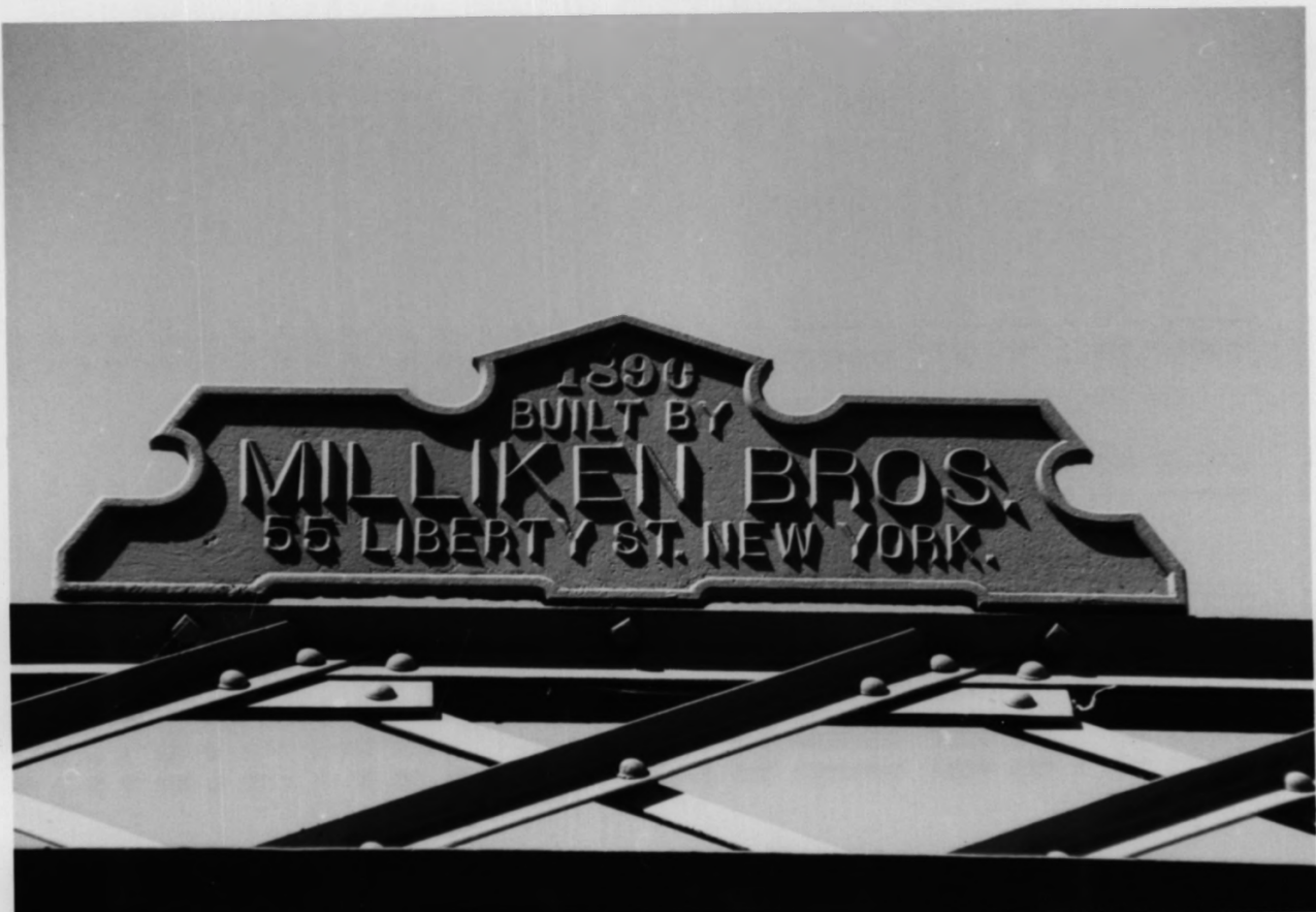
HCCINSVILLE RD. BRIDGES, SOMERSET + HUNTERDON COUNTIES, HILLSBOROUGH-READINGTON, NJ #A-6
