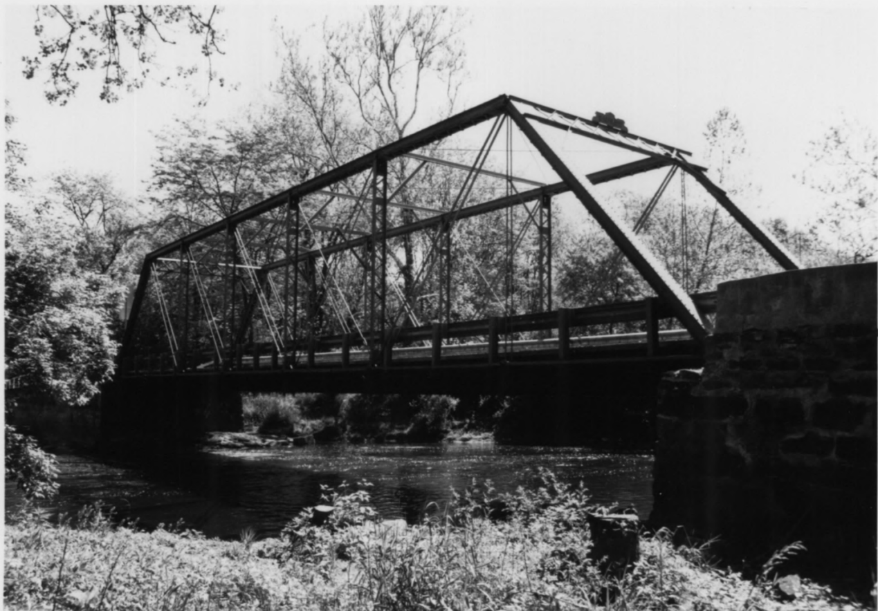
HIGGINSVILLE RD. BRIDGES, SOMERSET + HUNTERDON COUNTIES, HILLSBOROUGH-READINGTON TOWNS, N.J. # A-2
