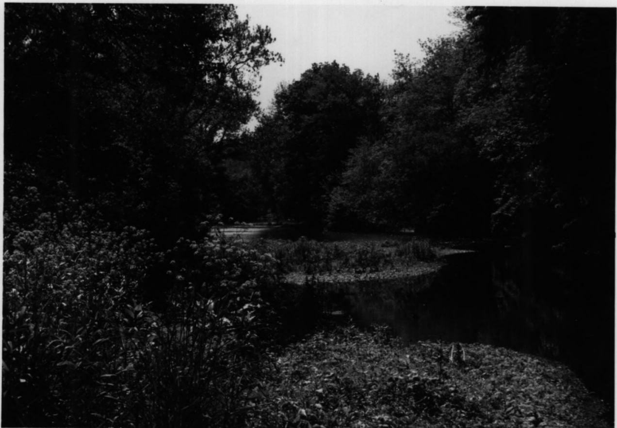
HIGGINSVILLE RD. BRIDGES, SOMERSET + HUNTERDON COUNTIES, HILLBOROUGH - READINGTON, NJ
