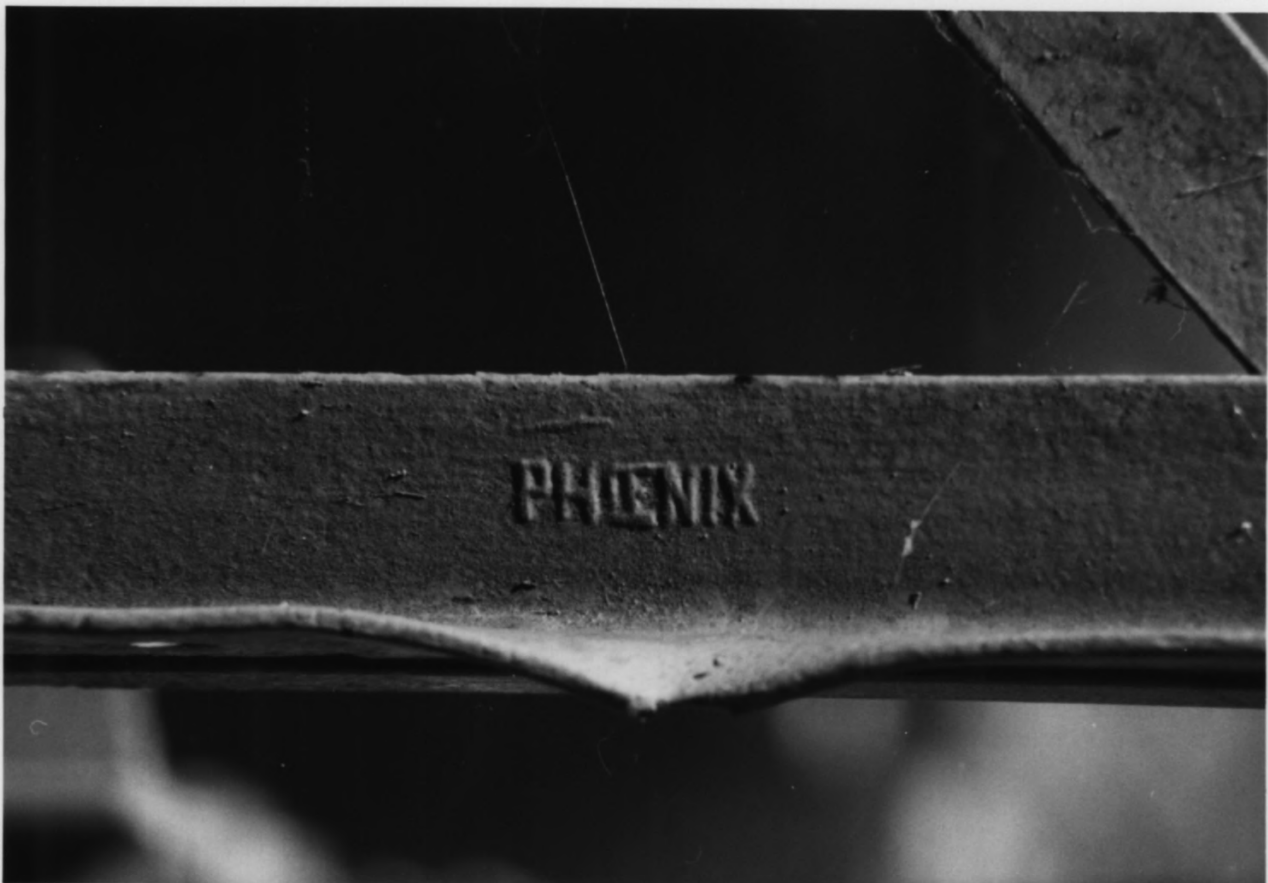
HIGGINSVILLE ED. BRIDGES, SOMERSET + HUNTERDON COUNTIES, HILLSBOROUGH - READINGTON, NJ # 8-7
