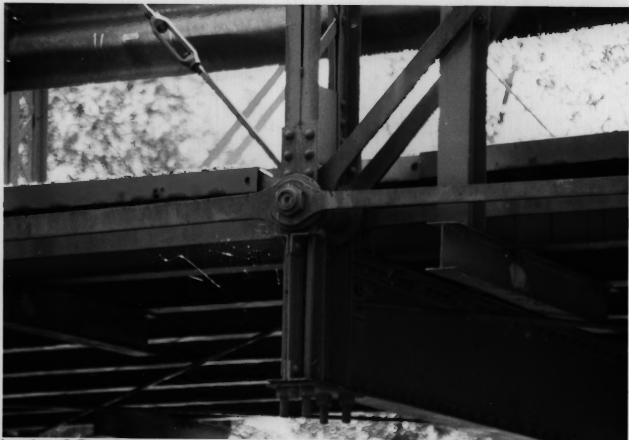
HIGGINSVILLE RD BRIDGES, SOMERSET+HUNTERDON COUNTIES, HILLSBOROUGH-READINGTON, NJ 4A-4
