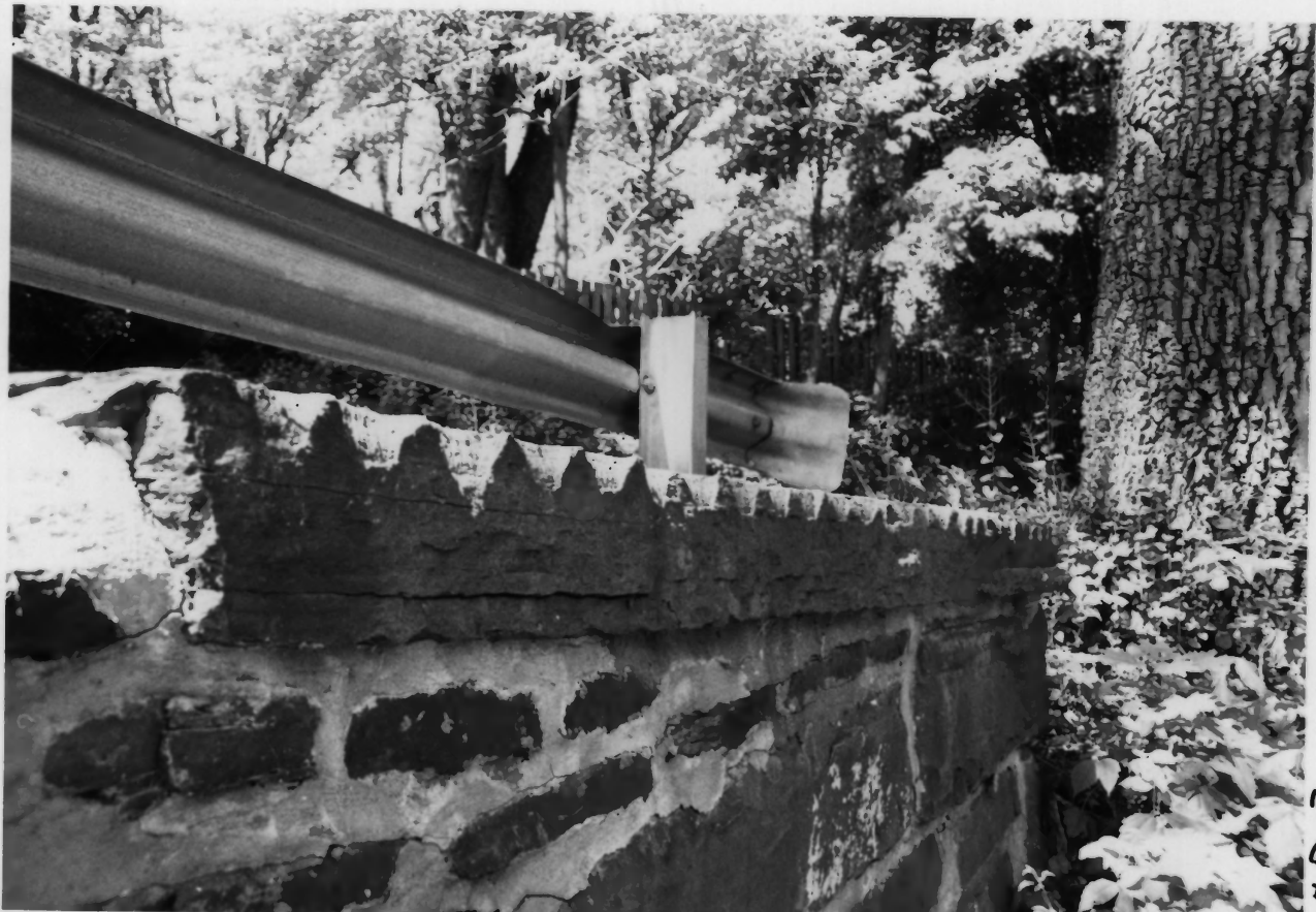
HIGGINSVILLE RD. BRIDGES, SOMERSET + HUNTERDON COUNTIES, HILLSBOROUGH - READINGTON, NJ
