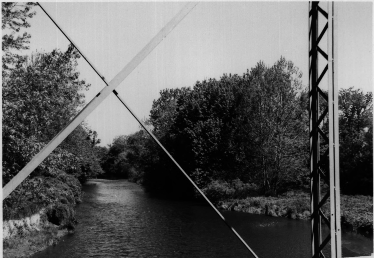
HIGGINSVILLE RD. BRIDGE, SOMERSET + HUNTERDON CTYS., HILLSBOROUGH - READINGTON, NJ # 3
