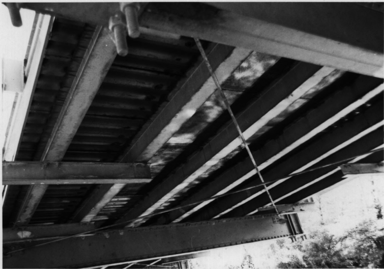
HIGGINSVILLE BRIDGES, SOMERSET + HUNTERDON COUNTIES, HILLSBOROUGH + READINGTON, NJ #A-10
