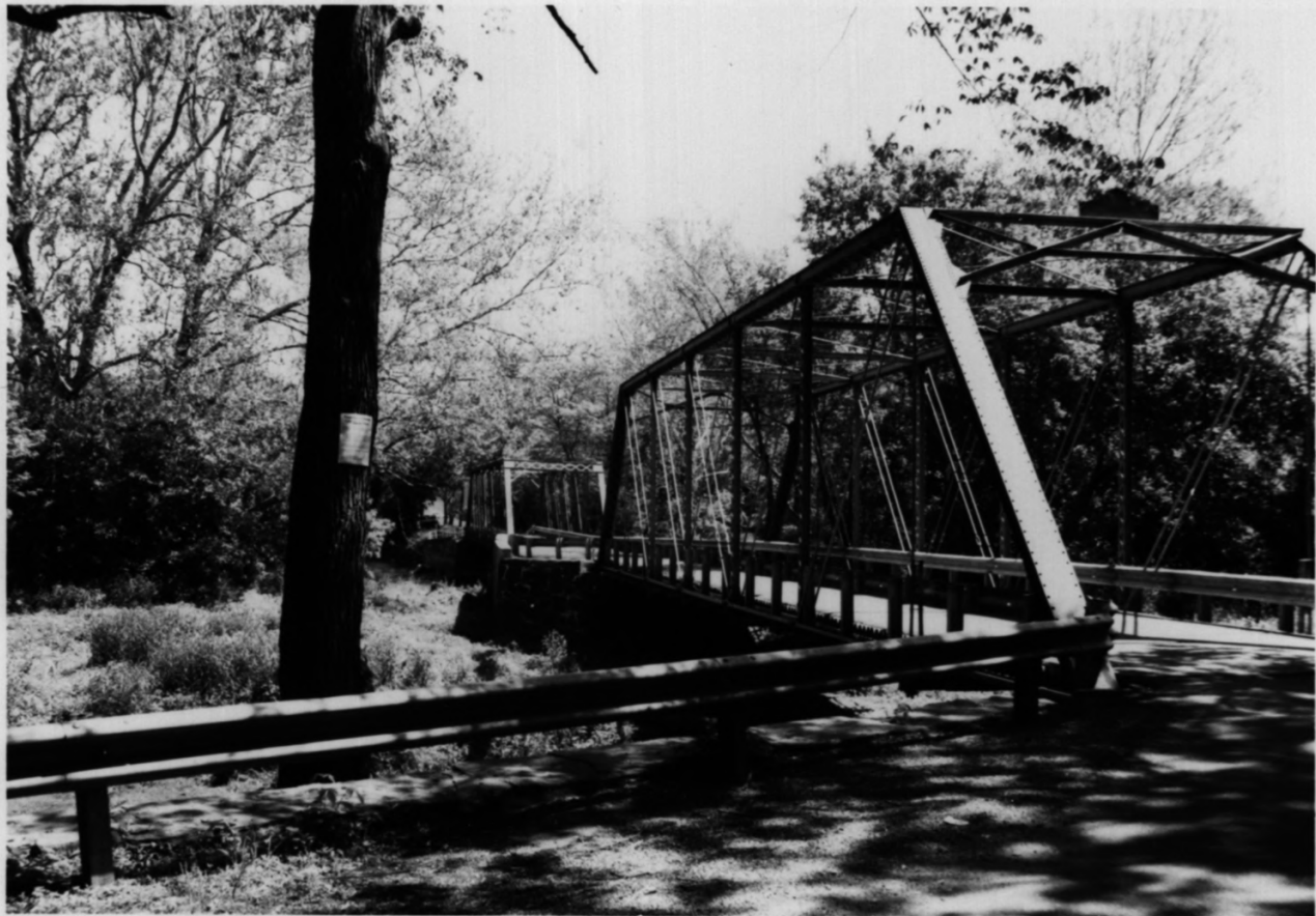
HIGGINSVILLE RD. BRIDGES, SOMERSET + HUNTERDON CV. HILLSBOROUGH-READINGTON TOWNS., NJ
