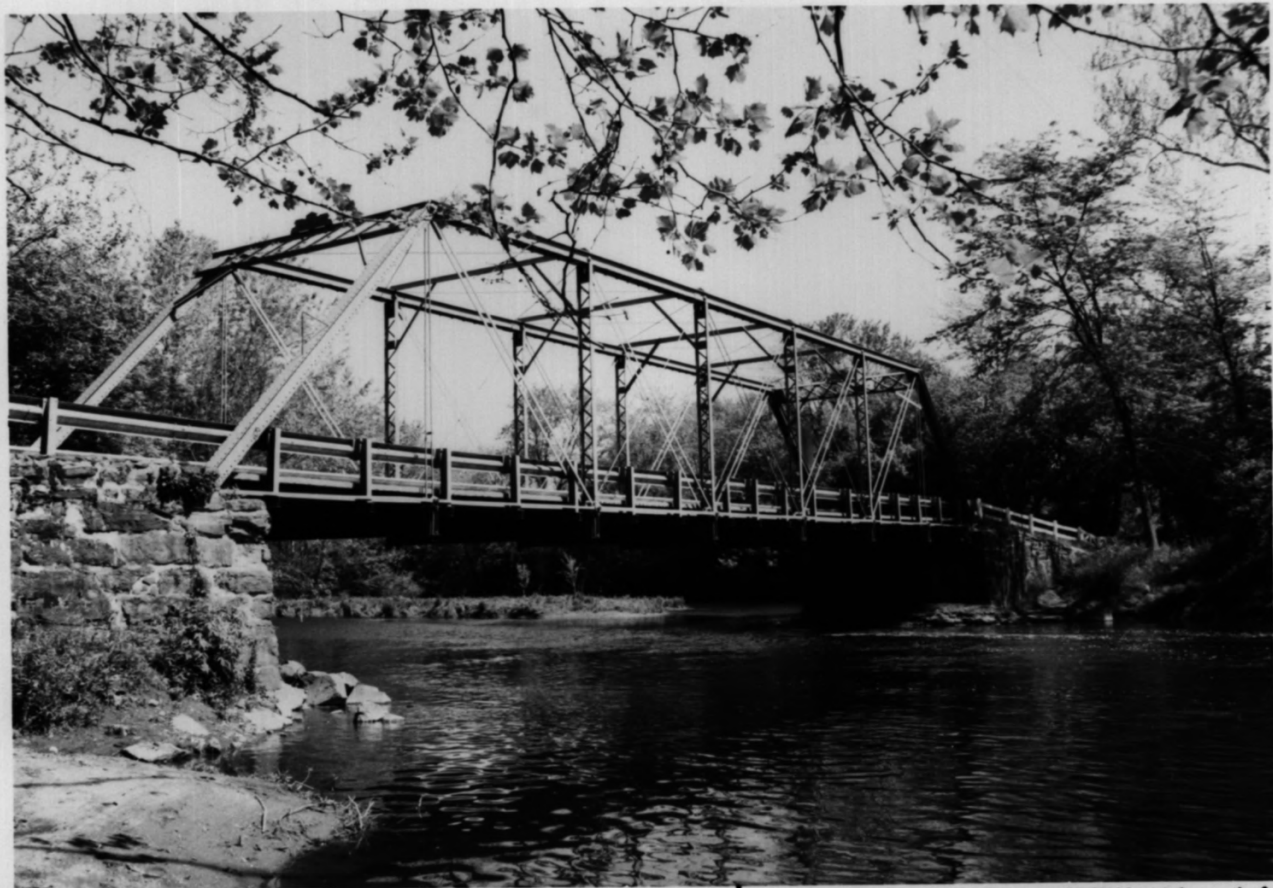
HIGGINSVILLE RD. BRIDGES, SOMERSET + HUNTERDON COUNTIES, HILLSBOROUGH - READINGTON, NJ # A-1
