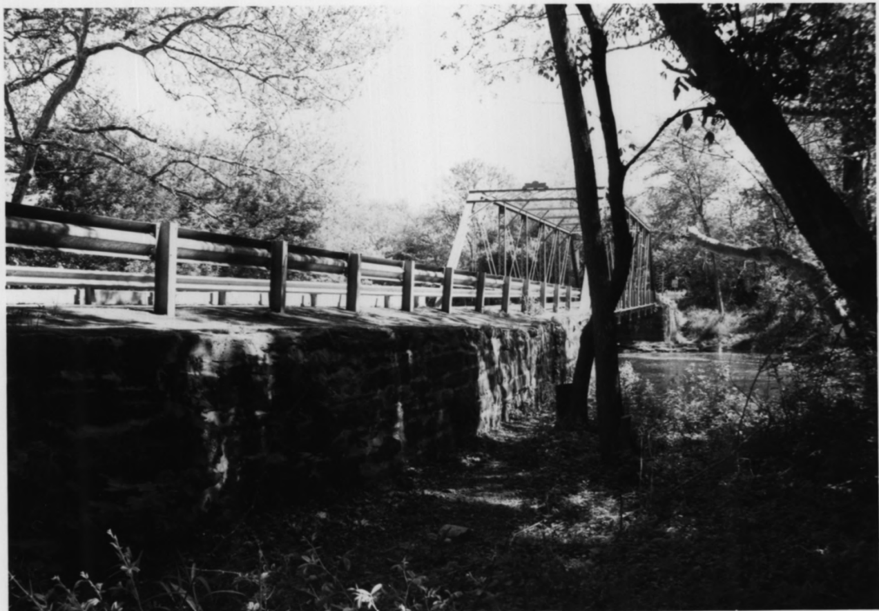
HIGGINSVILLE RD. BRIDGES, SOMERSET + HUNTERDON COUNTIES, HILLSBOROUGH-READINGTON NJ #A-12
