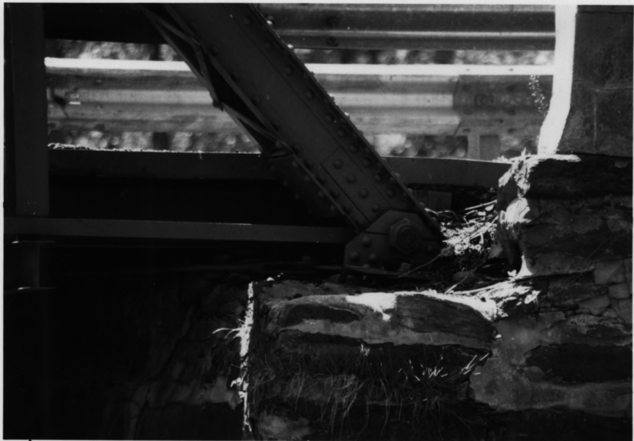
HIGGINSVILLE RD. BRIDGES, SOMERSET + HUNTERDON COUNTIES, HILLSBOROUGH - READINGTON, NJ #A-5
