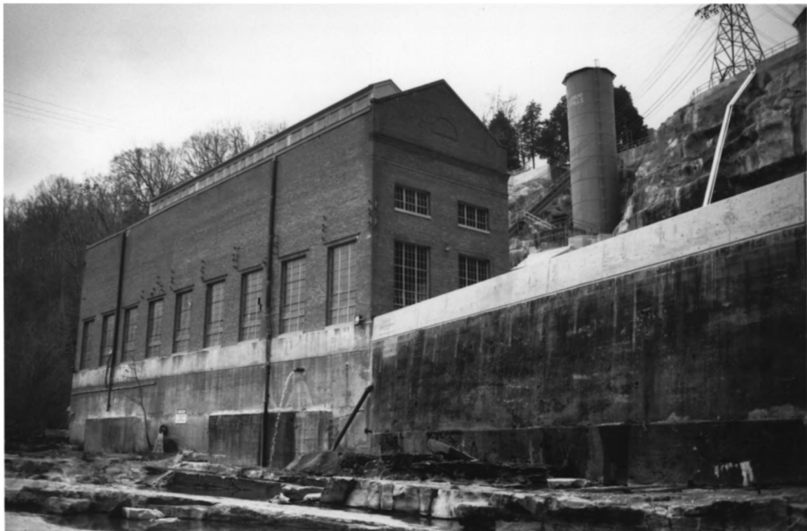
Great Falls Hydroelectric Station Rock Island vicinity, White & Narren Co's, TN
