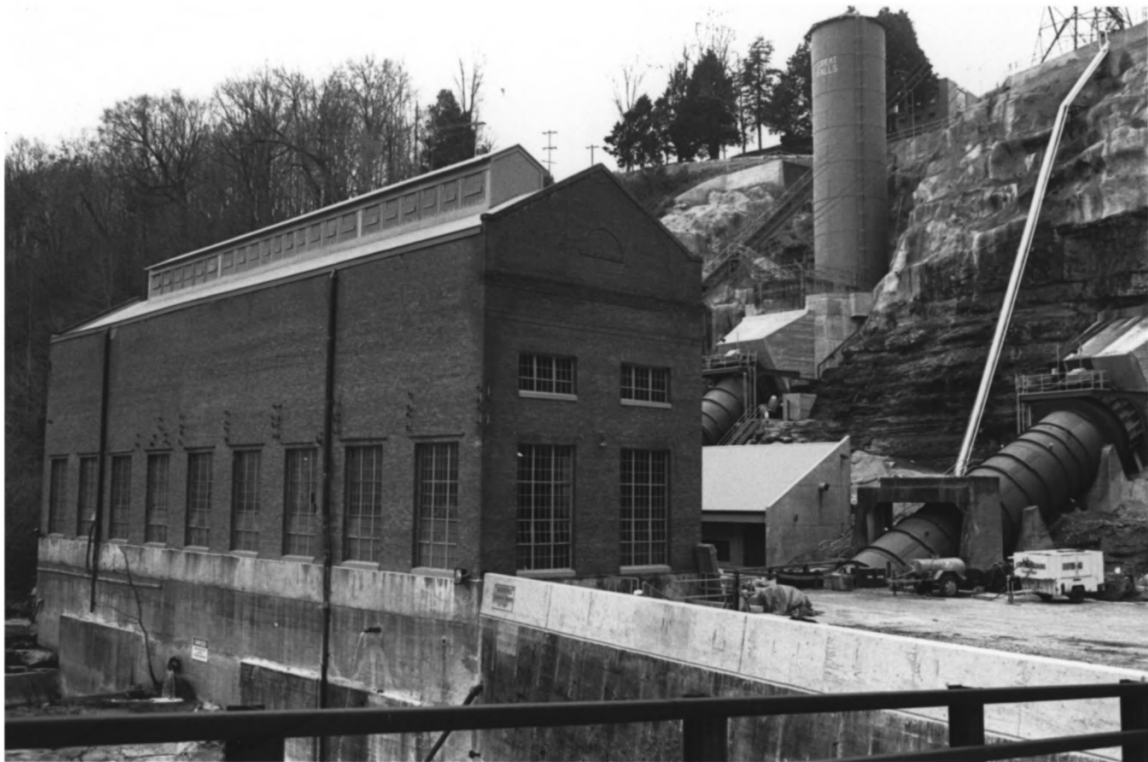
Great Falls Hydroelectric Station Rock Island vicinity, White & Warren Co's, TN
