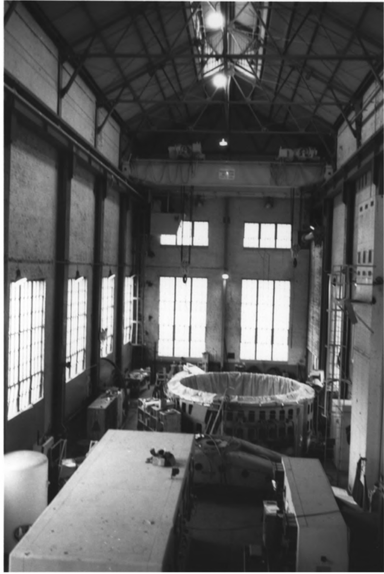
Great Falls Hydroelectric Station Rock Island vicinity, White & Warren Cos., TN
