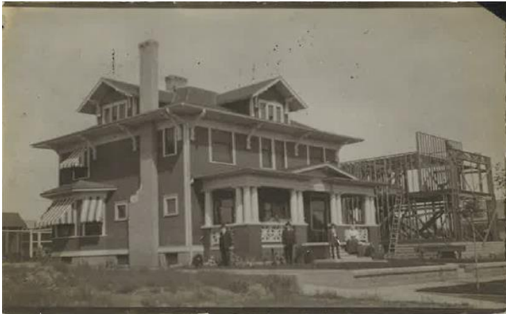
Southeast side of home (1909) (Robinson and Smith standing out front) Historic photo 1 of 12
