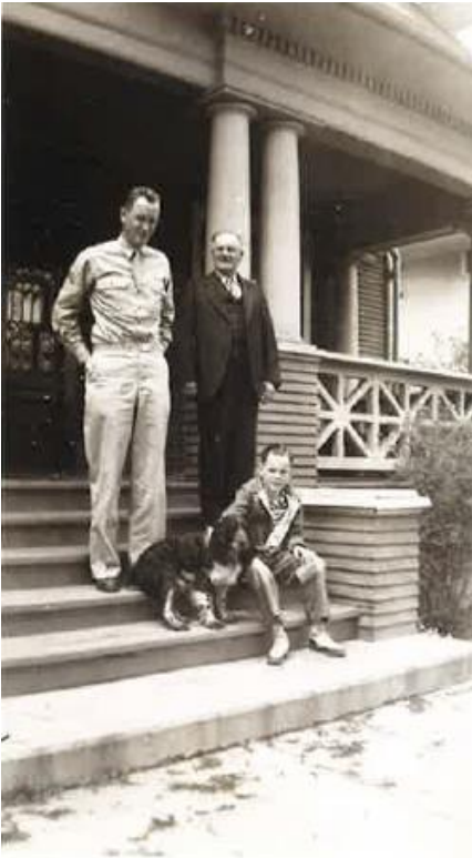
Stairs to front porch (1945) (from left to right Carl Ralston, Walter McNeil, Atley Ralston) Historic photo 6 of 12
