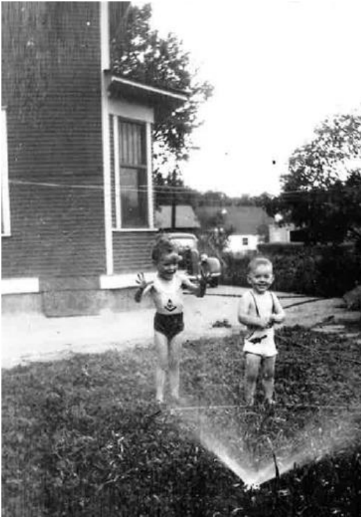
East side of house (1937) (Atley Ralston on left) Historic photo 10 of 12
