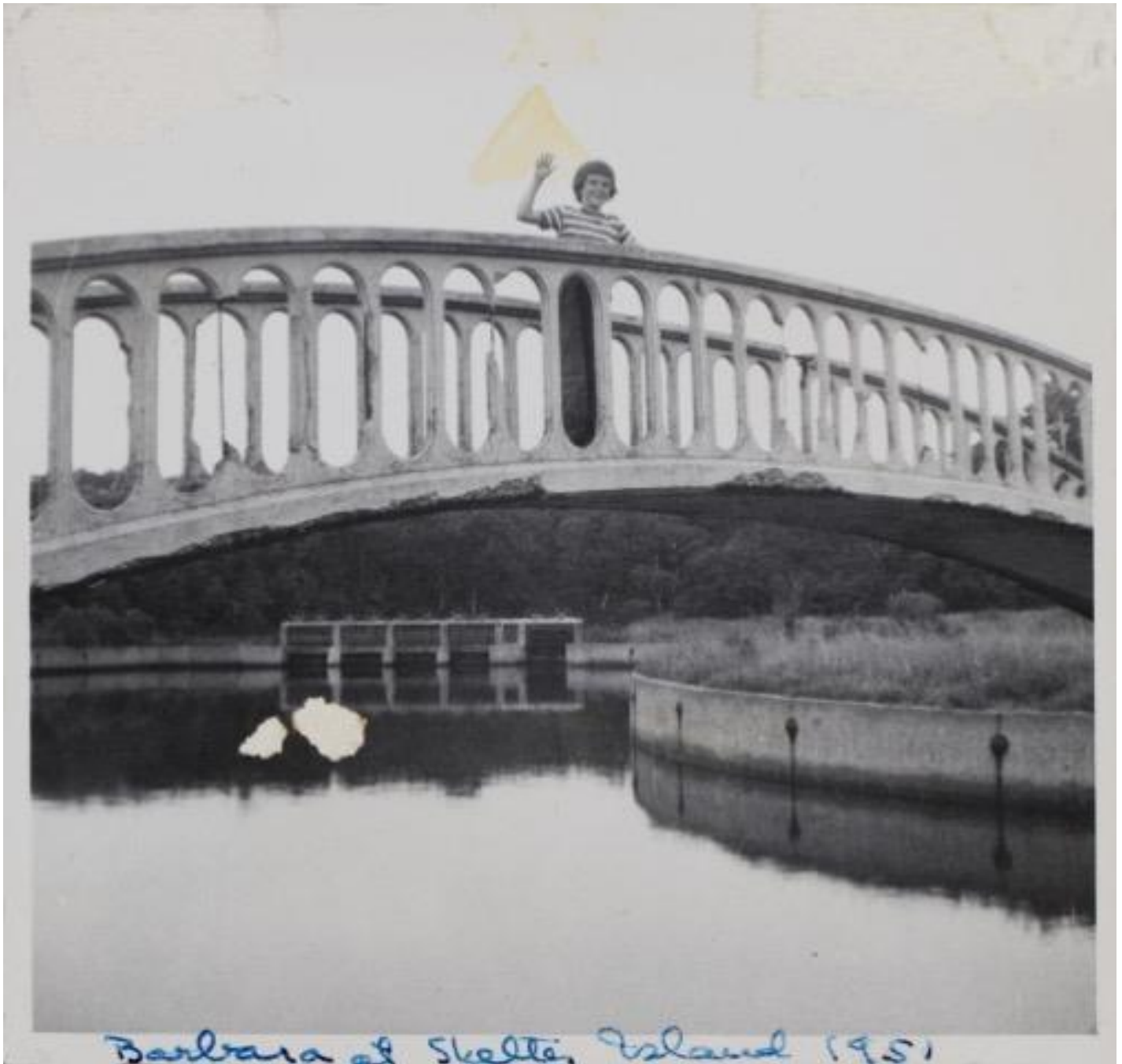
Figure 4. Bridge and Lagoon, 1951.
