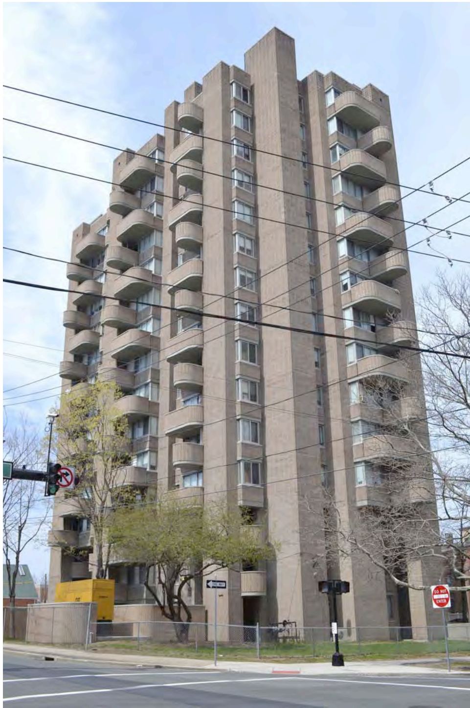
East (side) and south (rear) elevations of Crawford Manor from North Frontage Road, 1964-1966. Camera facing northwest. Photograph 1 of 19.
