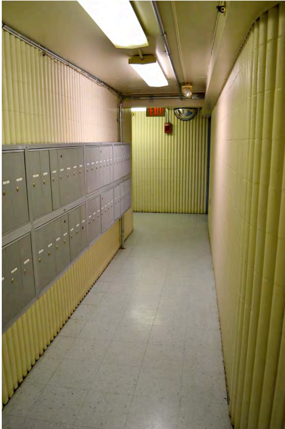
Detail of first-floor corridor, showing mailboxes, floor, wall, and ceiling details. Camera facing southeast. Photograph 8 of 19.
