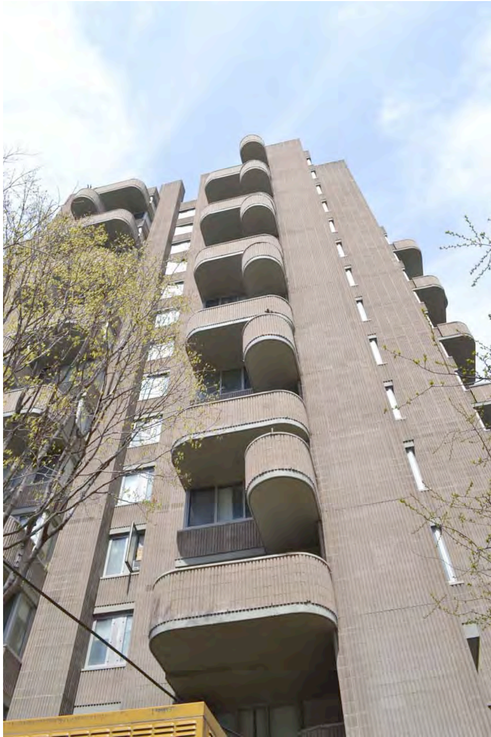
South (rear) elevation of Crawford Manor from North Frontage Road, 1964-1966, showing wall, balcony, and window details.
