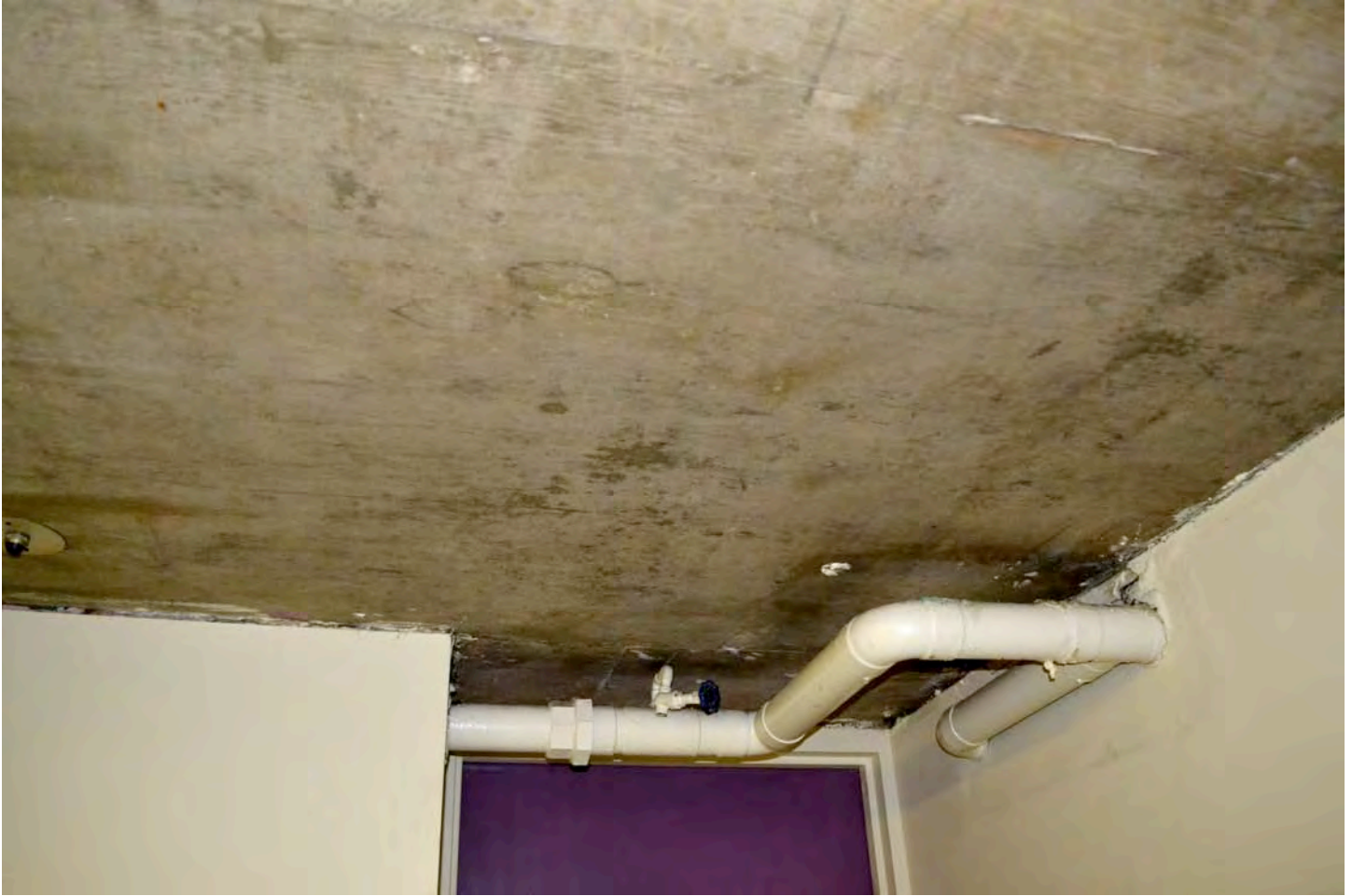
Detail of typical upper-floor ceiling. Camera facing southeast. Photograph 18 of 19.
