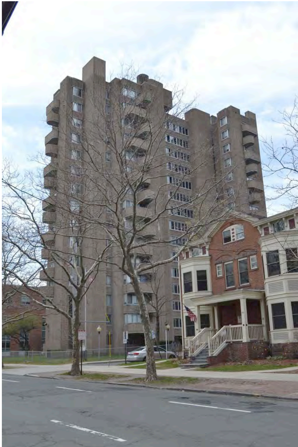
North (front) and east (side) elevations of Crawford Manor from Park Street, 1964-1966. Camera facing southwest. Photograph 2 of 19.
