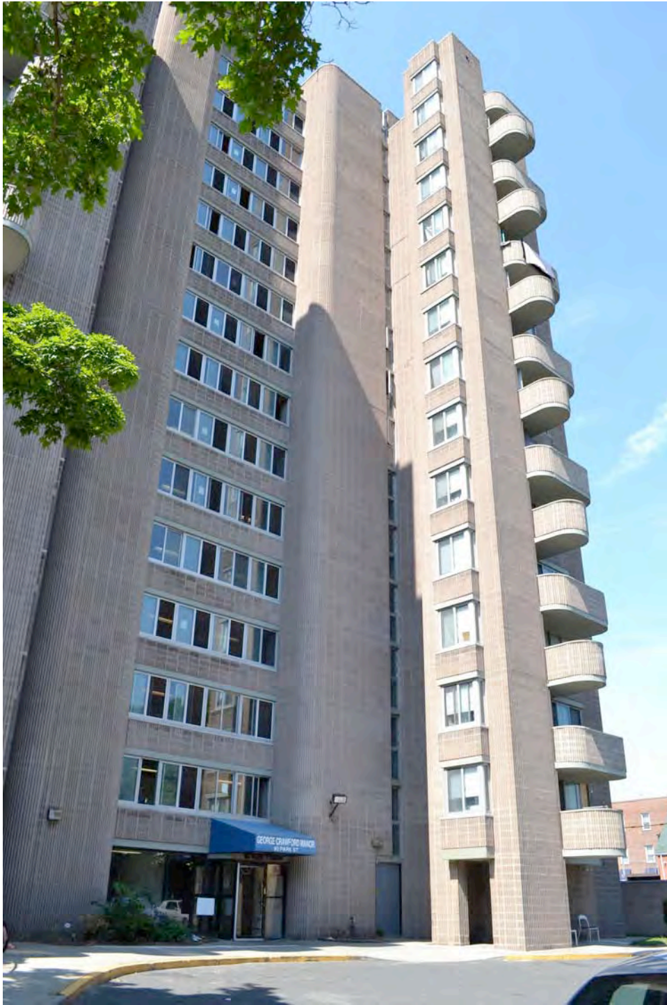
North (front) elevation of Crawford Manor from Park Street, 1964-1966. Camera facing southwest. Photograph 3 of 19.
