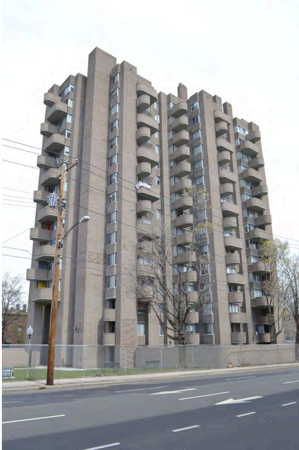
West (side) and south (rear) elevations of Crawford Manor from North Frontage Road, 1964-1966. Camera facing northeast. Photograph 5 of 19.
