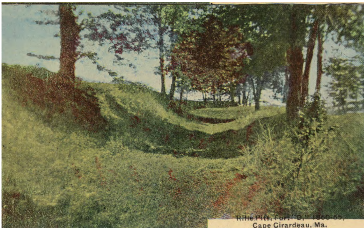
Figure 17. Postcard showing Fort D “rifle pits” ca. 1936 (probably south walls looking east) before renovation. Note incorrect state abbreviation.
