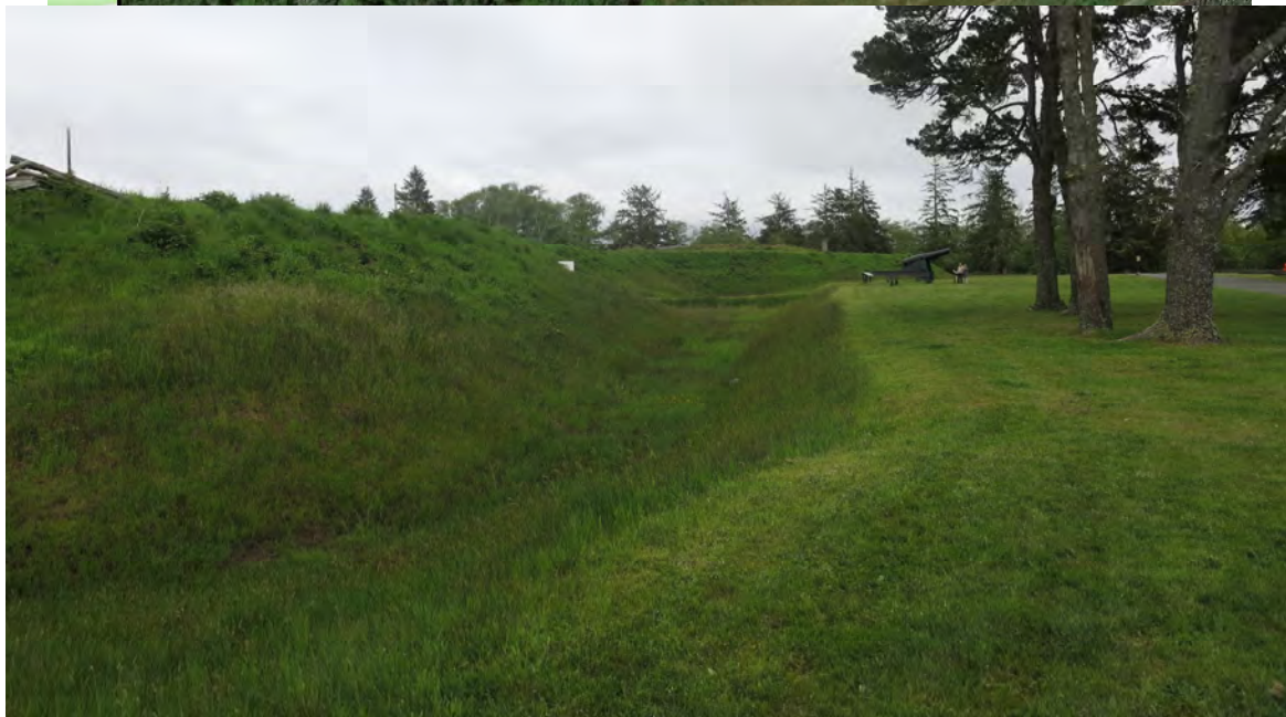
Figure 31. Redan walls at Fort Stevens, Oregon. SOURCE: Google Maps, 2018 & Photo by Scott House
