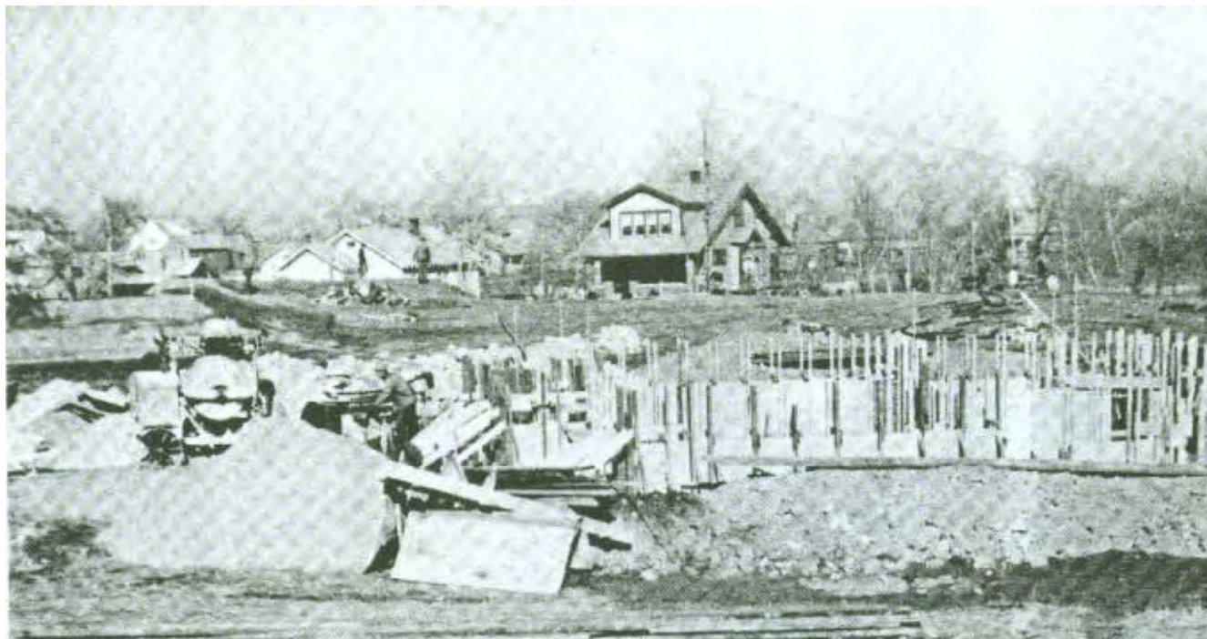
Figure 19. Construction underway on the blockhouse/museum structure looking west. SOURCE: Courtesy of Southeast Missourian.
