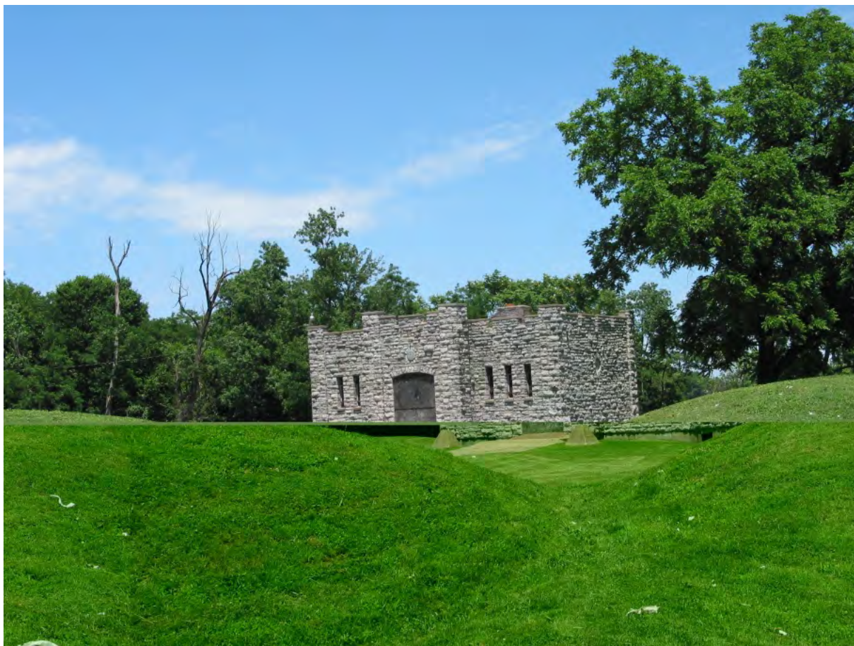
Figure 25: Looking northeast at south wall and blockhouse, prior to most recent renovation and interpretive works. 2004.
