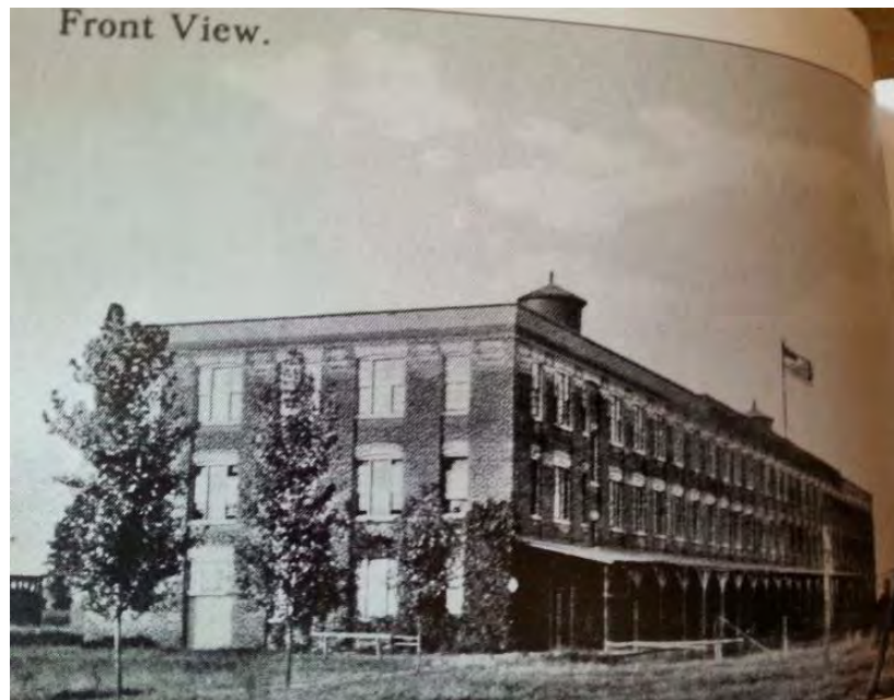
Figure 17. The Hickman-Ebbert Wagon Company building, demolished in 2010. 62
