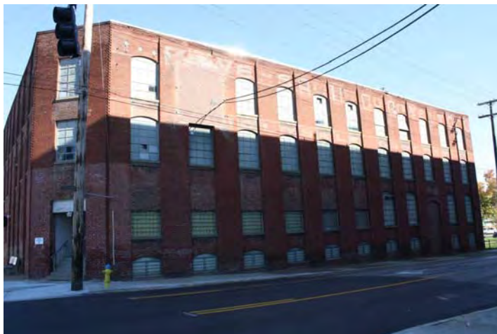
Figure 6. Façade (south elevation) of the KBC building, along East 9 th Street. (KY_DaviessCounty_KentuckyBuggyCompany_005)
