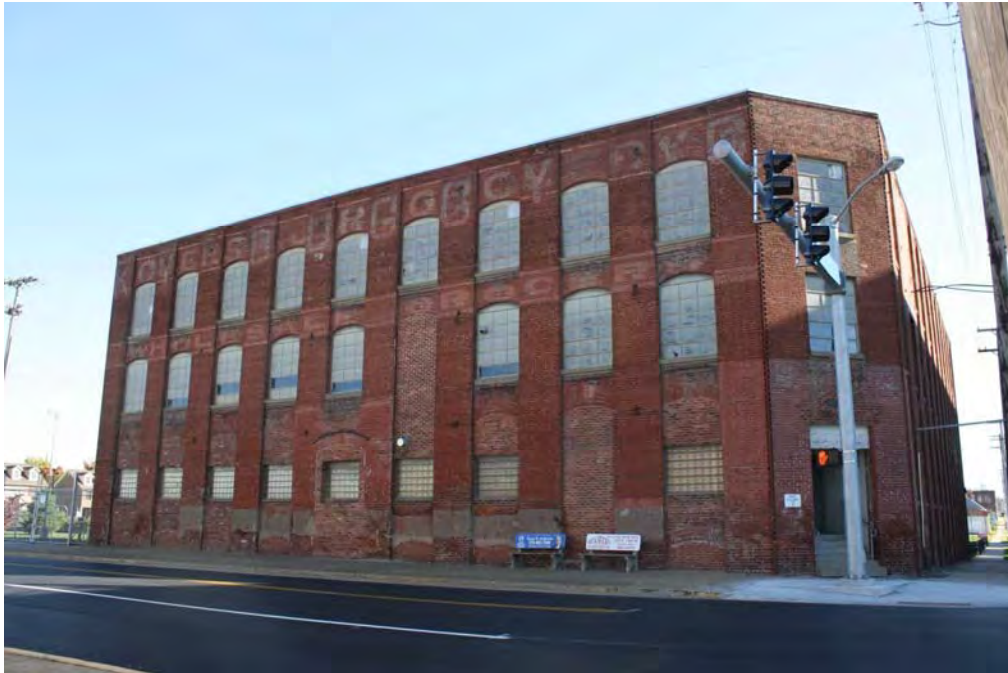
Figure 10. West elevation, which faces JR Miller Blvd. (KY_DaviessCounty_KentuckyBuggyCompany_003)
