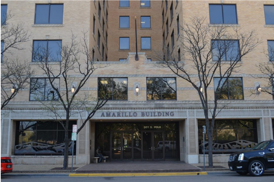
Photo 0005 – Detail of S. Polk entrance, view east.
