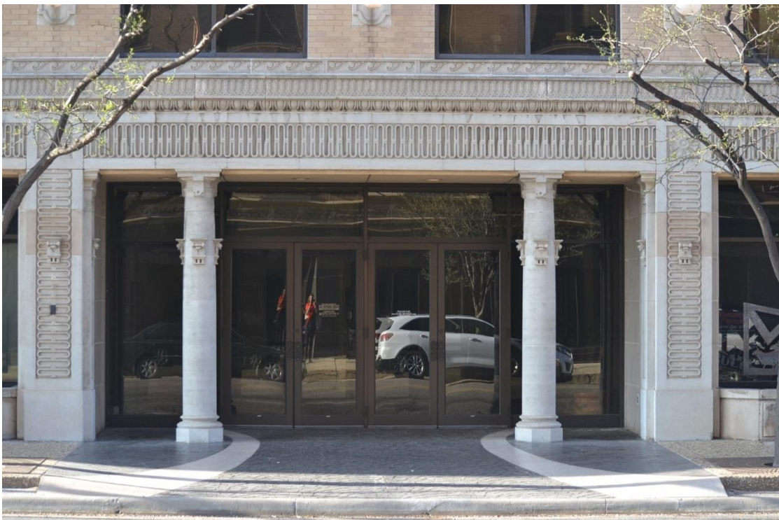
Photo 0006 – Detail of 3 rd Avenue entrance, view south
