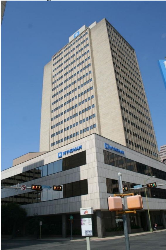
Photo 29 430 Soledad, National Bank of Commerce Building Camera facing NE
