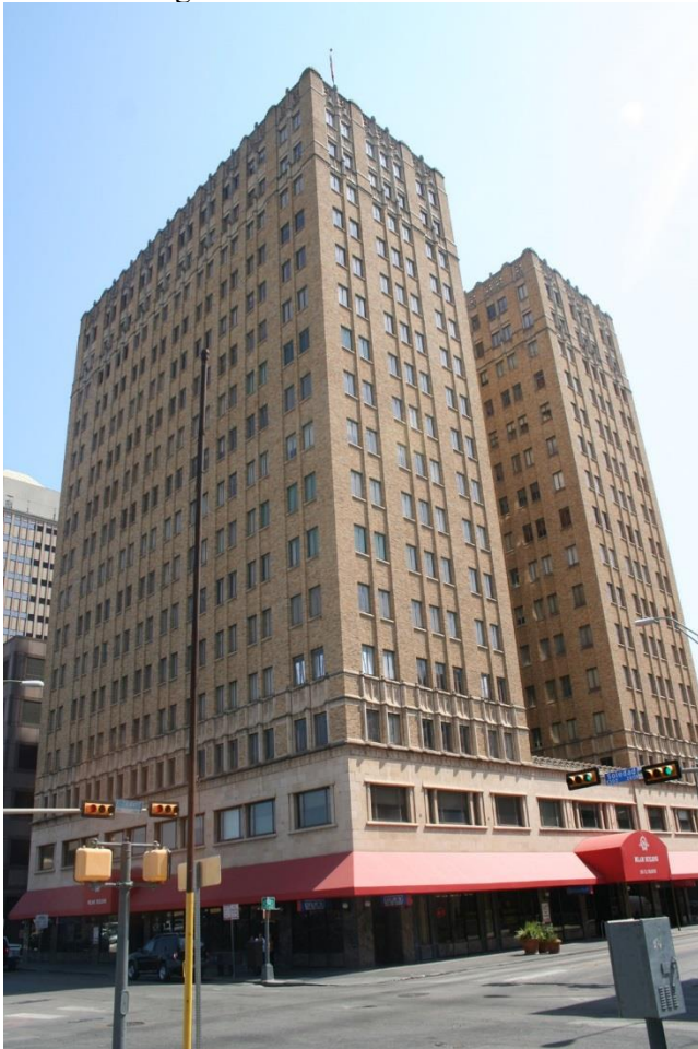
Photo 25 115 E Travis, Milam Building Camera facing NE
