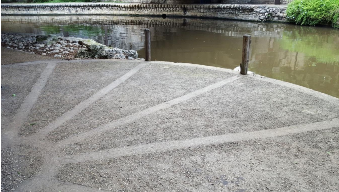
Photo 39 Block 4 (N St Mary's Street Bridge S26 to Augusta Street Bridge S07) Wagon wheel landing Camera facing W
