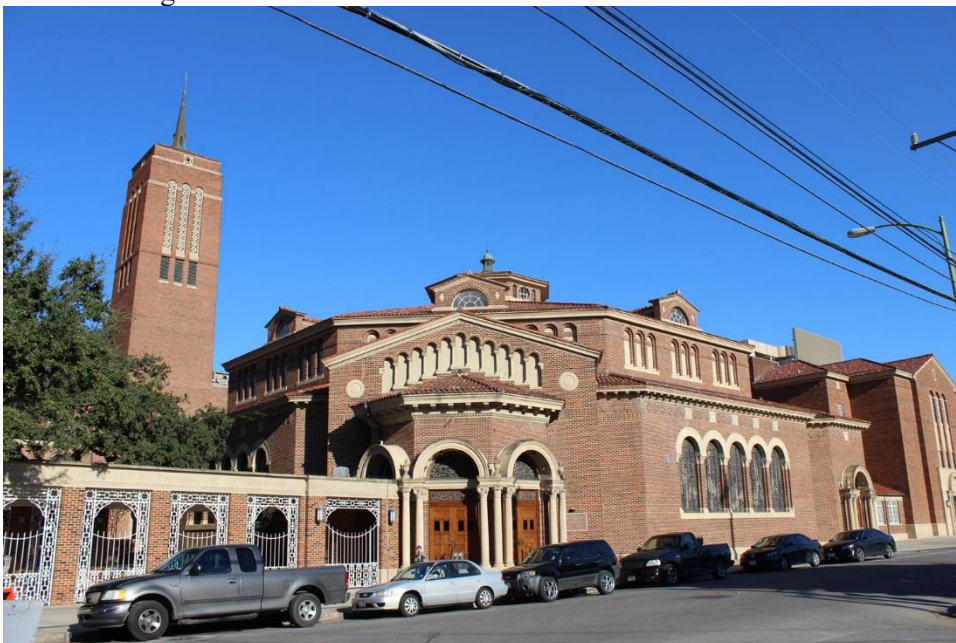
Photo 16 515 McCullough, First Baptist Church, Auditorium Camera facing E
