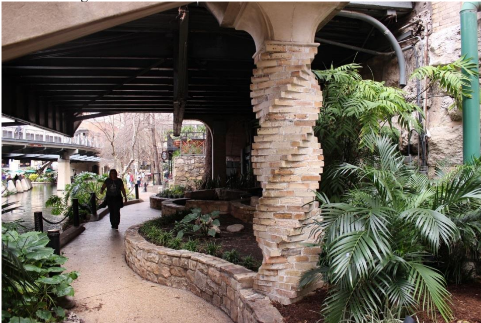
Photo 52 Block 15 (Crockett E Bridge S11 to Commerce Street Bridge / Jones Bridge S08) Twisted stair column Camera facing N
