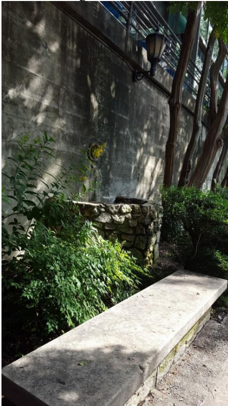
Photo 35 Block 2 (Richmond Ave Bridge S23 to Romana Street Bridge S24), Bench, drainage well, and crepe myrtles Camera facing SW
