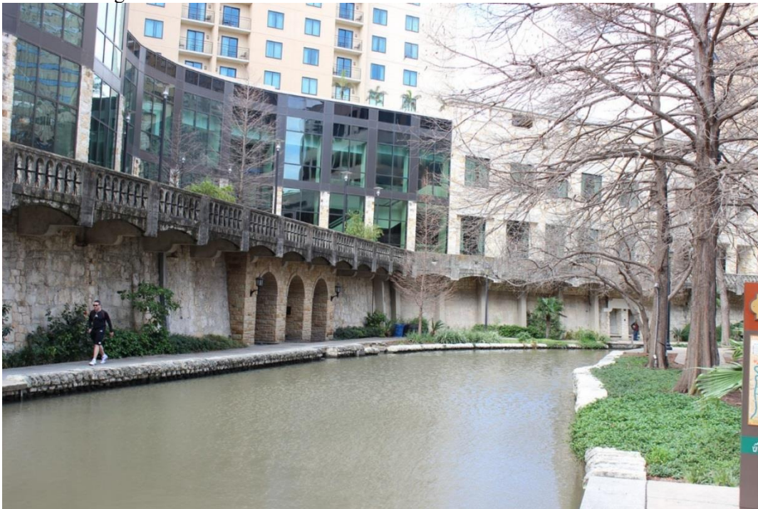
Photo 42 Block 9 (Travis Street Bridge S28 to Houston Bridge S12) Cantilevered walkway Camera facing NW
