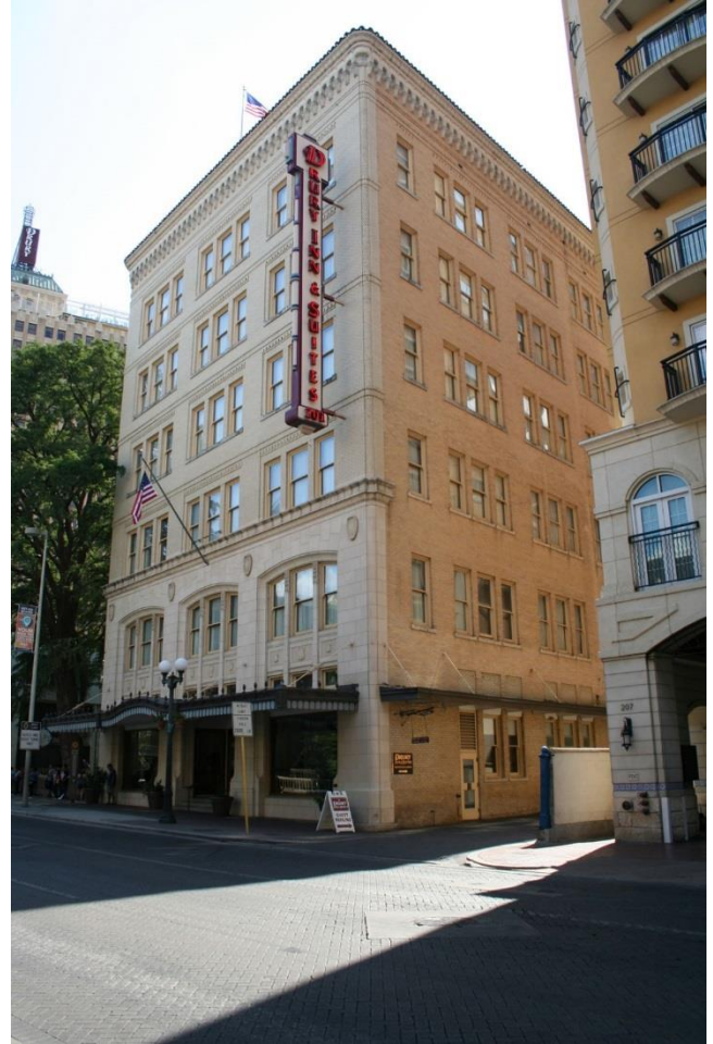
Photo 22 201 N St. Mary's, City Public Service Building Camera facing SW
