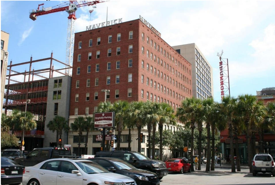
Photo 77 George Maverick Building Camera facing SE
