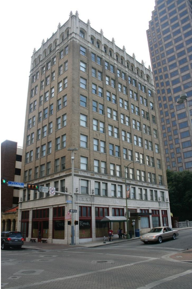
Photo 21 152 E Pecan, Builder's Exchange Building Camera facing SW
