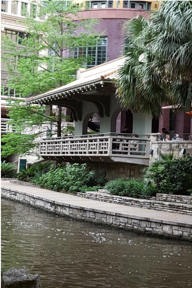
Photo 43 Block 10 (Houston Bridge S12 to Upper Flood Gate) Balcony Camera facing NE
