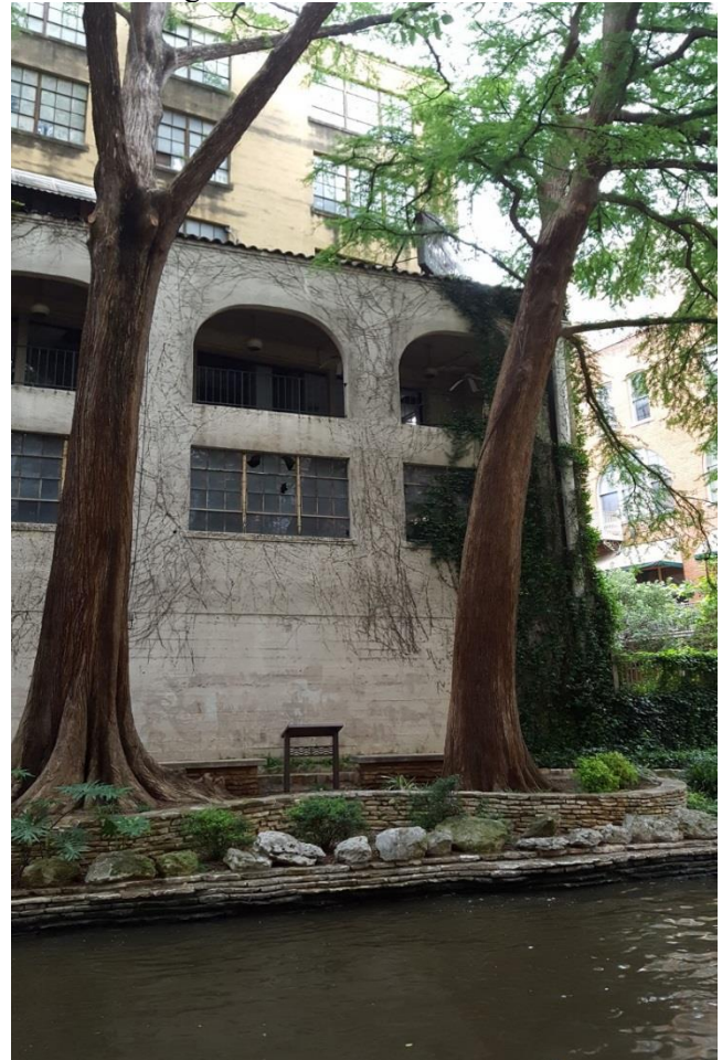
Photo 44 Block 10 (Houston Bridge S12 to Upper Flood Gate) Cypress trees Camera facing W
