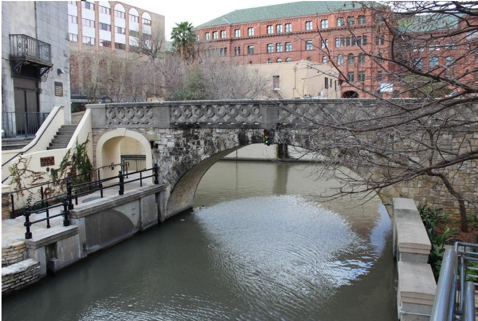
Photo 63 Block 20 (St. Mary's S Street Bridge S27 to Lower Floodgate) Floodgate Camera facing SW
