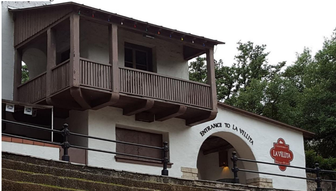
Photo 59 Arneson Theater Concession building Camera facing SW
