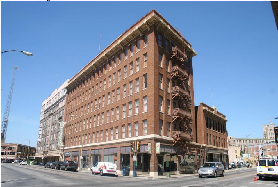
Photo 14 214 Broadway, Calcasieu Building Camera facing NE
