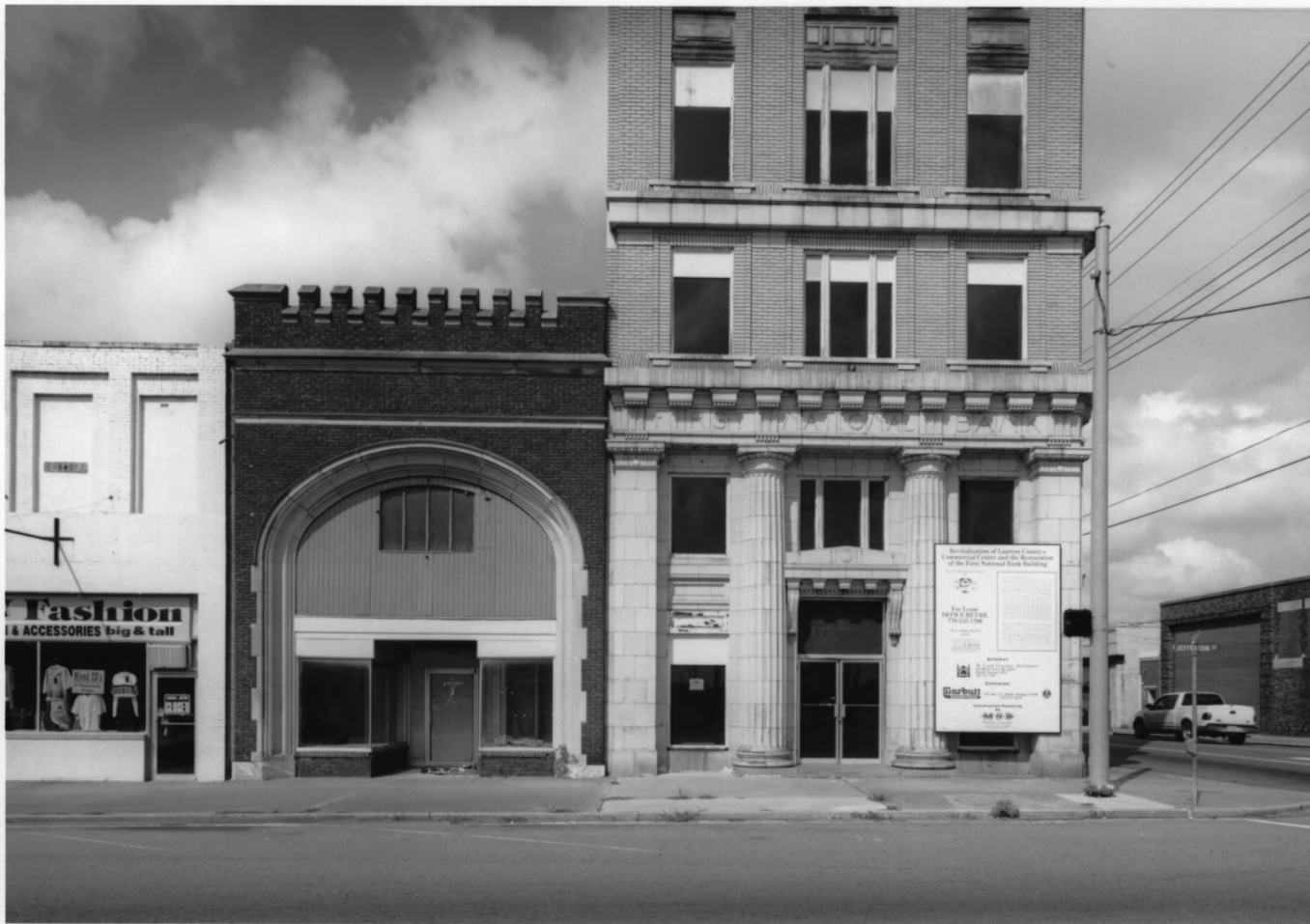
DUBLIN COMMERCIAL HISTORIC DISTRICT DUBLIN, LAURENS COUNTY, GEORGIA PHOTOGRAPH 14 OF 28
