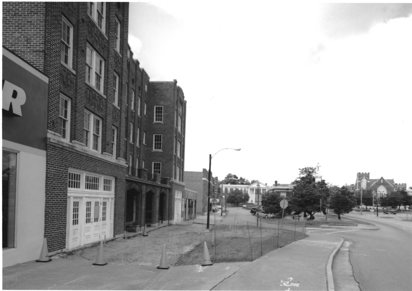
DUBLIN COMMERCIAL HISTORIC DISTRICT DUBLIN, LAURENS COUNTY, GEORGIA PHOTOGRAPH 26 OF 28
