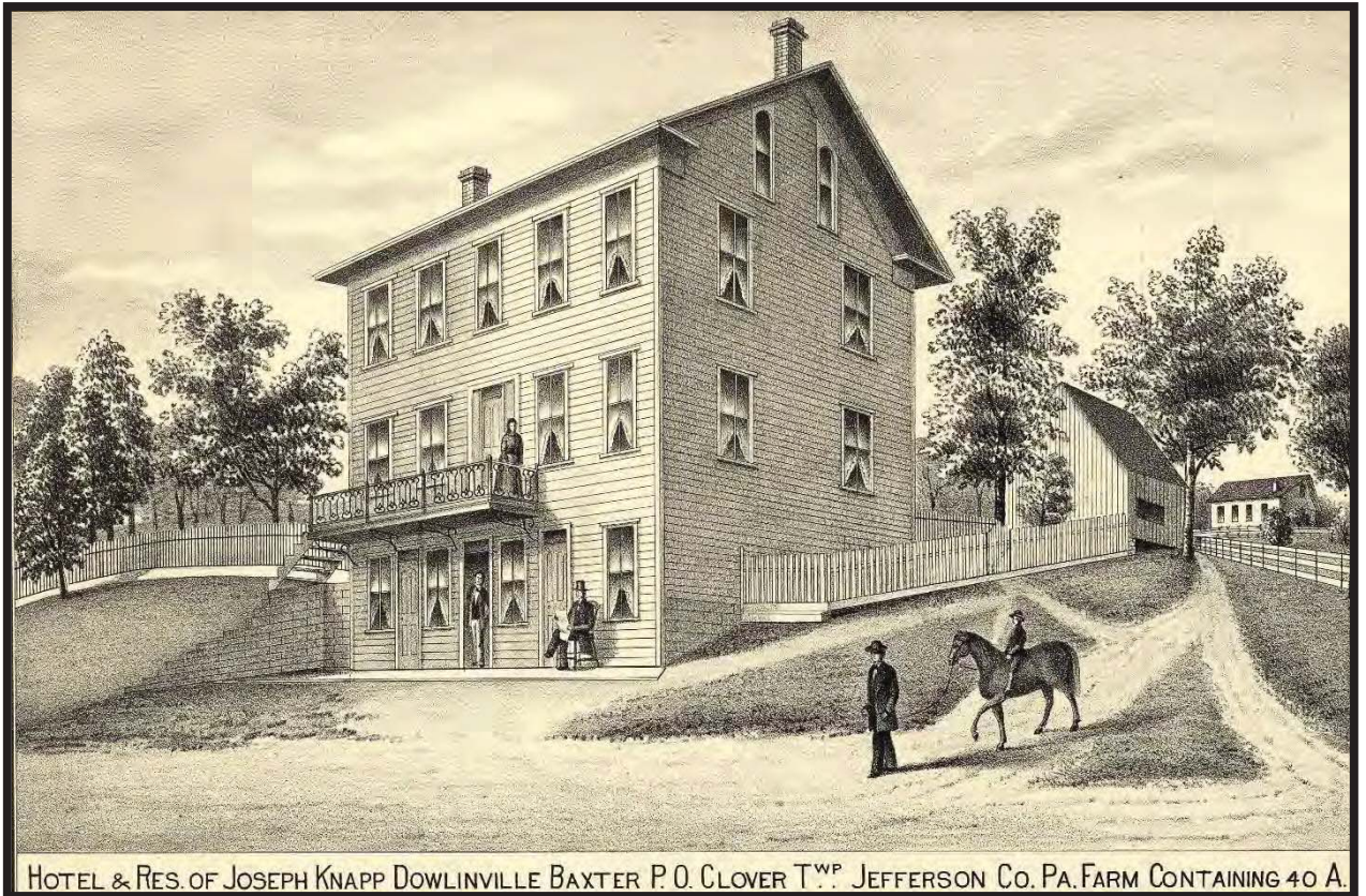
Figure 1: Sketch of Joseph Knapp Hotel from Caldwell's Atlas of Jefferson County Pennsylvania (1878:68) showing south façade and east elevation. Note the original wood and iron balcony on the façade at the second floor.
