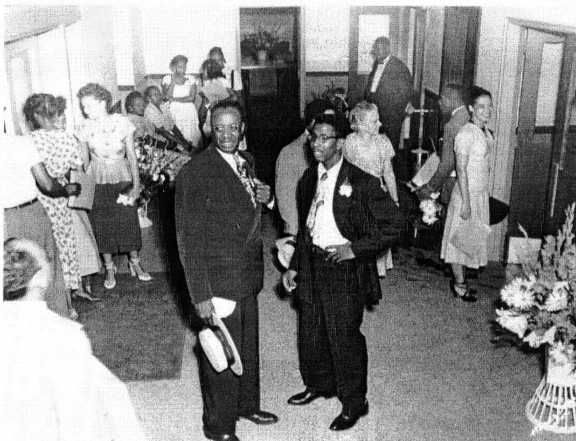
View of the lobby of the Universal Life Insurance Company building during its dedication celebration in 1949. At this time, the reception desk existing in the lobby had yet to be installed. Source: Memphis Public Library
