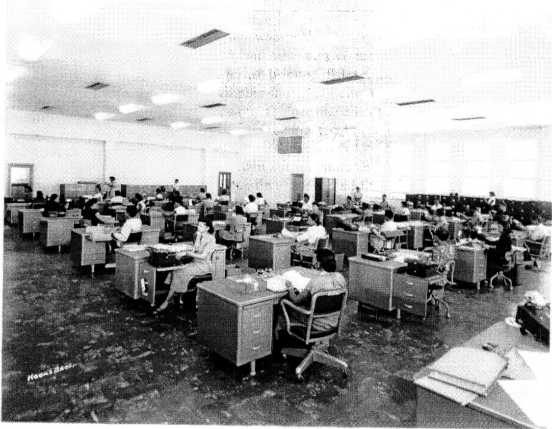
View across the large secretarial pool in the southeast quadrant of the second floor of the building, taken ca. 1955. Source: Memphis Public Library
