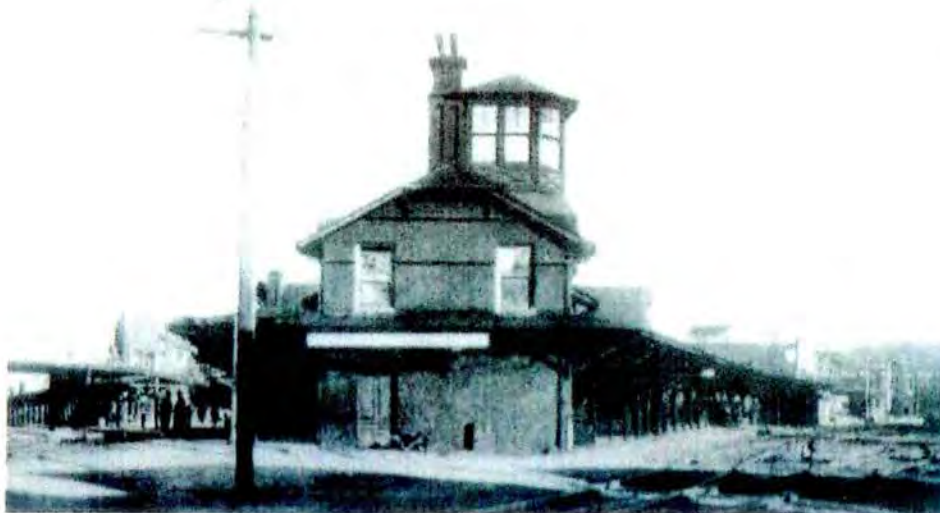
Fig. 317. South depot at Charl 1885, 1913
