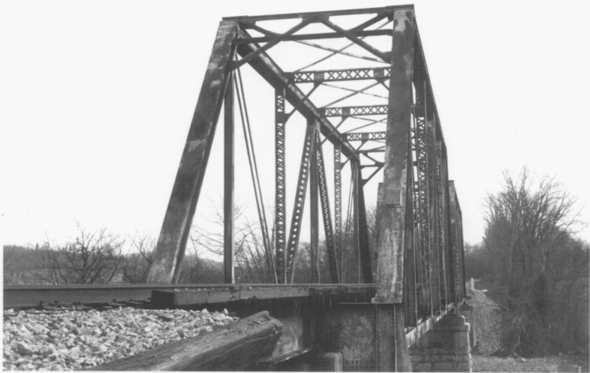
Southern Railroad Bridge, Blount Co., TN, Photo 1 of 2
