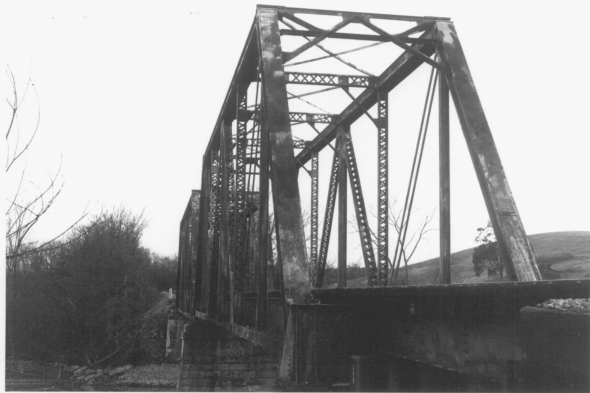
Southern Railroad Bridge, Blount Co., TN, Photo 2 of 2
