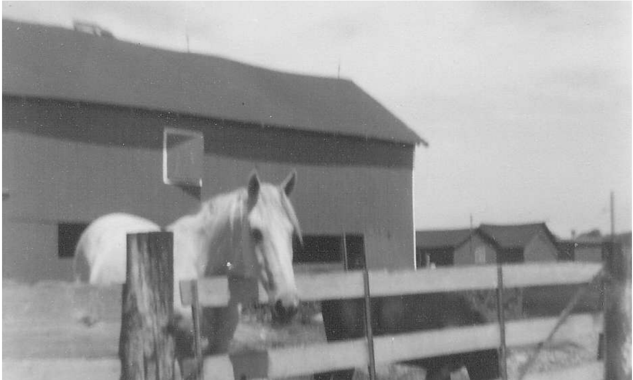
7. Southeast end of barn looking northeast, 1966. Horse stalls occupy the south side of the barn, the top of the silo is visible beyond the roof ridge, and labor houses stand beyond. (Courtesy Suzanne H. Culver)
