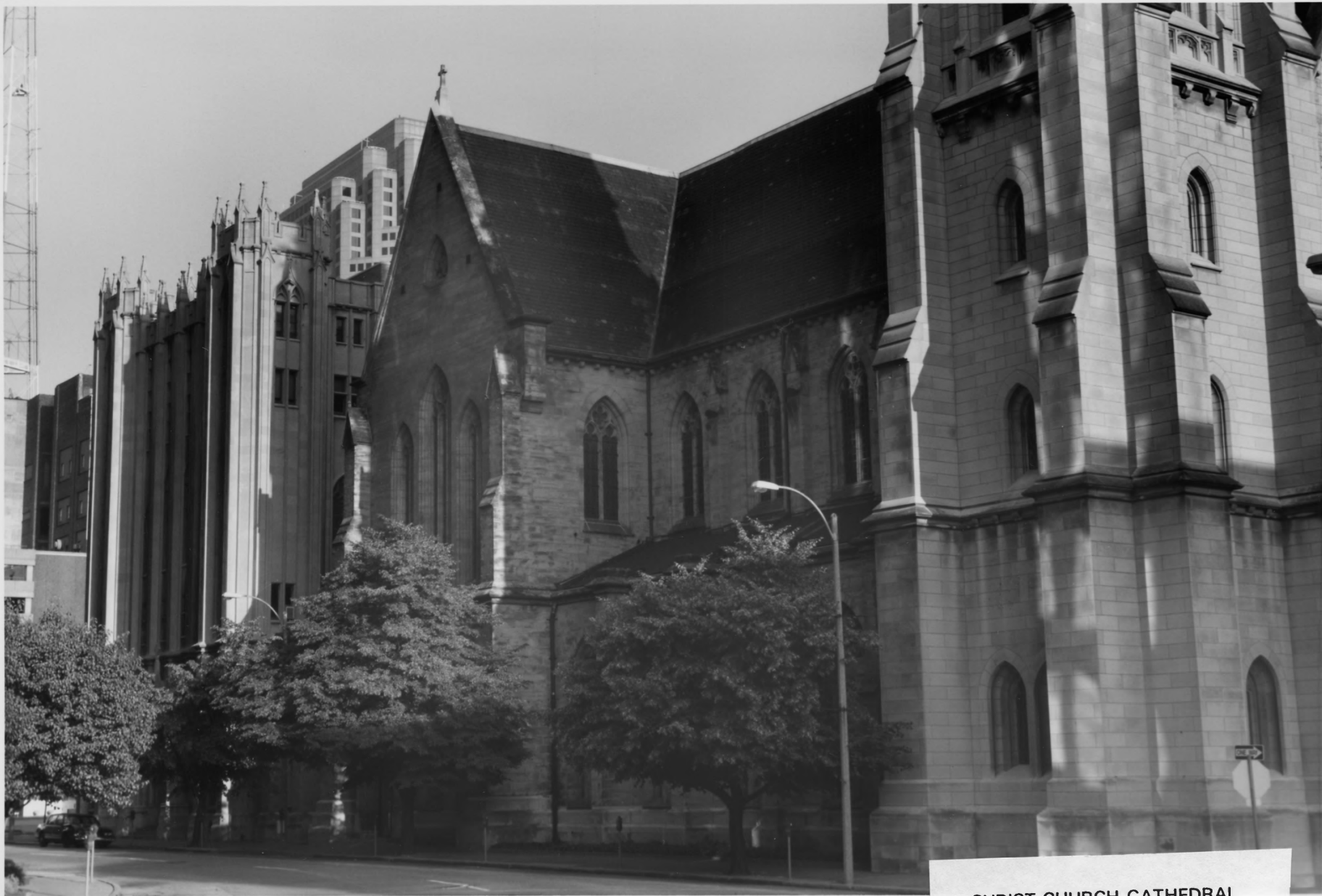
CHRIST CHURCH CATHEDRAL St. Louis, Missouri North transept & tower, Tuttle memorial in background Photo: Quinta Scott, 1988
