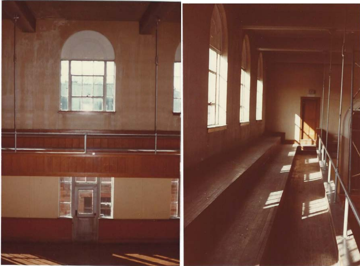
Figure 7: Memorial Building auditorium balcony prior to the 1983 renovations showing the original plaster ceiling, roof beams, and lunette windows.
