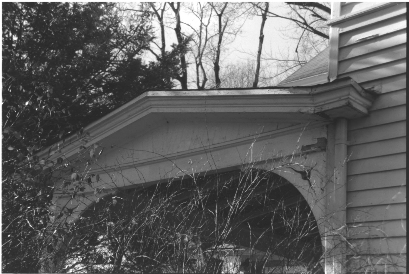
JOHN JACOB BOBERT HOUSE, HARRINGTON PARK, BERGEN COUNTY, NJ #14
