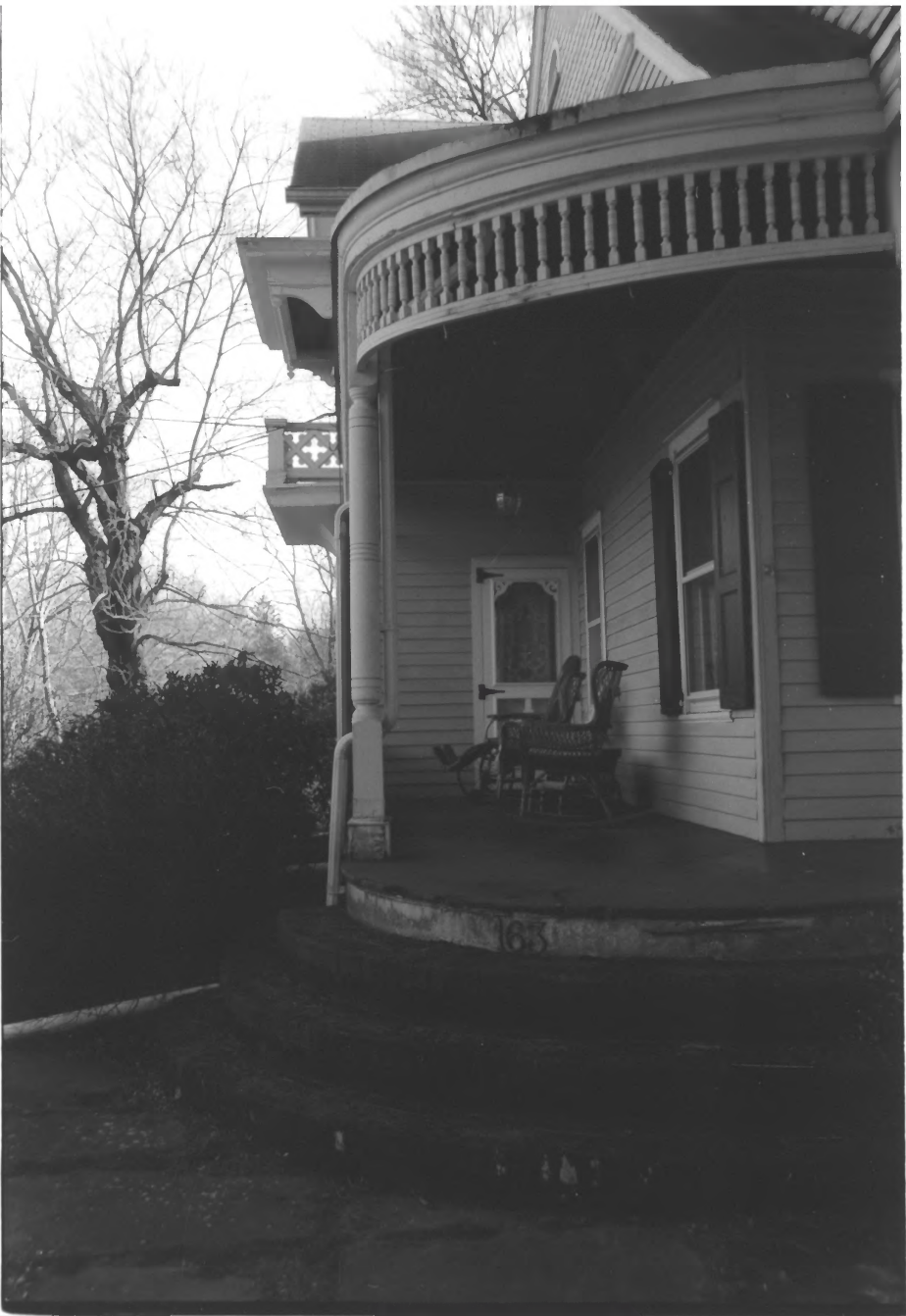
JOHN J. KOB BOESET HOUSE, HARRINGTON PARK, BERGEN COUNTY, NJ #4
