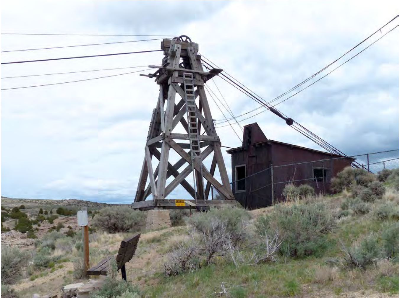
Photo #17: South cableway tower and cableway powerhouse (part of Feature M and Feature N, contributing). Camera facing east. See Photo #47 for opposite view.
