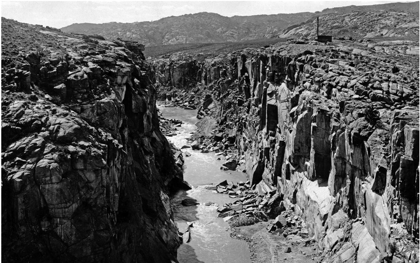
Historic Photo #2: Pathfinder Damsite. This view was taken August 17, 1905 from a point a short distance below the damsite. It shows the river at low water. At the foot of the canyon wall on the right of the picture is the outlet of the north tunnel. The spoil in the channel further up the stream shows the location of the north tunnel intake. The location of the shaft is shown by the waste material near the top of the canyon wall.
