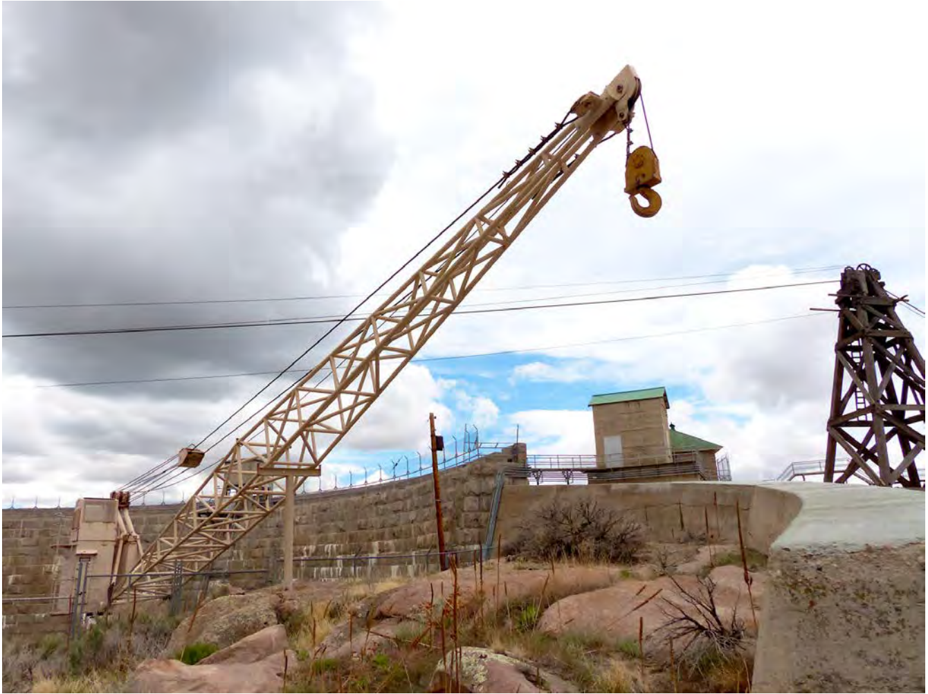
Photo #15: From left, LeTourneau electric deck crane (Feature L, non-contributing), Sluice Gatehouse, and north cableway tower. The spillway training wall extends from the right foreground over to connect with the dam's left (north) abutment in the center of the view. Camera facing southwest.
