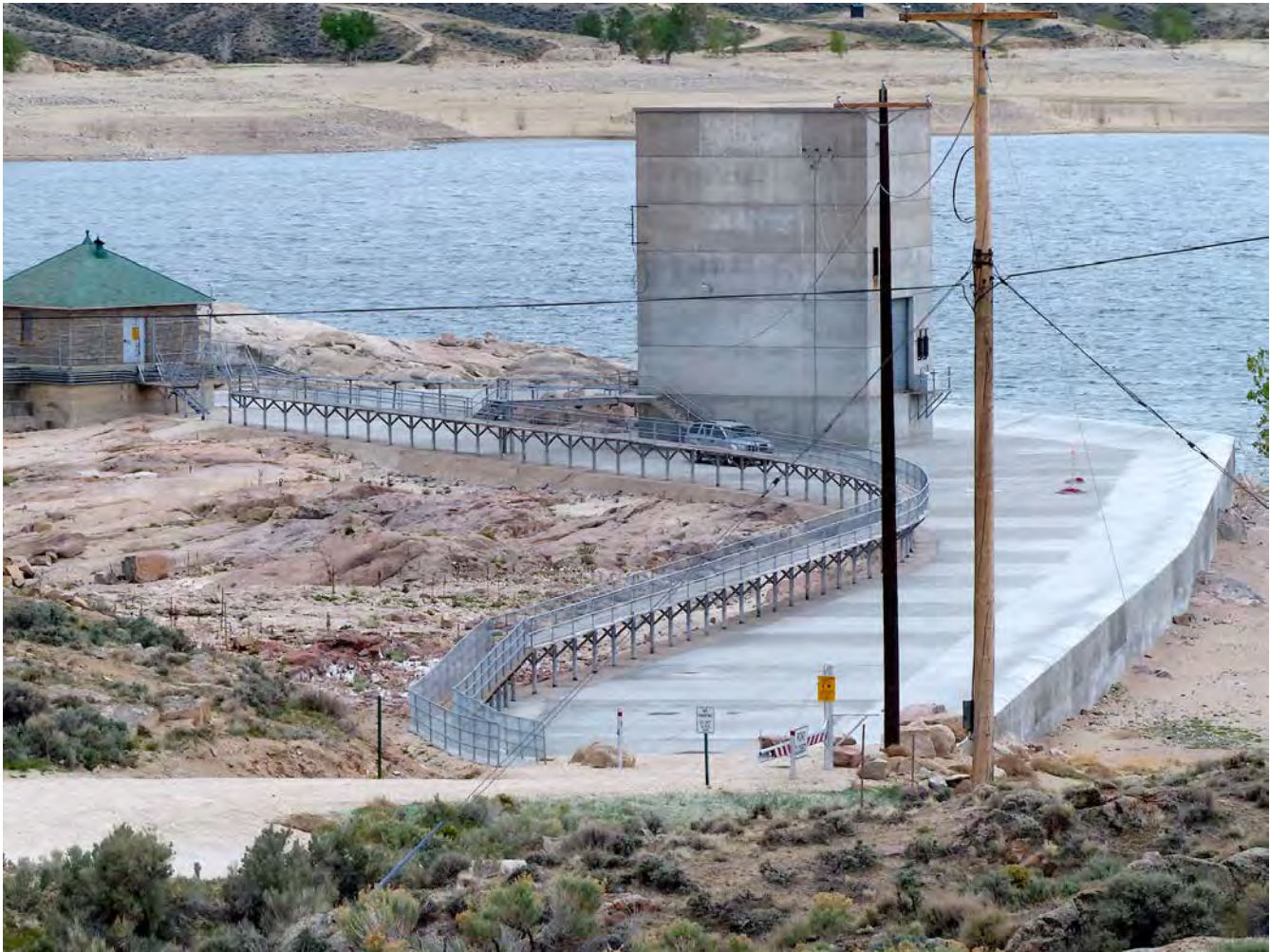
Photo #6: Emergency Gatehouse at left of view; the Fremont Canyon Power Plant Conduit Fixed Wheel Gatehouse at center of the view (Feature K, non-contributing); the facility access walkway (Feature I, non-contributing) across the upstream end of the Pathfinder spillway. The new spillway ogee weir and concrete apron (Feature J, non-contributing) are to the right of the walkway, and the natural (original) surface of the spillway is the left of the walkway. Pathfinder main quarry (Feature 7A, non-contributing) was situated in the area of the spillway seen here to the left of the walkway, and was incorporated in 1909 into the spillway channel. Camera facing south.
