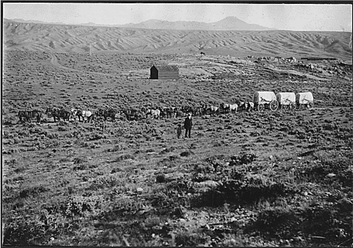
Historic Photo #1, July 16, 1907, Pathfinder Dam, 22-horse freighter hauling cement and other construction materials from rail head at Casper to dam site, 47 miles distant.
