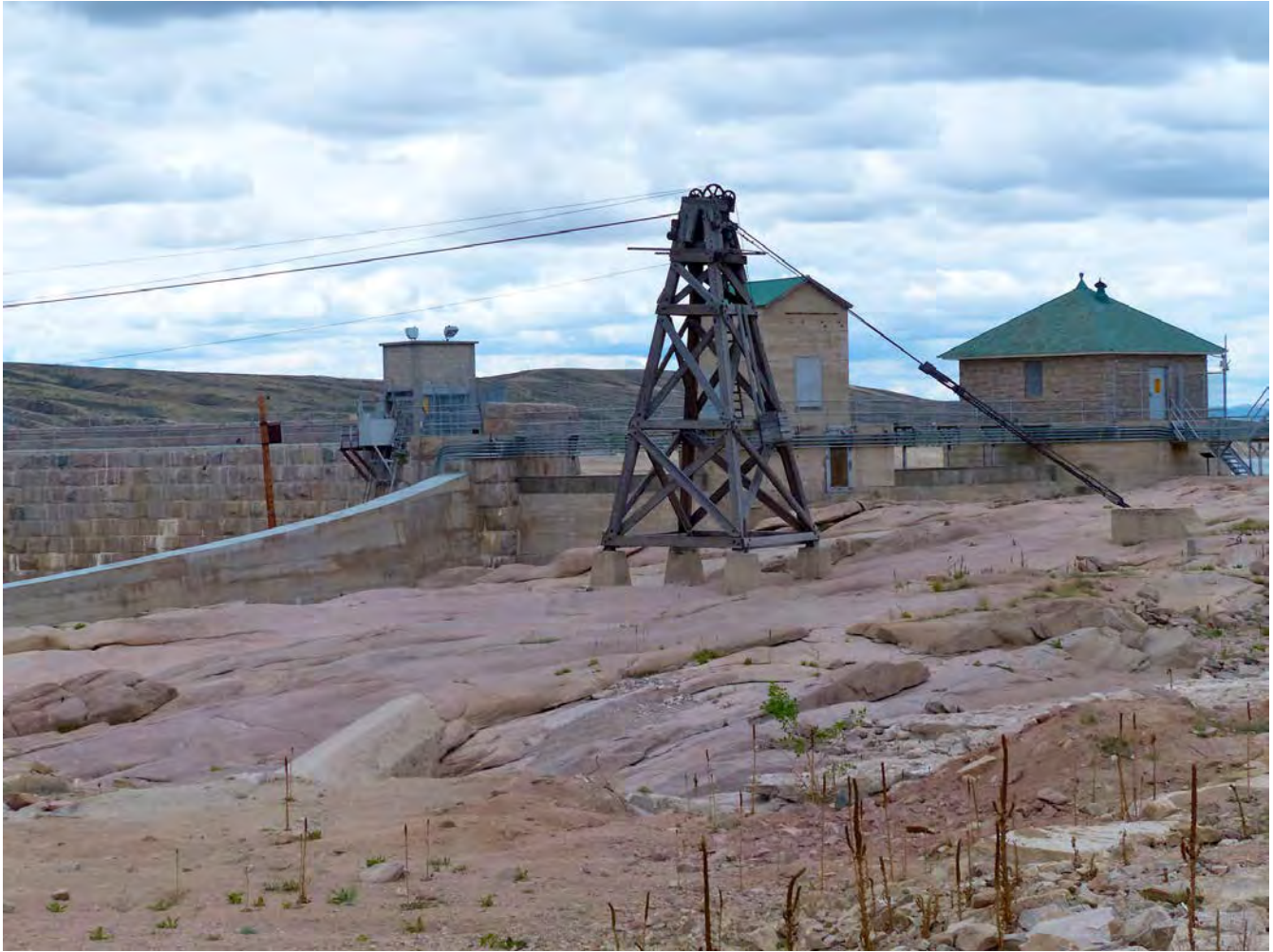
Photo #16: From left, dam crest, spillway training wall, elevator machine house, north cableway tower, Sluice Gatehouse, and Emergency Gatehouse. "Natural" spillway in foreground. The main quarry is out of view to the left. Camera facing south-southwest.
