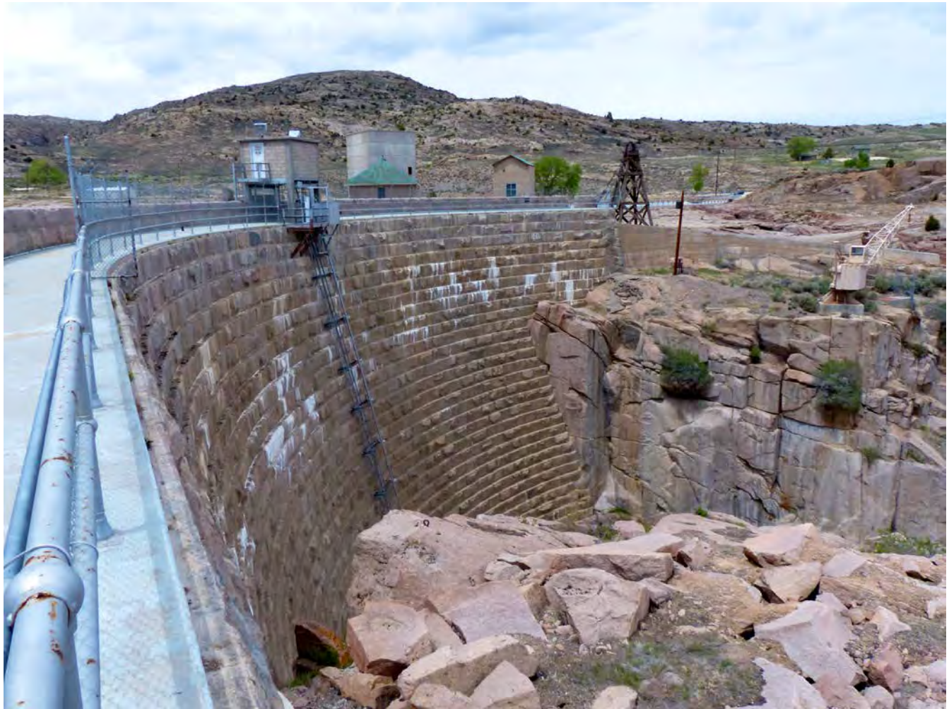
Photo #2: Pathfinder Dam from south abutment. Camera facing north.
