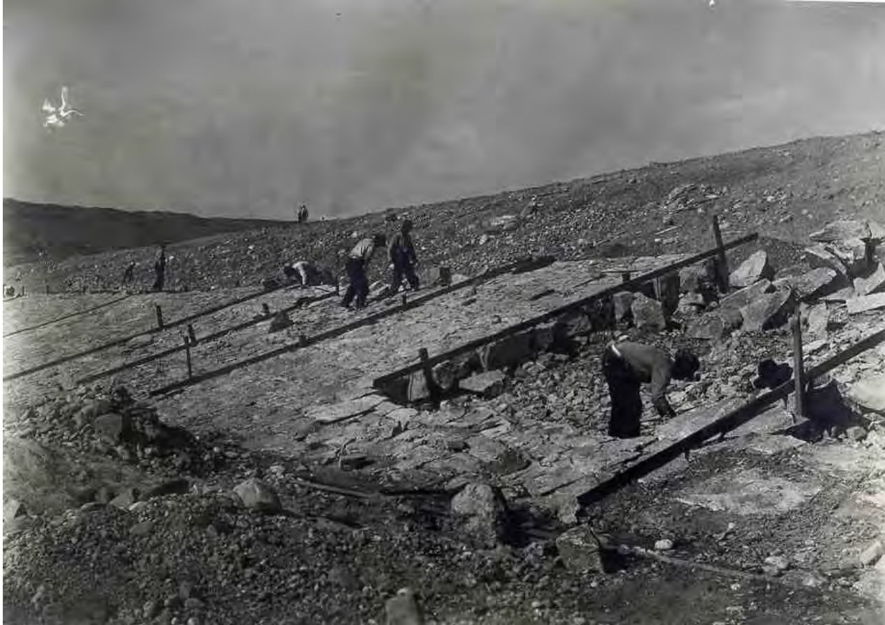
Historic Photo #20: August 8, 1910, Pathfinder Dike, showing stone paving on upstream face.
