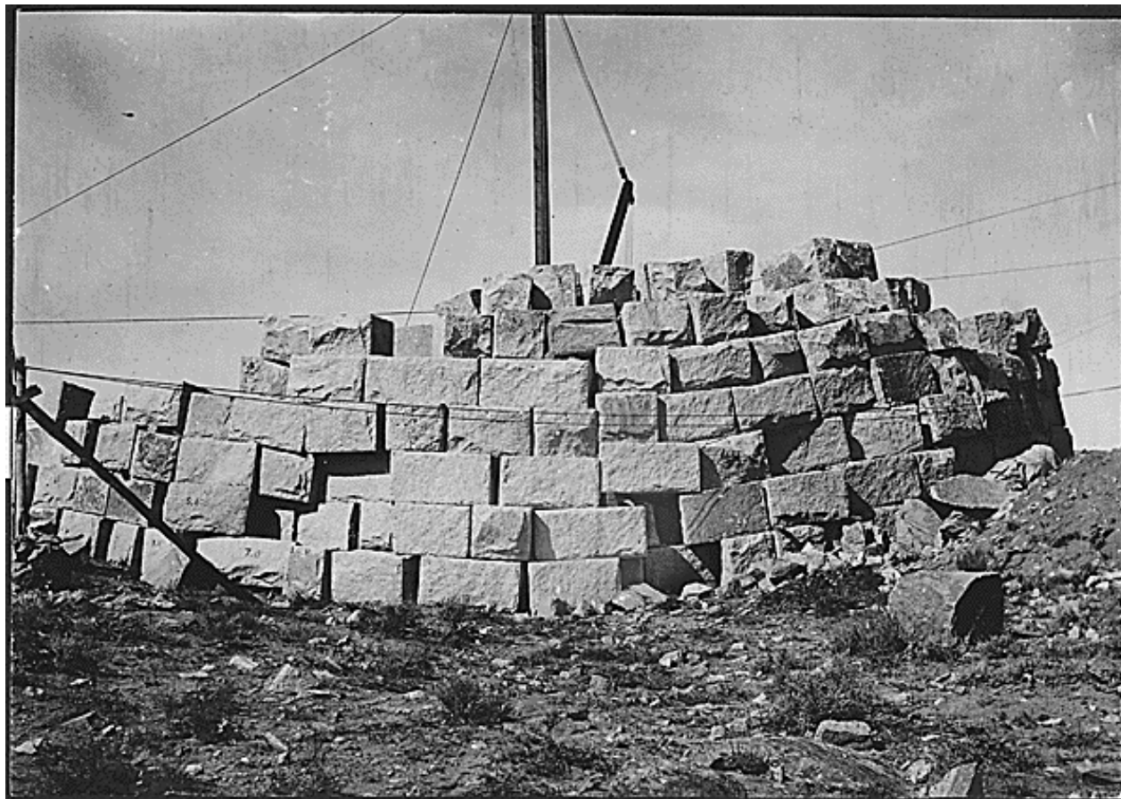
Historic Photo #13 1908, Pathfinder Dam, three-foot face stones in storage
