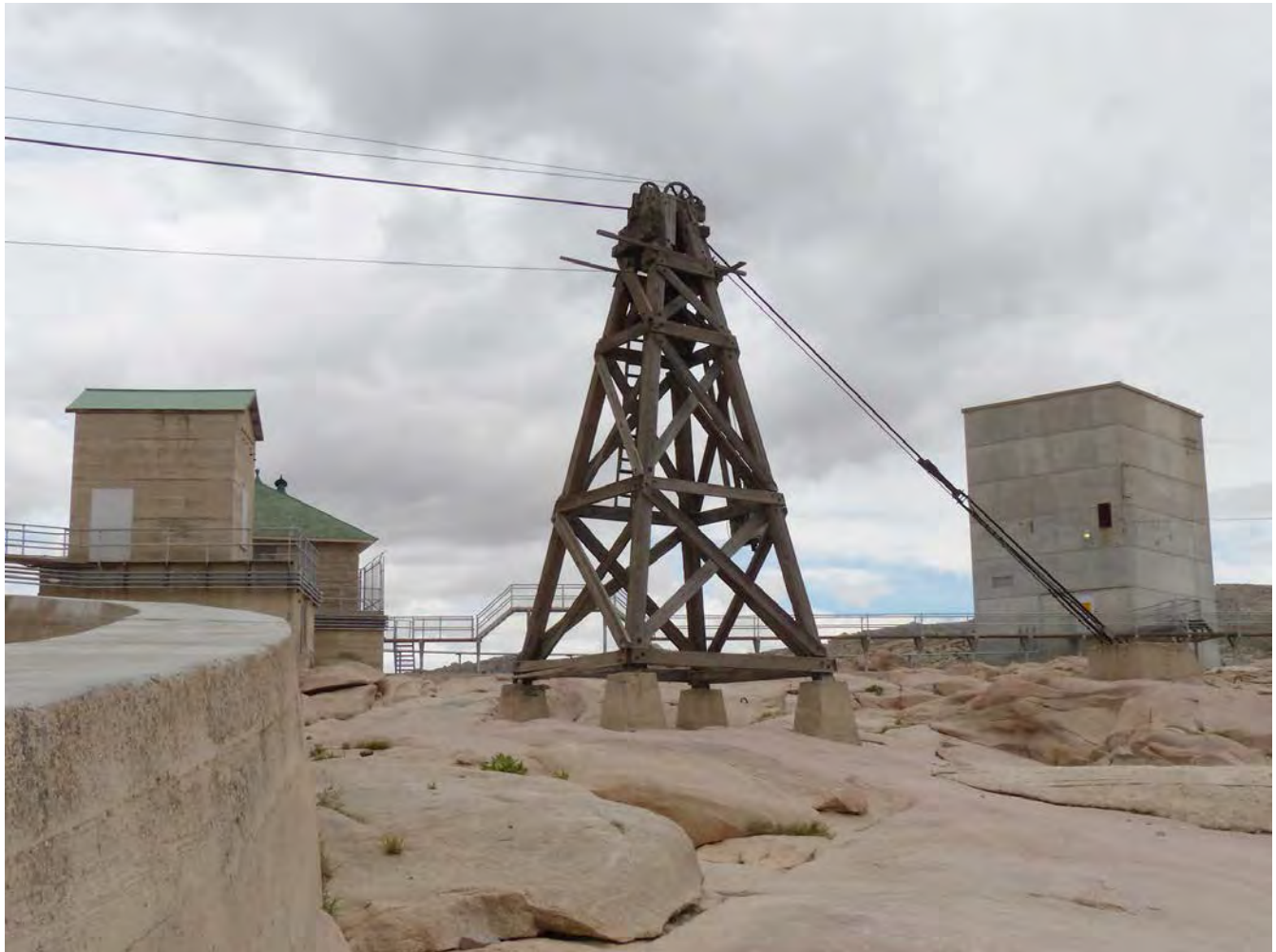
Photo #9: In the foreground, a section of the spillway and spillway training wall (Feature H, contributing). Behind, from left are: the Sluice Gatehouse (Feature D, non-contributing) with the Emergency Gatehouse behind it; the north cableway tower and associated concrete anchor pad and connecting cable (Feature M, contributing); and the Fixed Wheel Gatehouse. Camera facing northwest.
