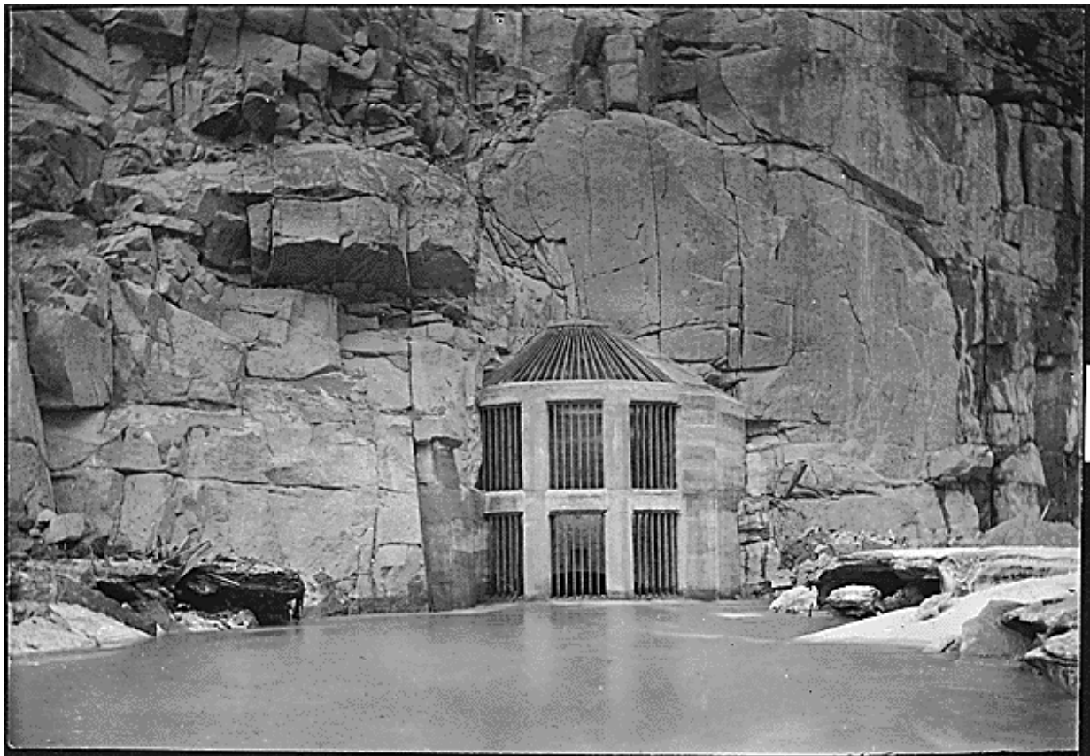
Historic Photo #16: February 5, 1909, grillage at entrance to (north) Pathfinder Tunnel
