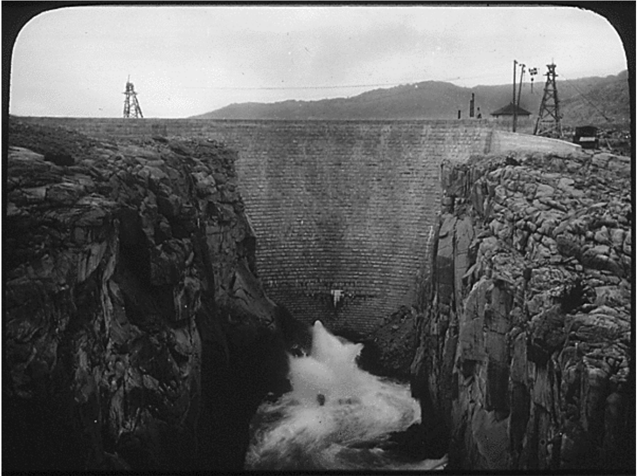
Historic Photo #19: Pathfinder Dam, 1909, showing river outflow from the dam conduit outlet. Note that one of the two original cableway systems remains in use. The Emergency Gatehouse roof is visible at right.
