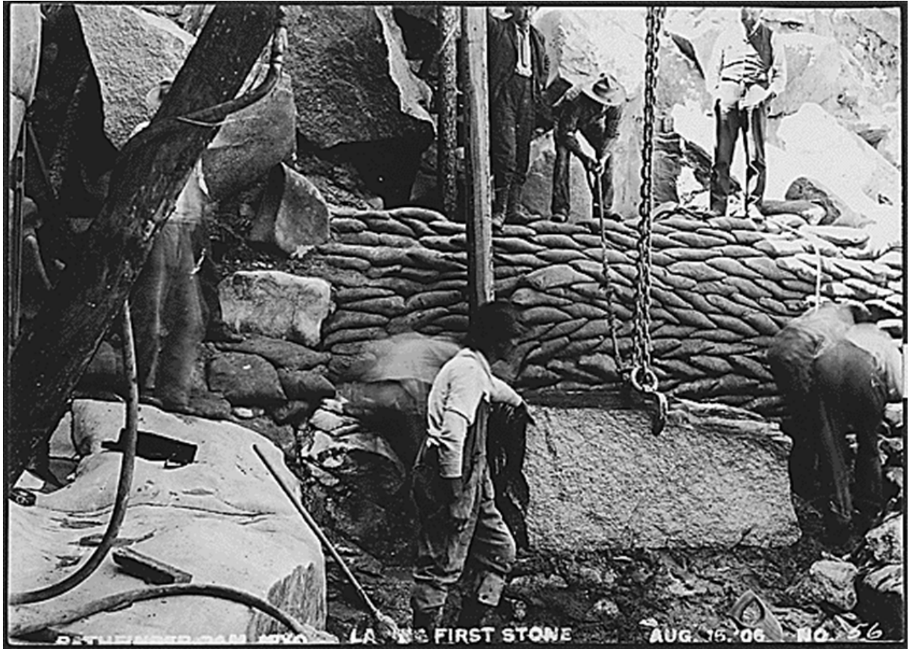
Historic Photo #6: Pathfinder Dam, laying the first stone, August 15, 1906
