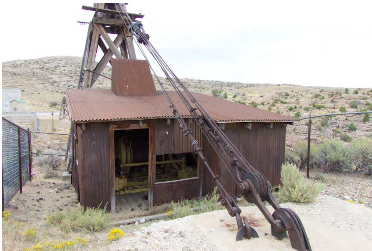
Photo #47: Cableway powerhouse (Feature N, contributing) south elevation. In foreground, guy and tension wire anchors for south cableway tower. Camera facing south.
