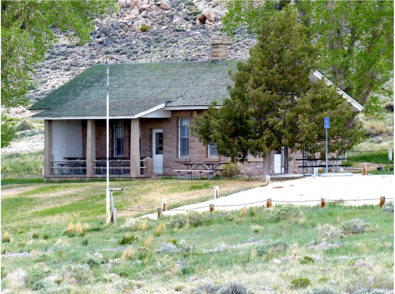
Photo #24: Dam tender's house, main (south) elevation. Camera facing northwest.
