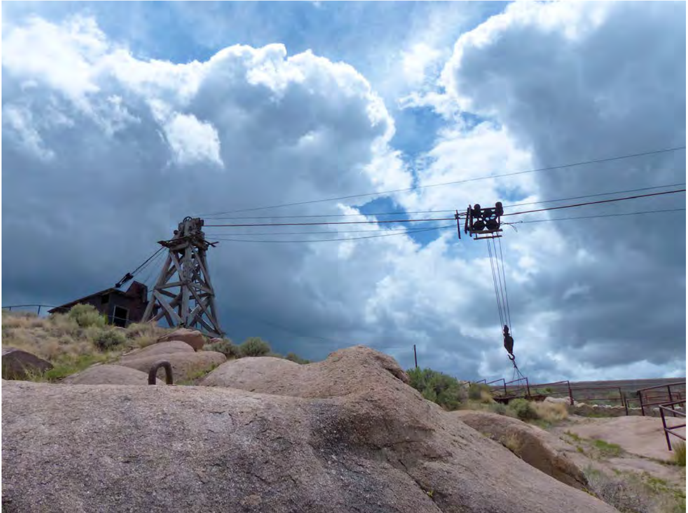
Photo #19: South cableway tower , carriage assembly, and cableway powerhouse. Note U-bolt set into granite during dam construction, likely used as a crane or gaff guy wire anchor. Camera facing southwest.
