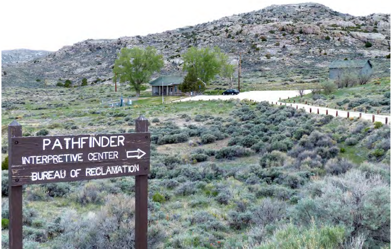
Photo #23: Pathfinder dam tender complex (Element 3, two contributing buildings). Camera facing northwest.
