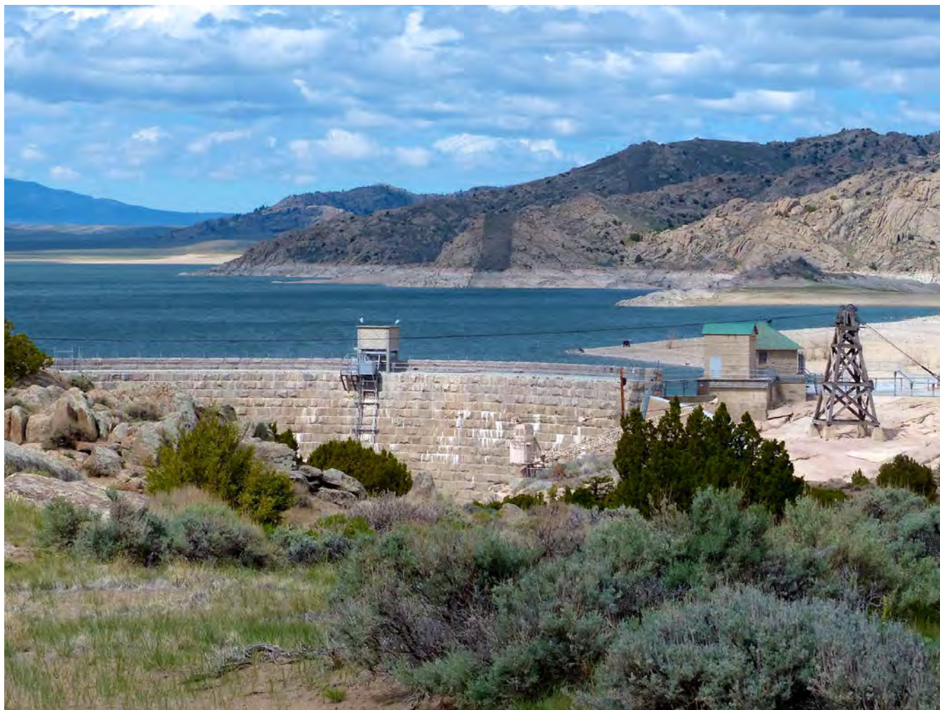
Photo #43: Pathfinder facility and Pathfinder Reservoir overview. Camera facing west.
