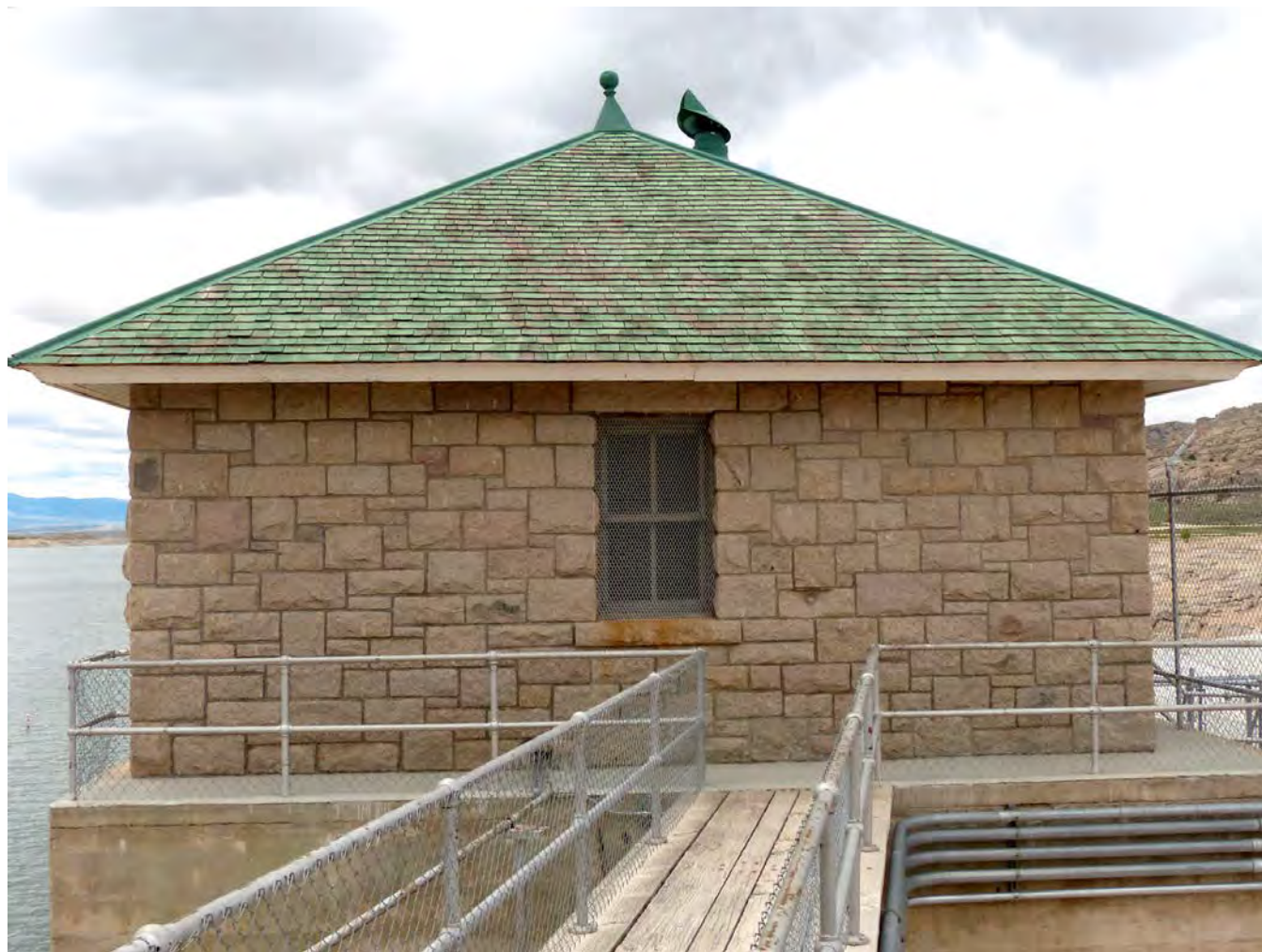
Photo #8: Pathfinder Dam Emergency Gatehouse (Feature C, non-contributing). Camera looking west.
