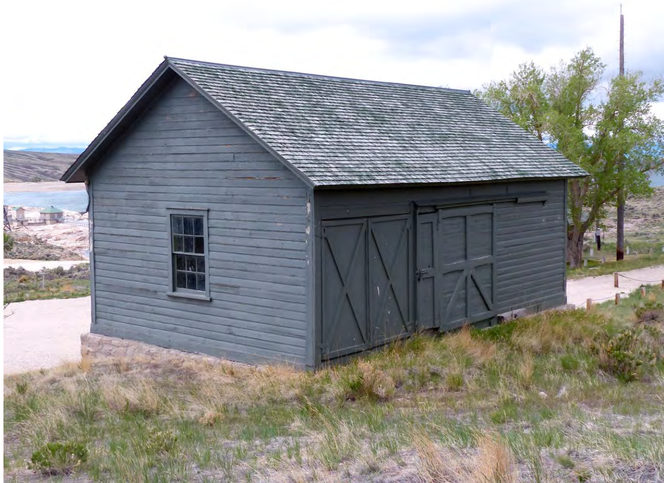
Photo #28: Pathfinder dam tender complex barn, north and east elevations. Note the spillway and Emergency and Sluice Gatehouses visible to the left of barn. Camera facing southwest.
