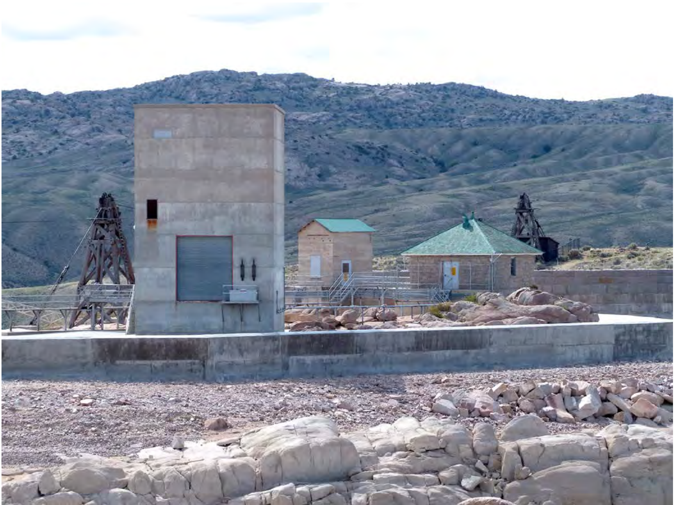
Photo #13: View of Pathfinder facility at the dam crest elevation. From the left: the north cableway tower; Fremont Canyon Power Plant Fixed Wheel Gatehouse; Sluice Gatehouse; Emergency Gatehouse; and south tramway tower. Upper face of the new spillway ogee weir in foreground. Camera facing southeast.
