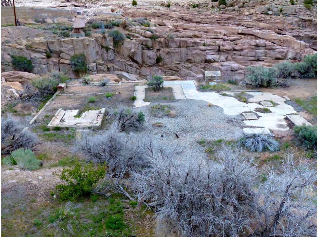
Photo #18: Foundations (Feature O, non-contributing) on south side of canyon above the south access ladderway. Camera facing north. See historic photo #22 to view the buildings that stood here in 1940.
