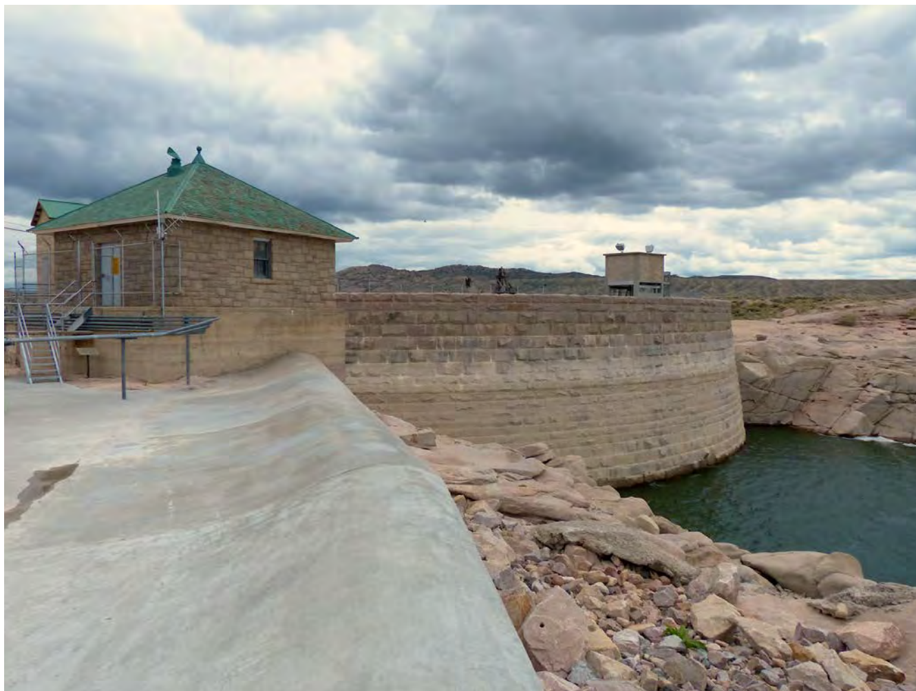
Photo #5: Pathfinder Dam's upstream face, and Emergency Gatehouse (Feature C, contributing) on the left. Note new concrete spillway ogee weir and apron (Feature J, non-contributing). Camera facing southeast.
