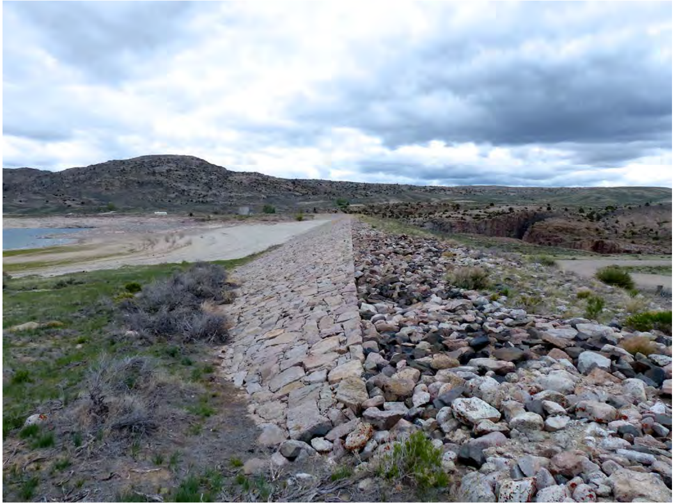
Photo #22: Pathfinder Dike. Camera facing north from south end of dike.
