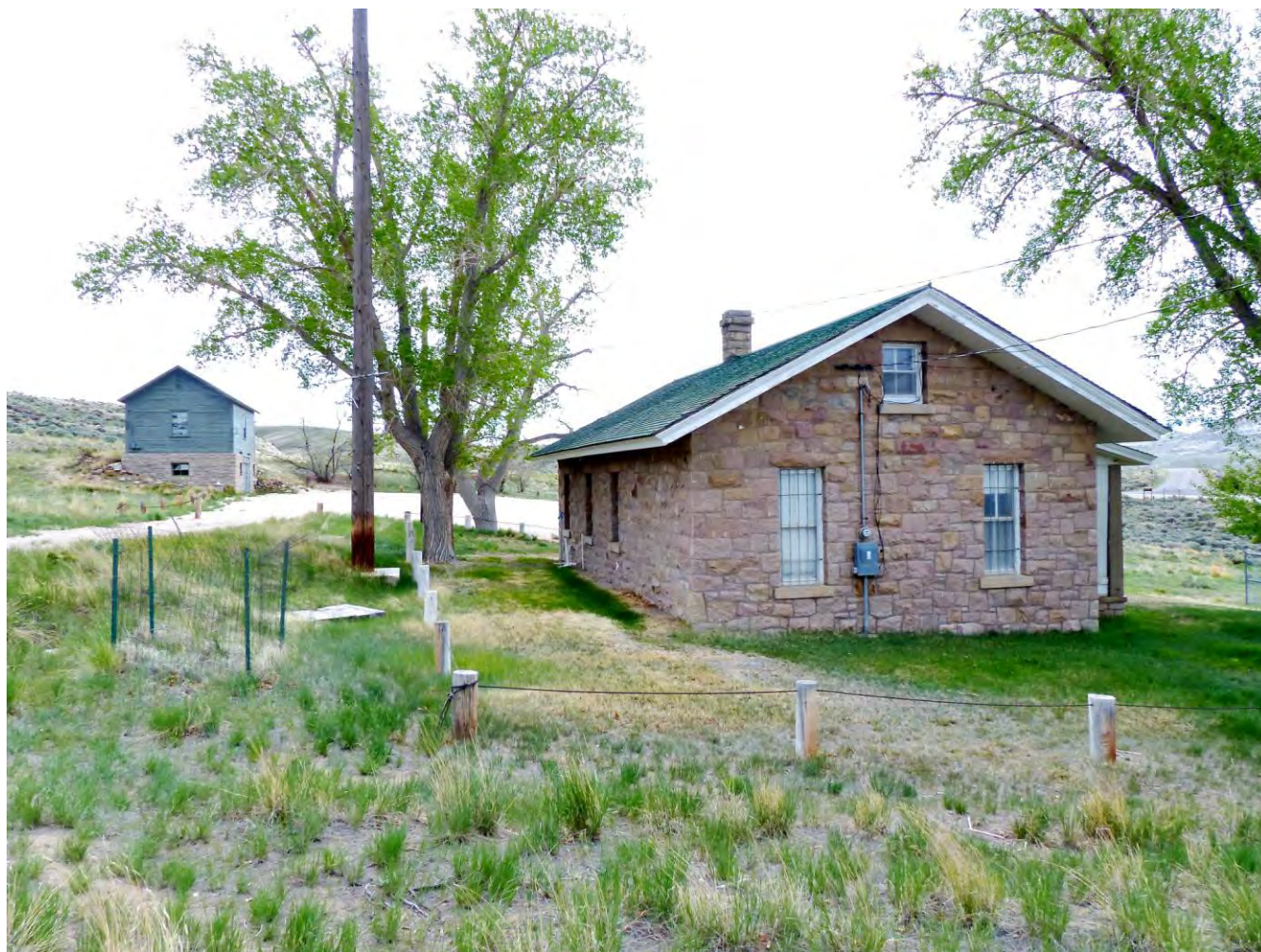
Photo #25: Pathfinder dam tender complex, house and barn west elevations. Camera facing east.
