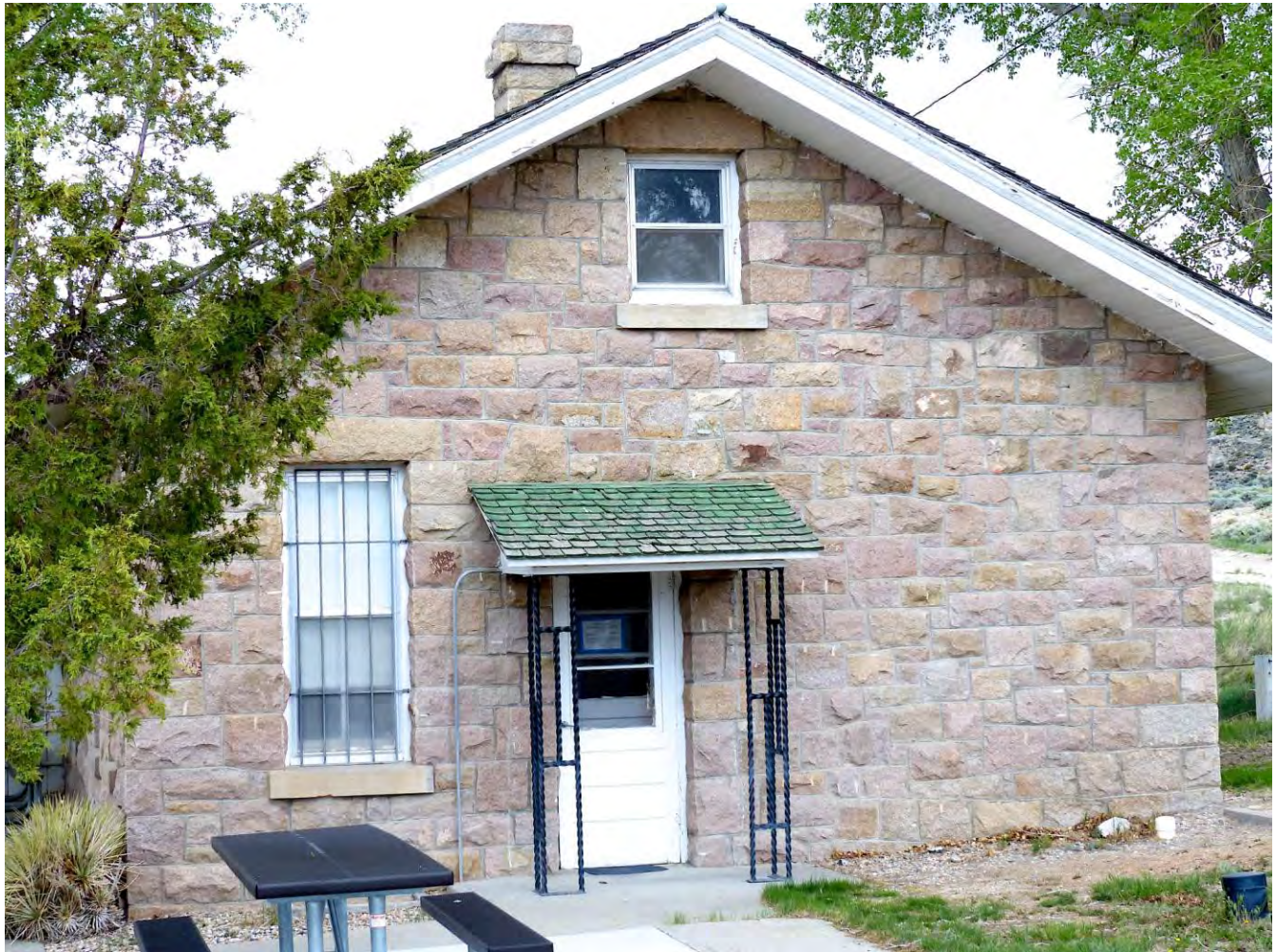
Photo #26: Dam tender house east elevation. Camera facing west.
