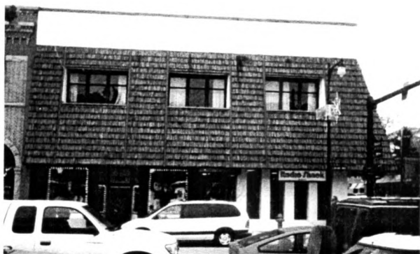
Bank building prior to rehabilitation in 2000
