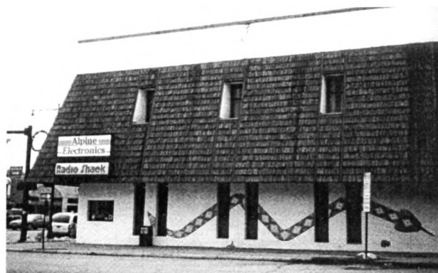
Bank building prior to rehabilitation in 2000
