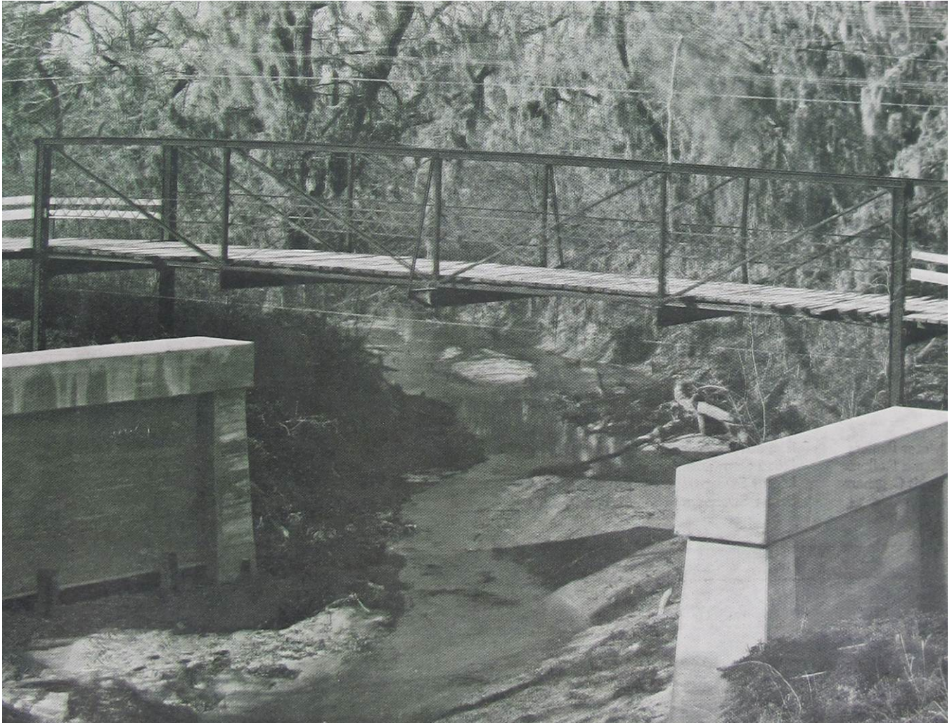
Figure 1. Bedstead Truss Bridge in Fayette County, Fayette County, Texas. (Source: Texas Highway Bulletin , December 1922).
